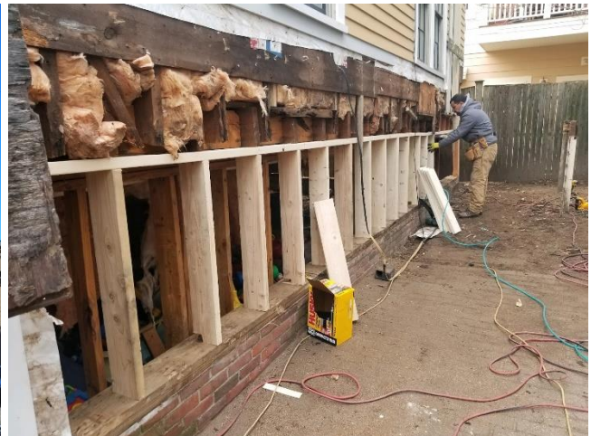
Non-Profit Row, 93-99 Bp. Allen Drive, as restored by the Cambridge Redevelopment Authority (left); replacement of rotted framing for affordable housing at 71 Bolton Street, by Just A Start, Inc.
