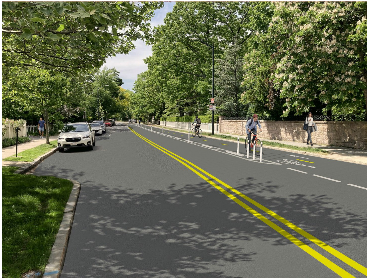
Example images of pre-cast concrete curbs with strategically placed flex-posts City of Cambridge | Brattle Street Separated Bike Lanes & Intersection Safety Improvements
