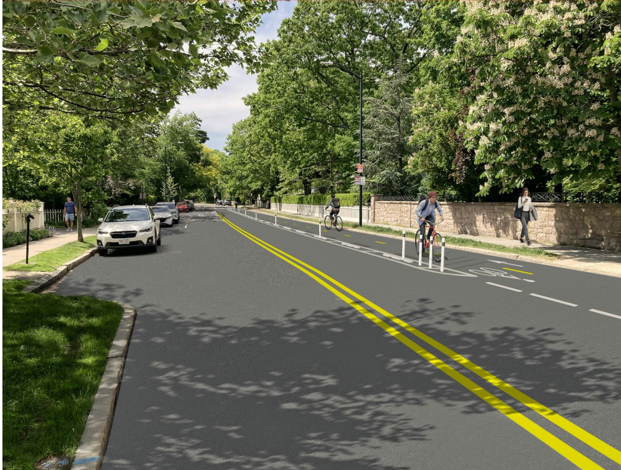
Example images of pre-cast concrete curbs with strategically placed flex-posts
