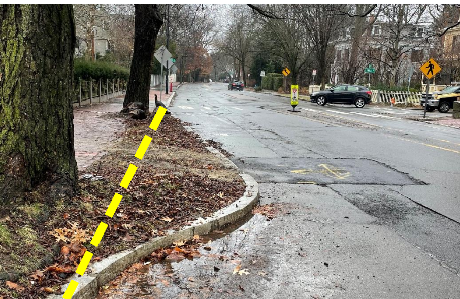
Photo of an existing curb bump out
