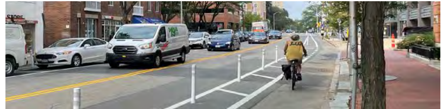
Separated bike lanes on Massachusetts Avenue
