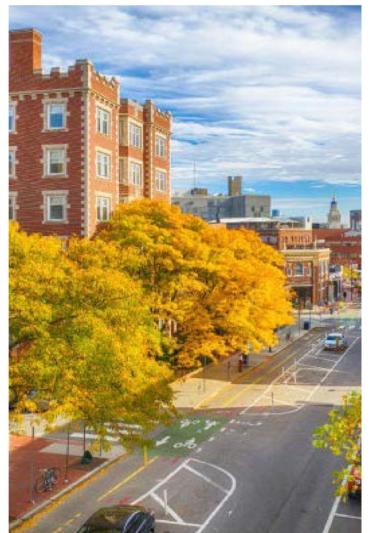
A separated bike lane on Brattle Street
