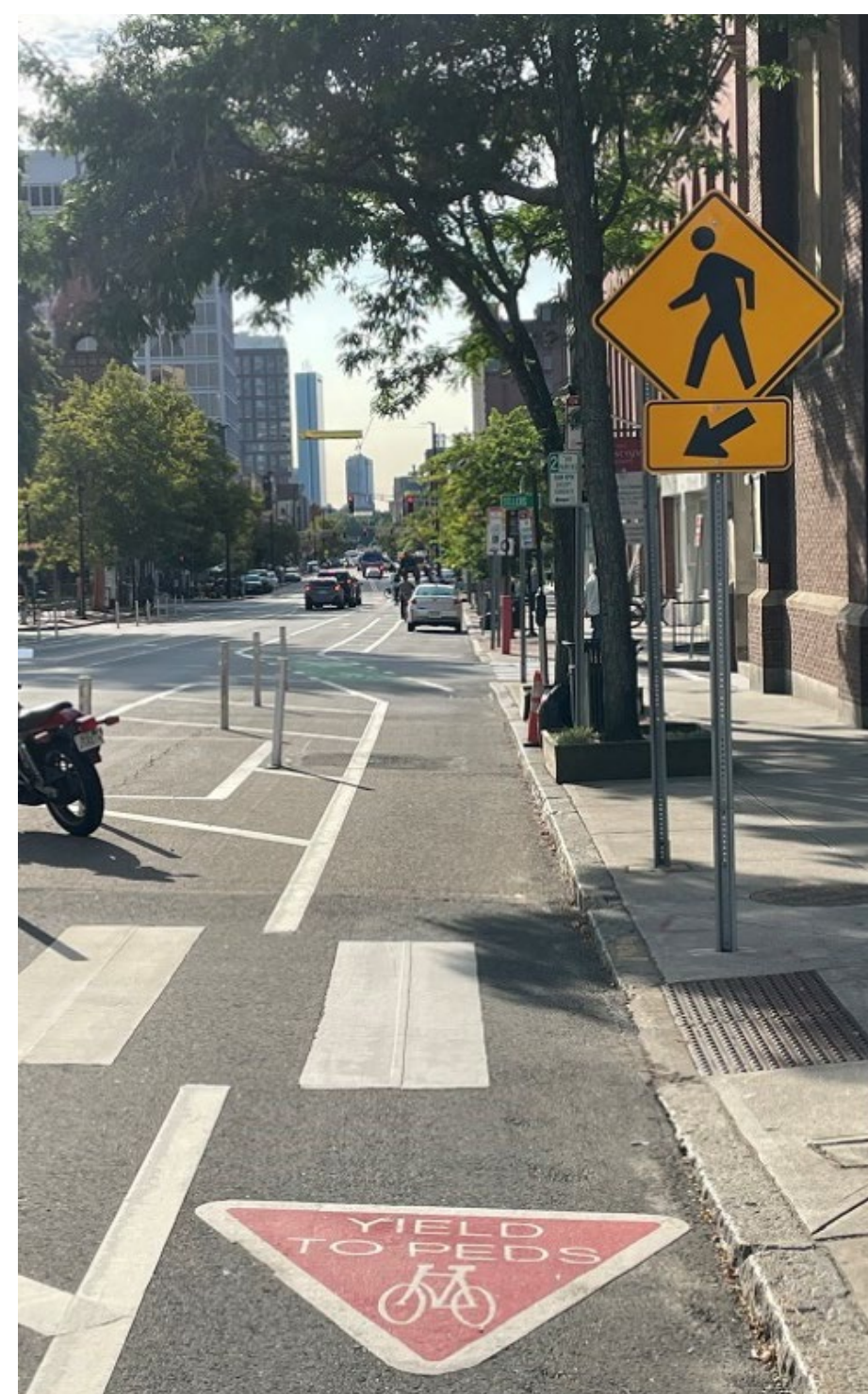
Example: Separated bike lane at crosswalk at Mass Ave at Clinton St
