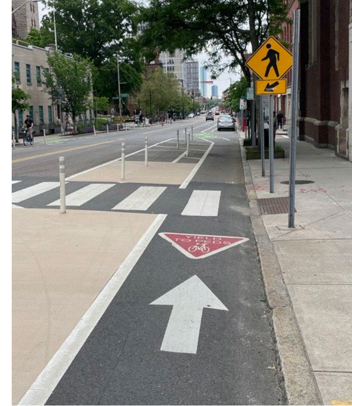
Example: Separated bike lane at crosswalk at Mass Ave at Clinton St
