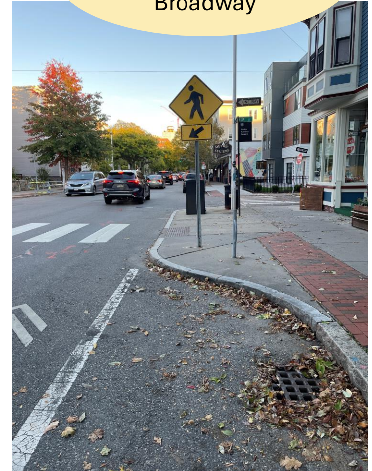
Existing Curb Extension at Elm St
