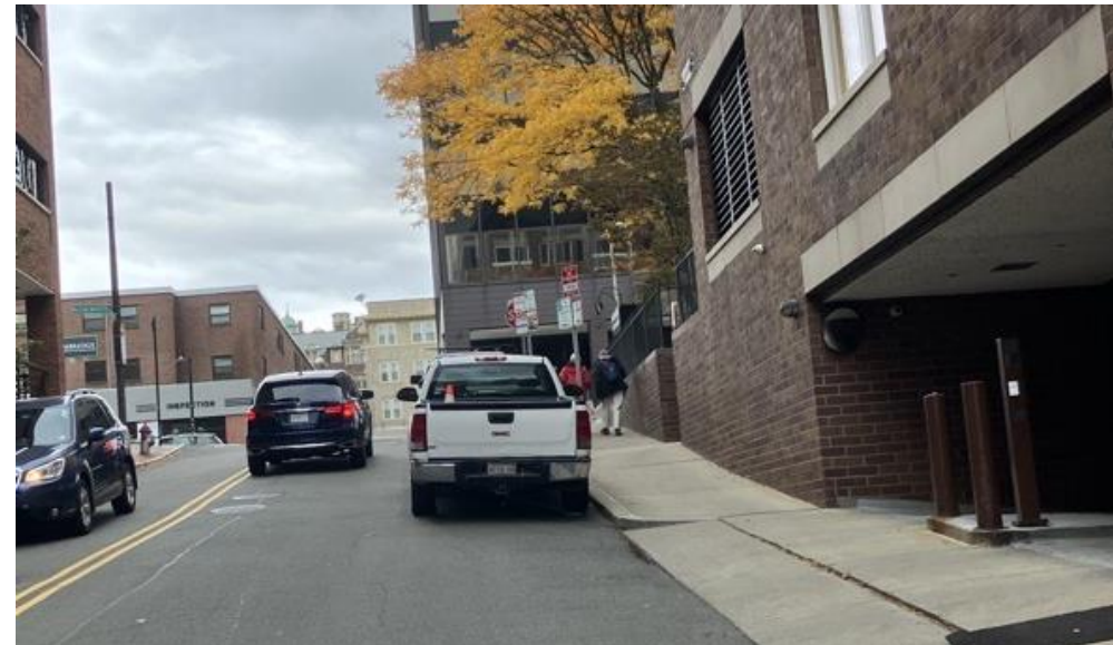
Bay Street, New Parking Created
