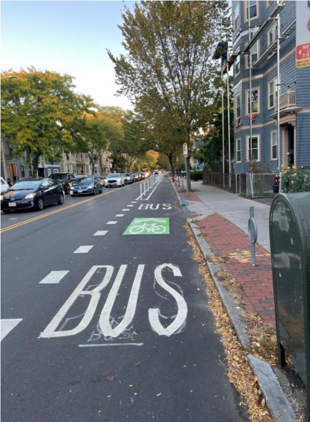
Completed quick-build style bus stop in Section A
