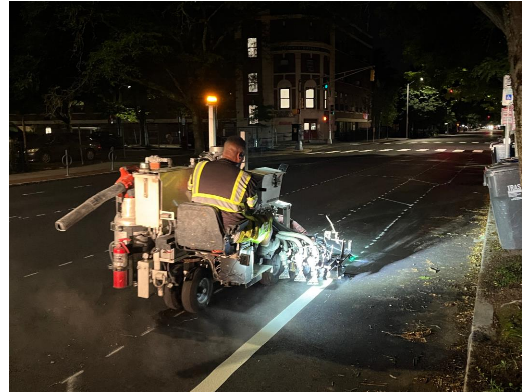
Image: Installation of thermoplastic lane lines on Broadway
