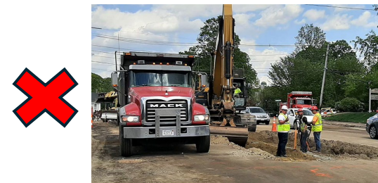
Full Depth Reconstruction
