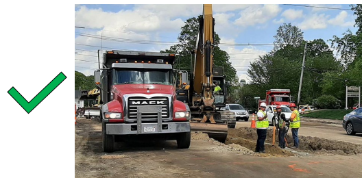
Full Depth Reconstruction
