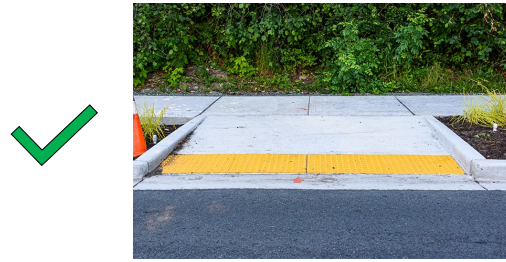
Retrofit Curb Ramps
