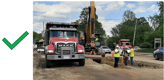
Full Depth Reconstruction
