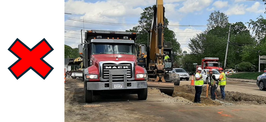
Full Depth Reconstruction
