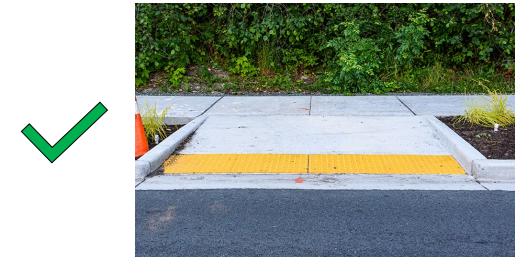
Retrofit Curb Ramps
