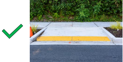
Retrofit Curb Ramps
