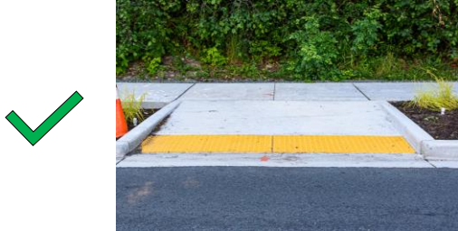
Retrofit Curb Ramps
