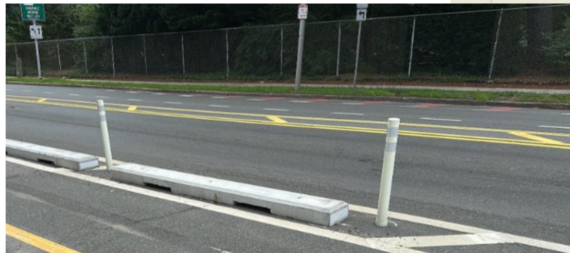
Precast curbing in use on Mt. Auburn St
