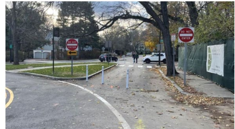
Photo showing the reconfiguration of Craigie St, installed as part of Phase 1 of the project last Fall.
