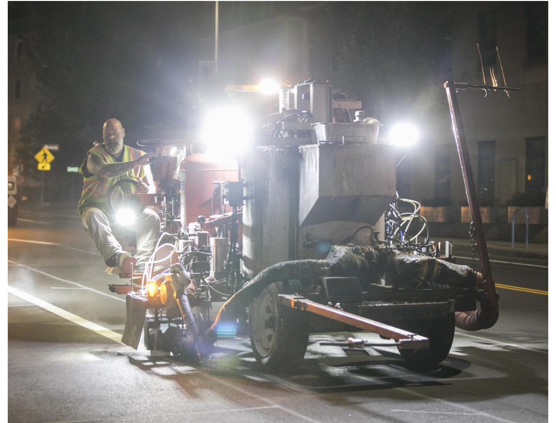
A worker installs new lines on Mass Ave
