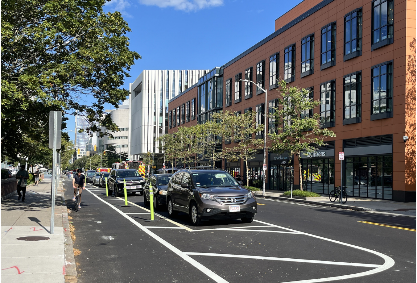
Main Street Safety Improvement Project, Post- Installation, November 2025.
