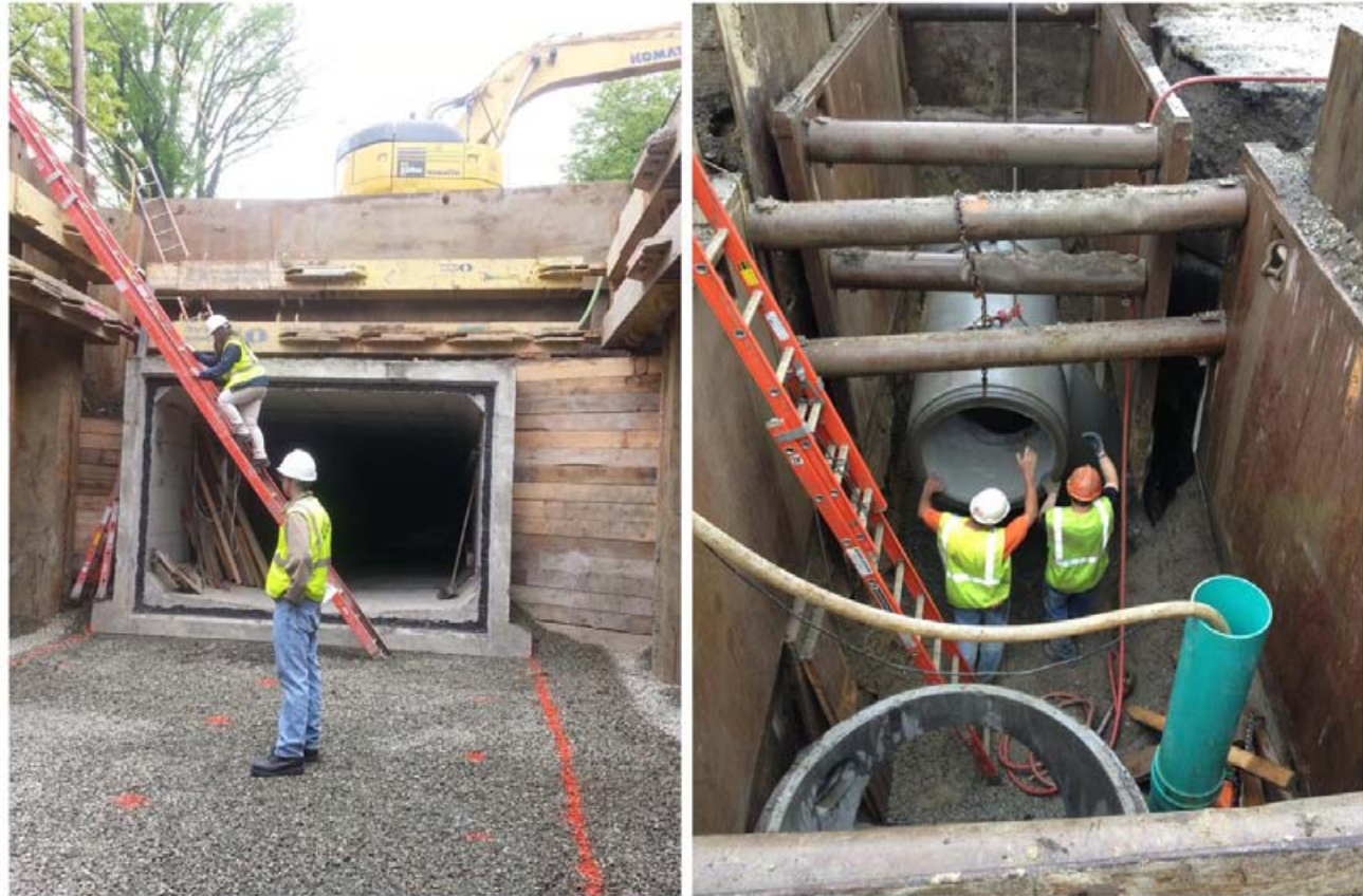
(L): Construction of a 160,000 gallon storm water holding tank on Hovey Street to reduce flooding in the Agassiz neighborhood. (R): Installation of 36" drain pipe, Western Avenue.
