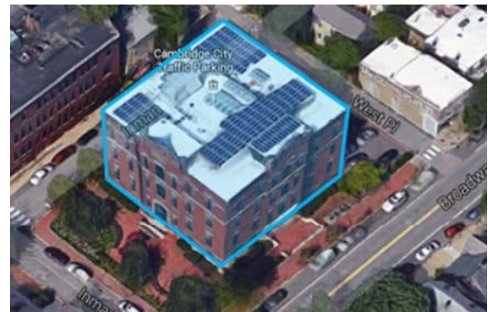
Energy reduction projects include comprehensive evaluations of building envelope to support efficiency projects.
