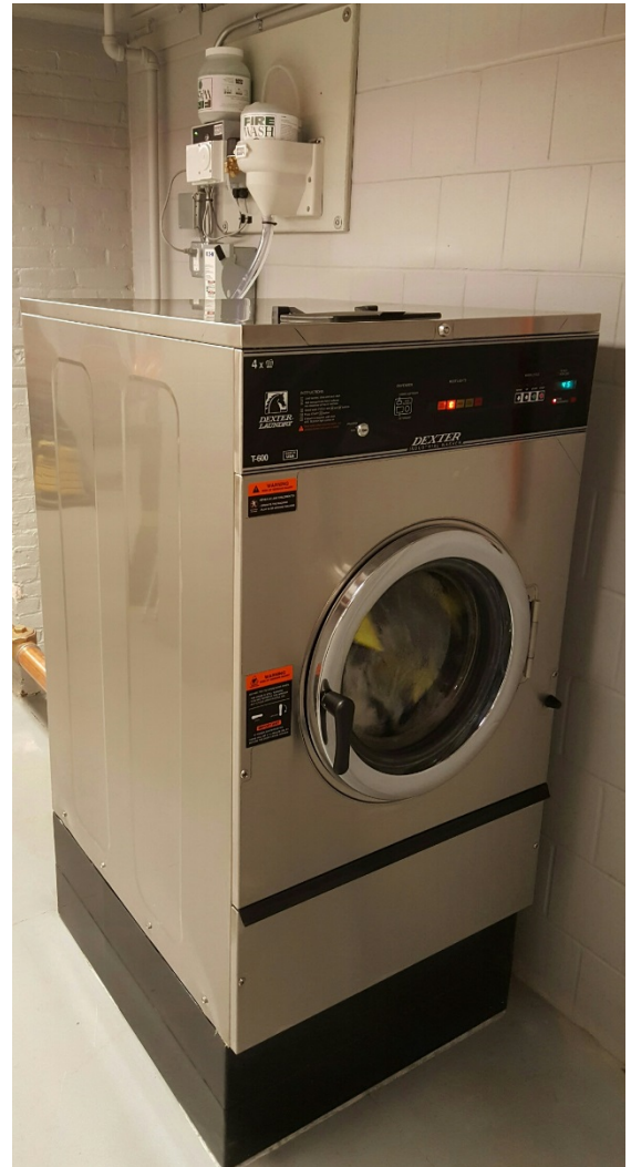
Firefighting gear washers have been installed in three fire stations and will soon be installed in a fourth. Products of combustion contain carcinogens that can permeate protective clothing, so CFD personnel are encouraged to wash their gear after each exposure.
