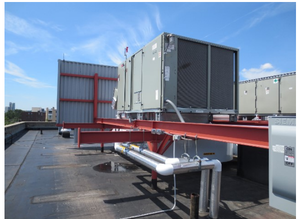
Public Works upgraded HVAC equipment on the Citywide Senior Center roof this year.
