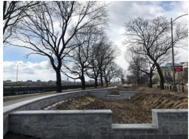
The Longfellow Bridge Project's subsurface gravel wetland
