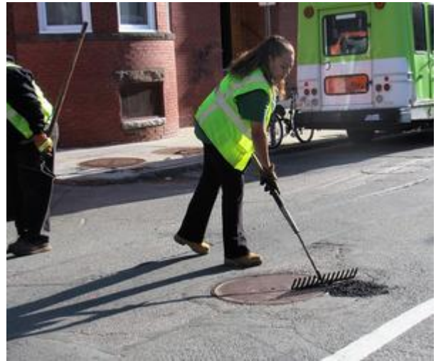
Repairing a pothole
