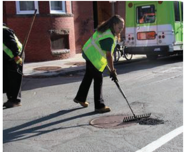
Repairing a pothole
