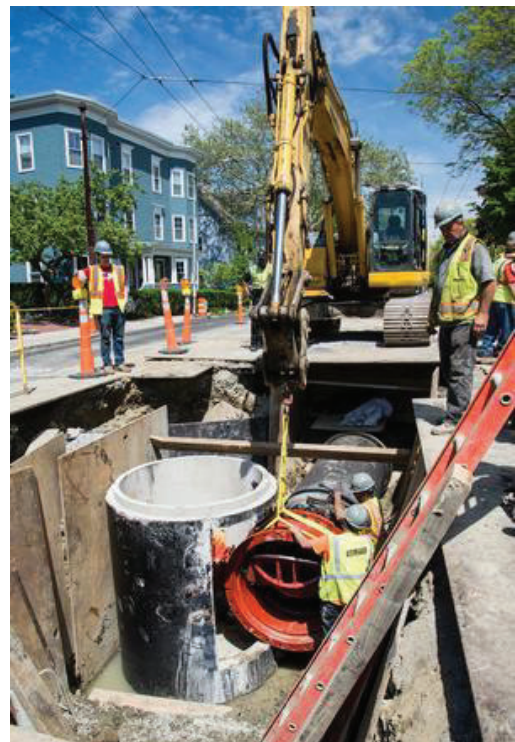
Sewer replacement work
