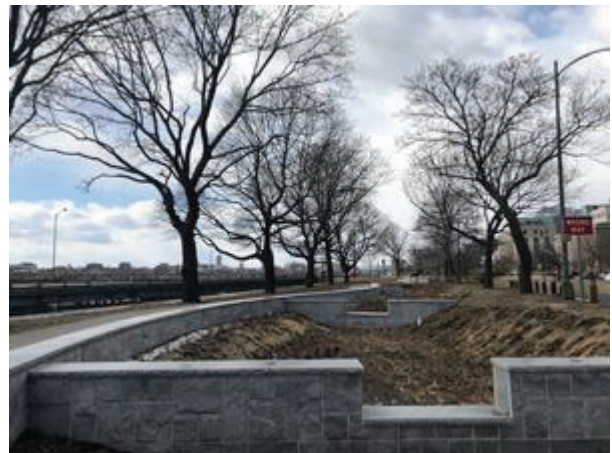
The Longfellow Bridge Project's subsurface gravel wetland
