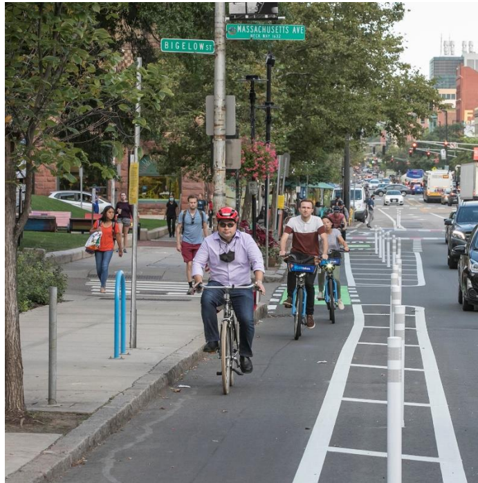
A newly-installed quick-build bike lane in Central Square
