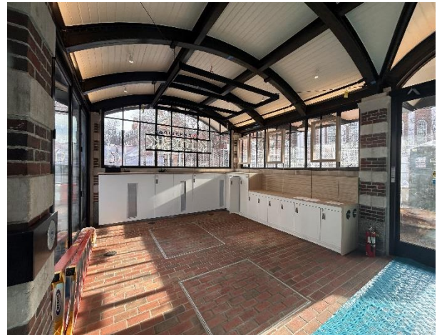
Interior of renovated Harvard Kiosk
