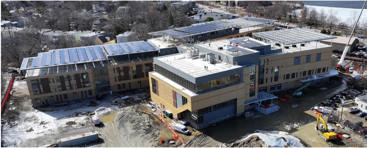
Construction of the Tobin Montessori and Darby Vassall Upper School Building
