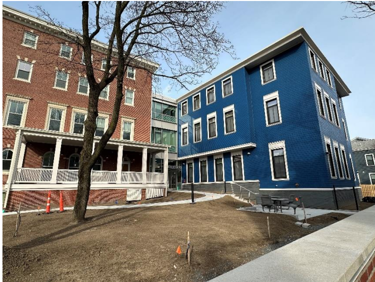
62 affordable supportive housing units at 116 Norfolk St. for residents who have been homeless
