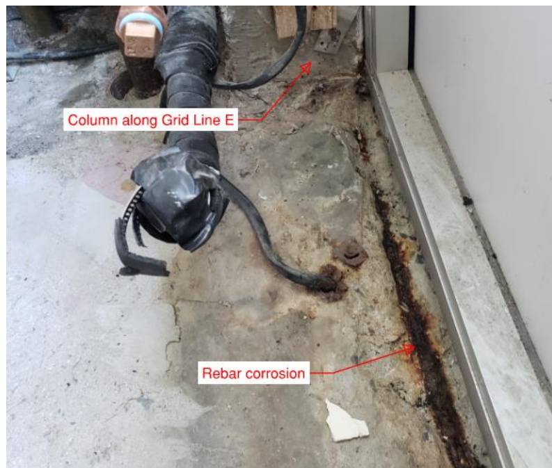
Figure 4: Concrete spalls and rebar corrosion near slab edge along Grid Line E.
