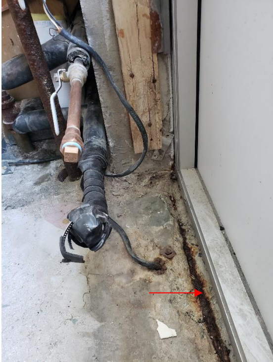
Photo 5: Concrete spalls and rebar corrosion near slab edge along Grid Line E.
