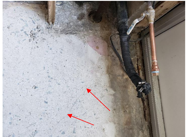
Photo 6: Hairline slab cracks in vicinity of a column along Grid Line E.
