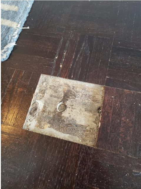
Photo 5. View of thin floor finish inside Unit 705 with exposed concrete floor slab.
