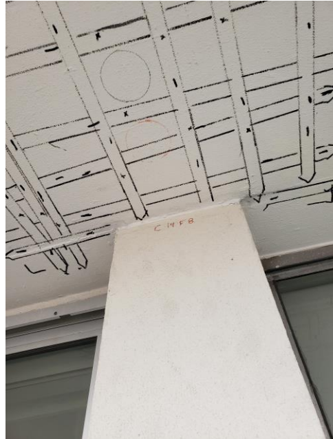
Photo 2. Underside of 8 th Floor balcony slab near column B-14 (GPR markings by SGH).
