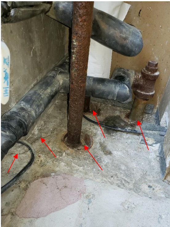
Photo 7: Typical slab-to-column connection exhibiting core holes and cracks around a column.
