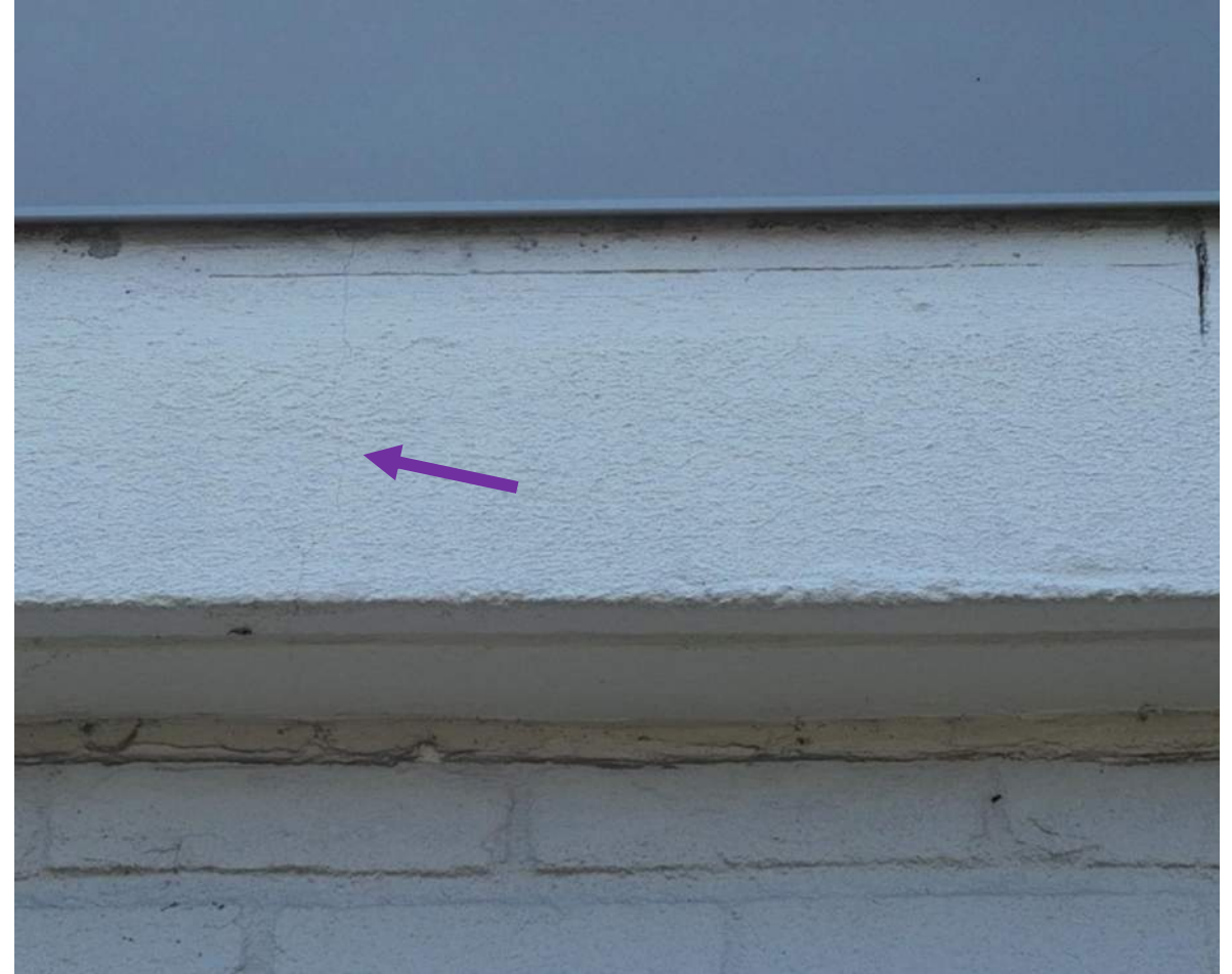
21 April 2025 Drone Survey, IMG#302
