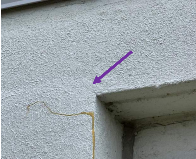
18 June 2024 Drone Survey, IMG#10-092
