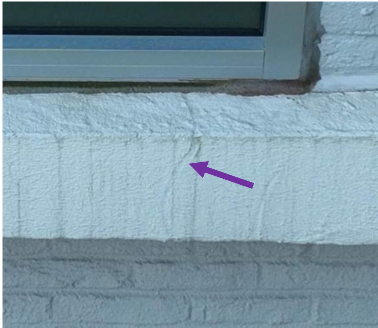
18 June Drone Survey, IMG#3-020
