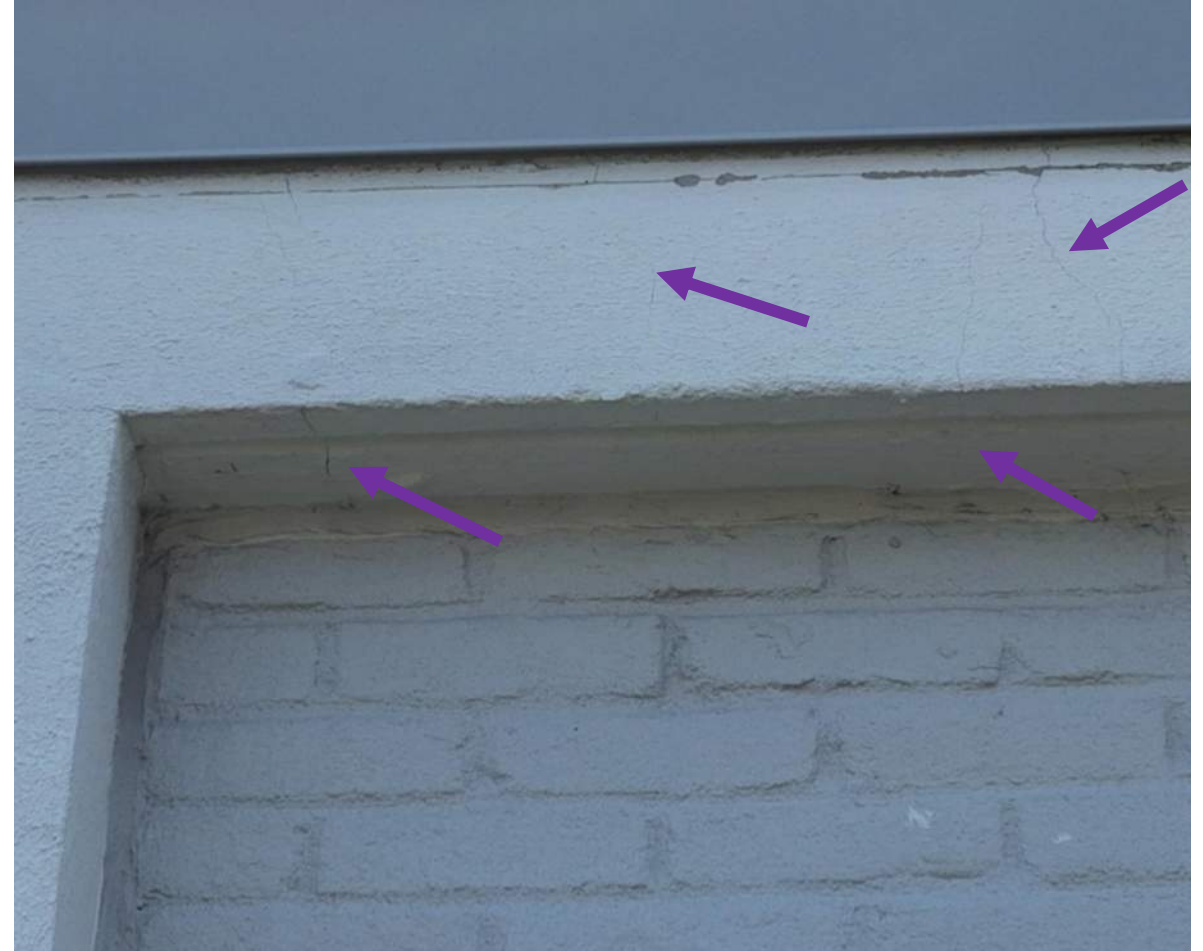
21 April 2025 Drone Survey, IMG#206
