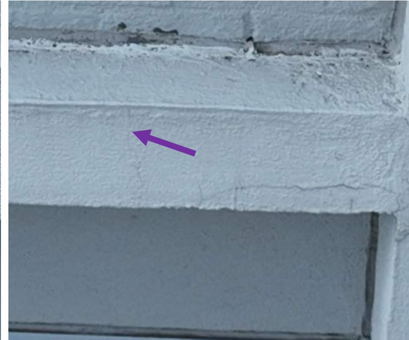
21 April 2025 Drone Survey, IMG#72
