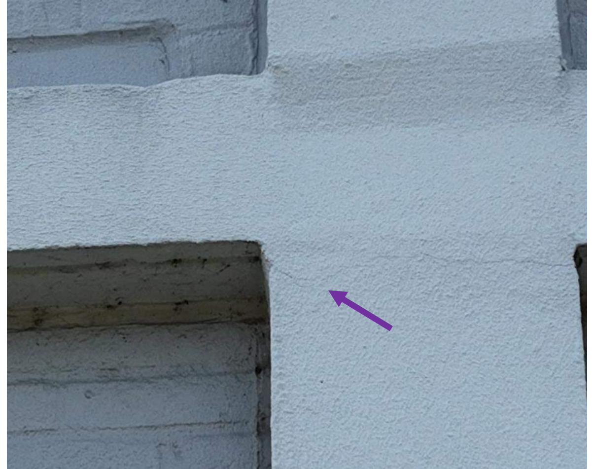
21 April 2025 Drone Survey, IMG 510
