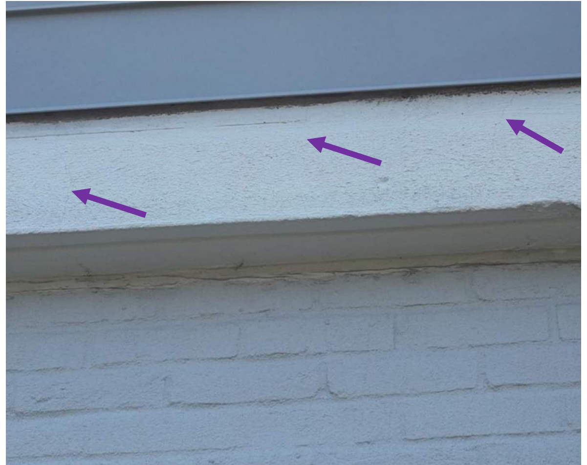
21 April 2025 Drone Survey, IMG#239
