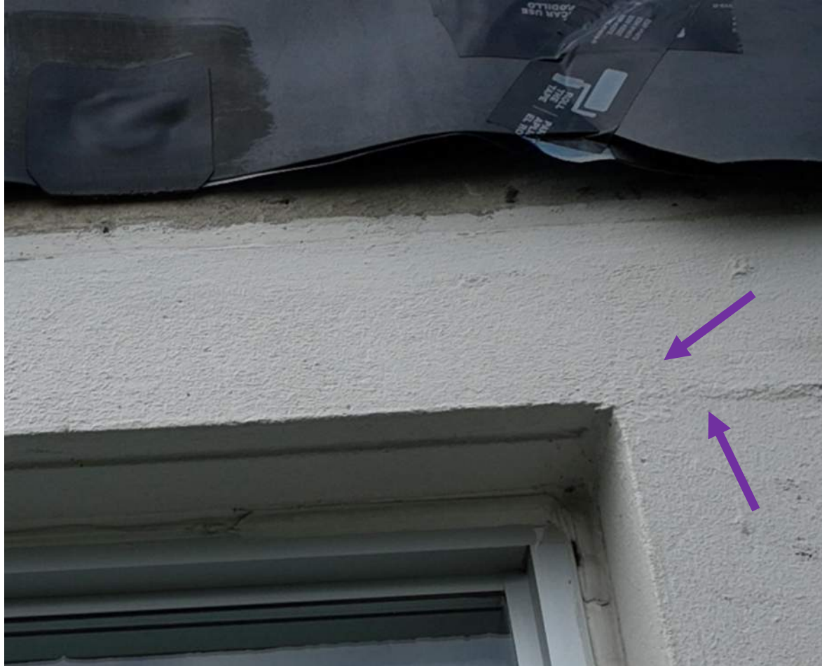
18 June 2024 Drone Survey, IMG#132
