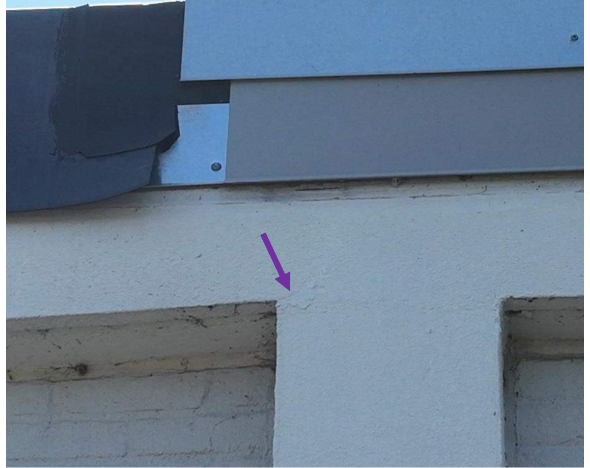
21 April 2025 Drone Survey, IMG 23
