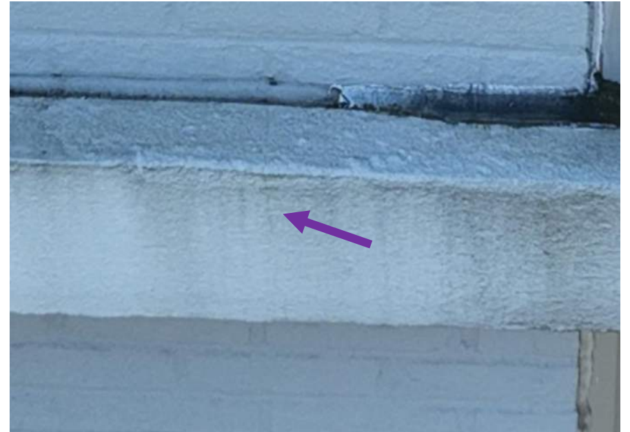
21 April 2025 Drone Survey, IMG#640
