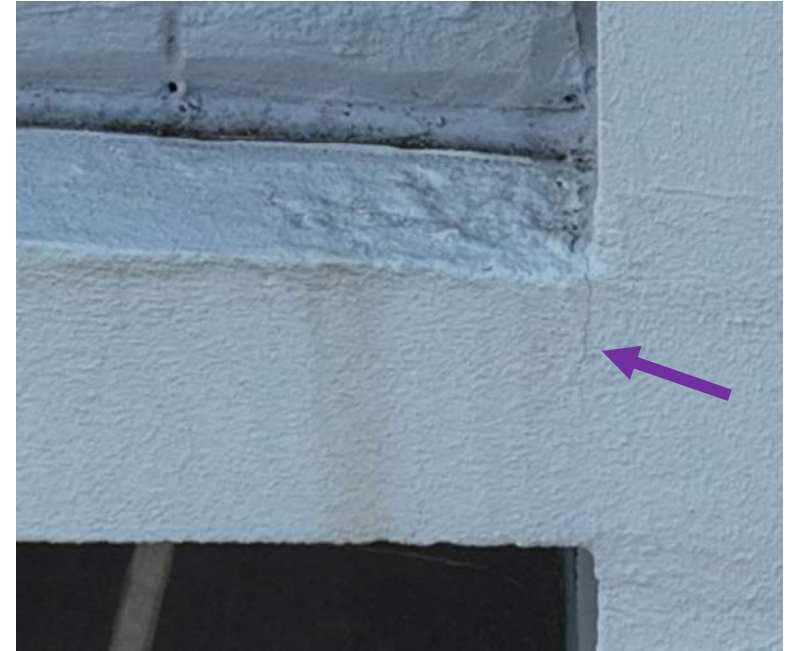
21 April 2025 Drone Survey, IMG#137
