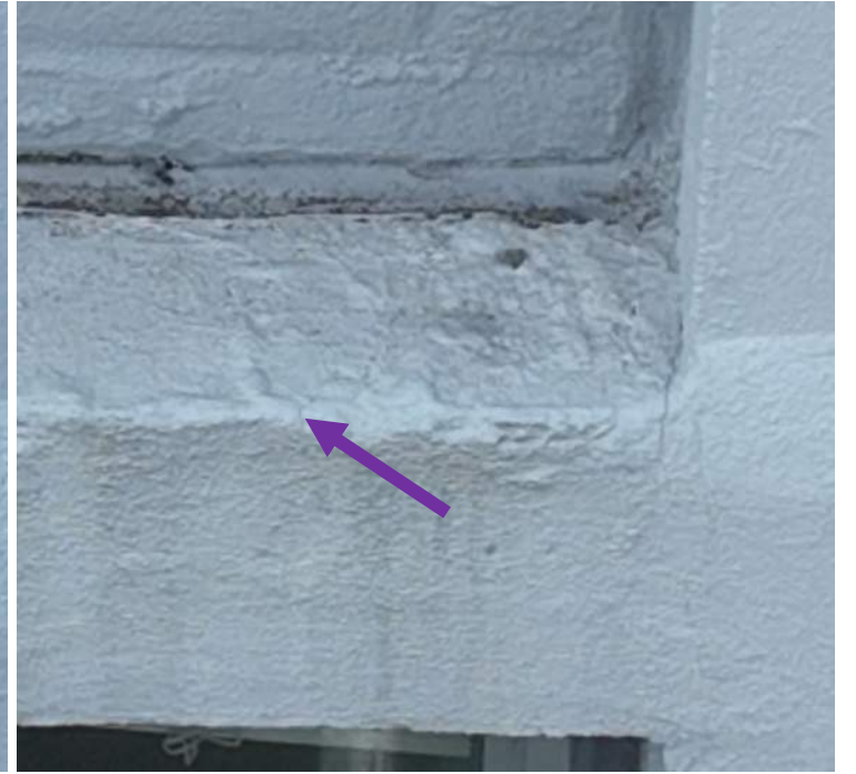
21 April 2025 Drone Survey, IMG#59
