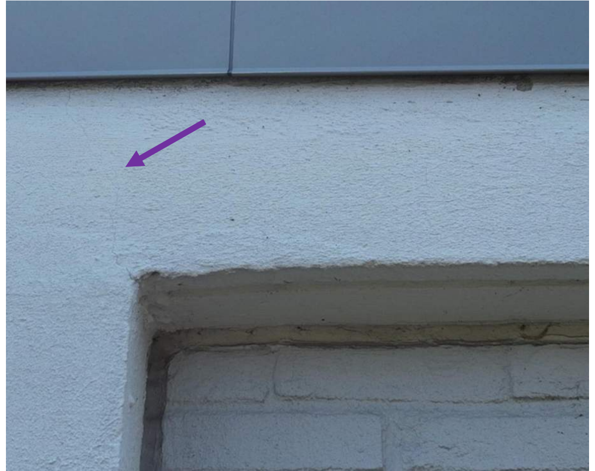
21 April 2025 Drone Survey, IMG#301
