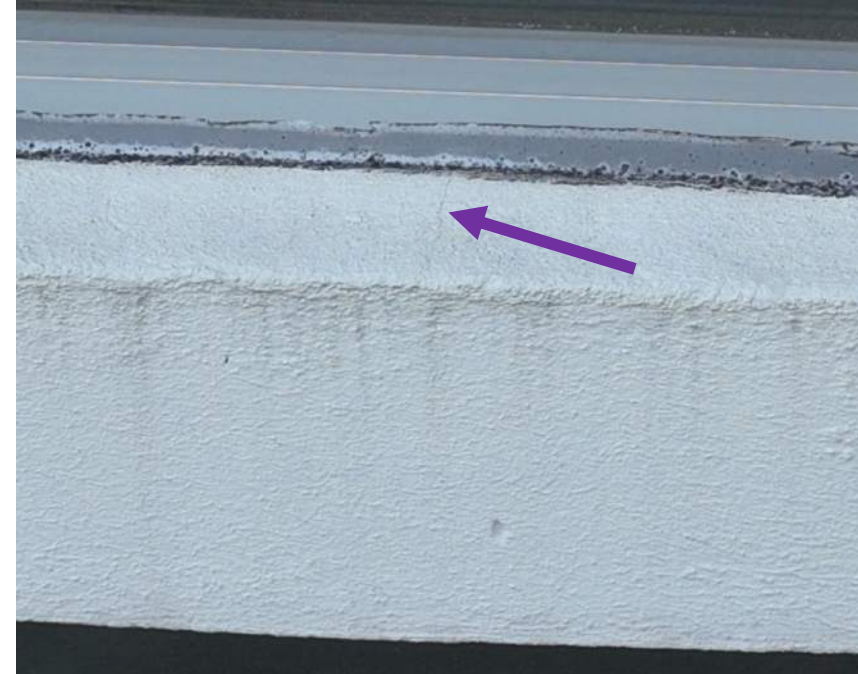
21 April 2025 Drone Survey, IMG#400
