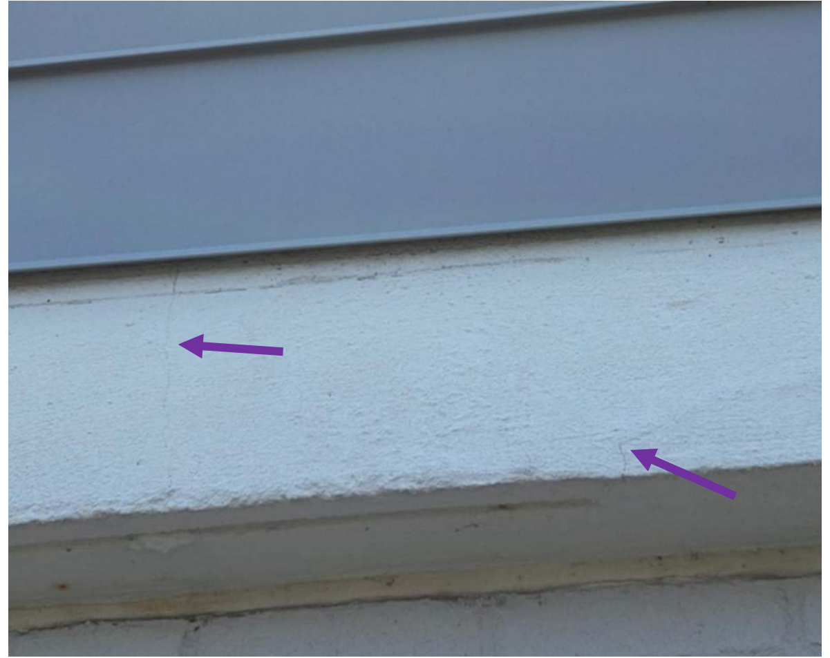
21 April 2025 Drone Survey, IMG#270
