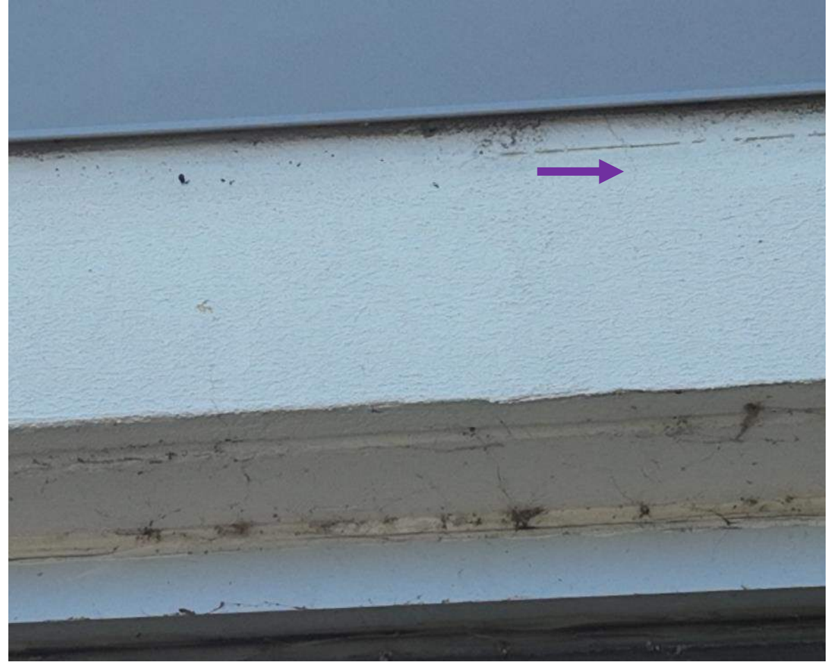
21 April 2025 Drone Survey, IMG 34
