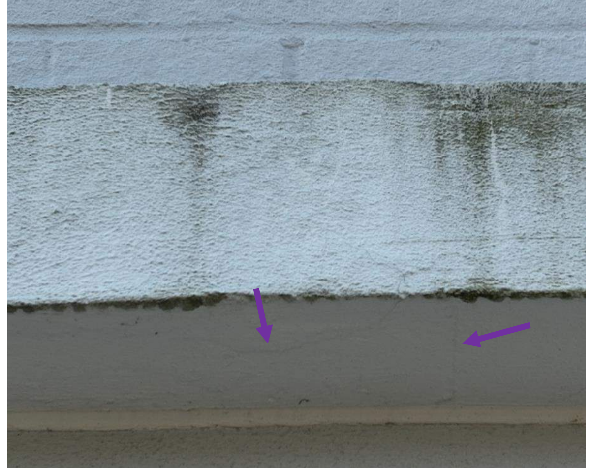
21 April 2025 Drone Survey, IMG 265
