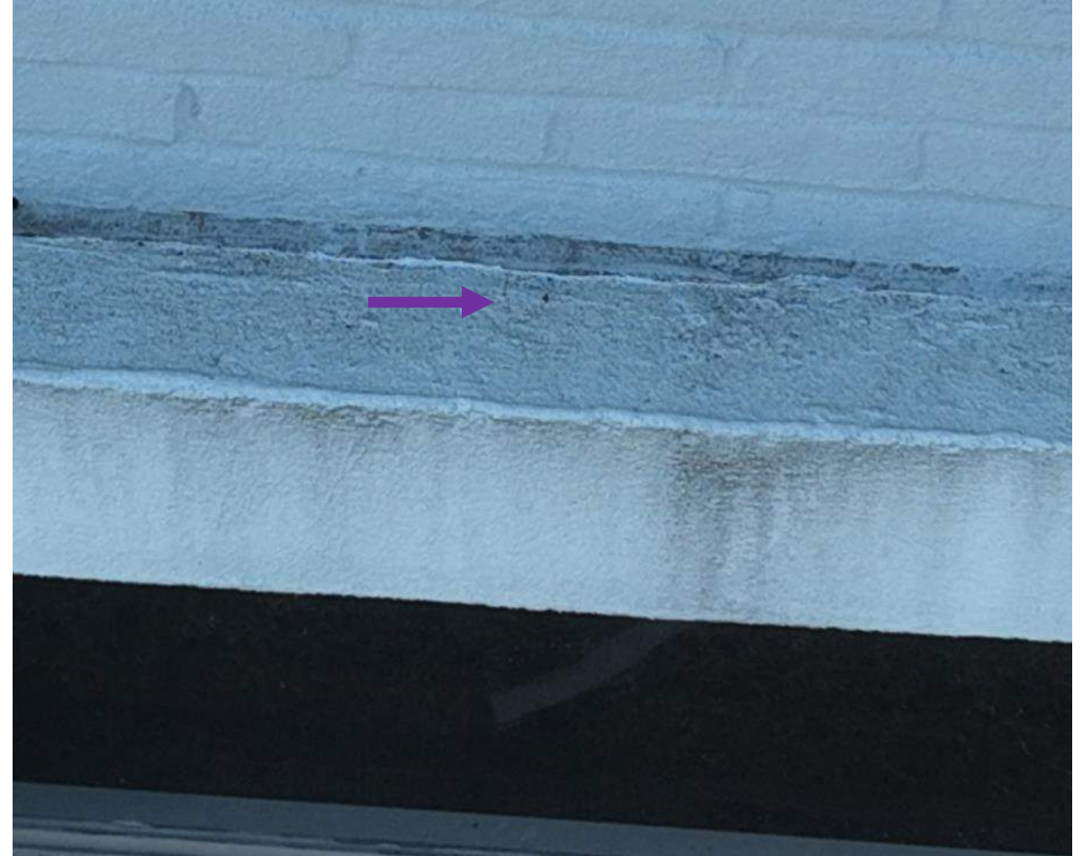
21 April 2025 Drone Survey, IMG 94
