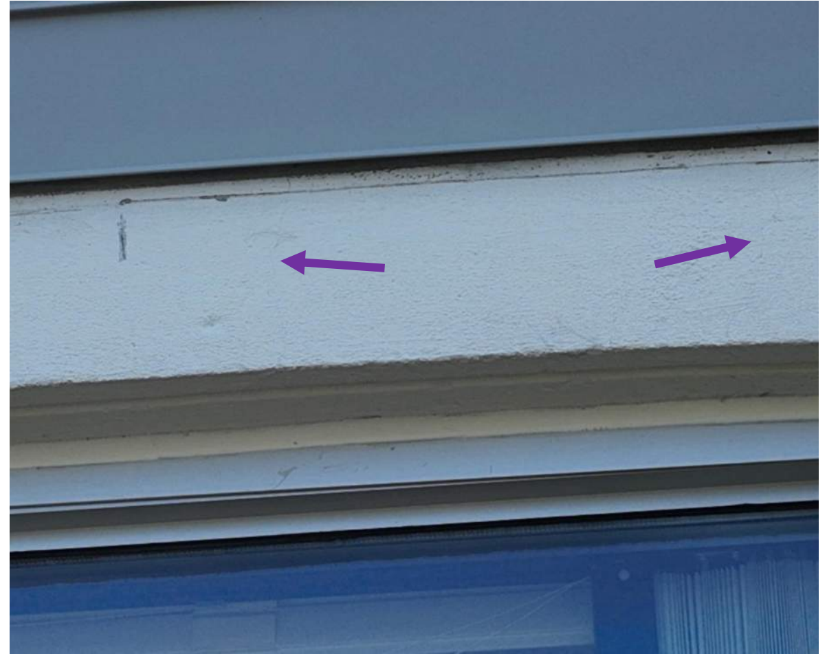
21 April 2025 Drone Survey, IMG#251
