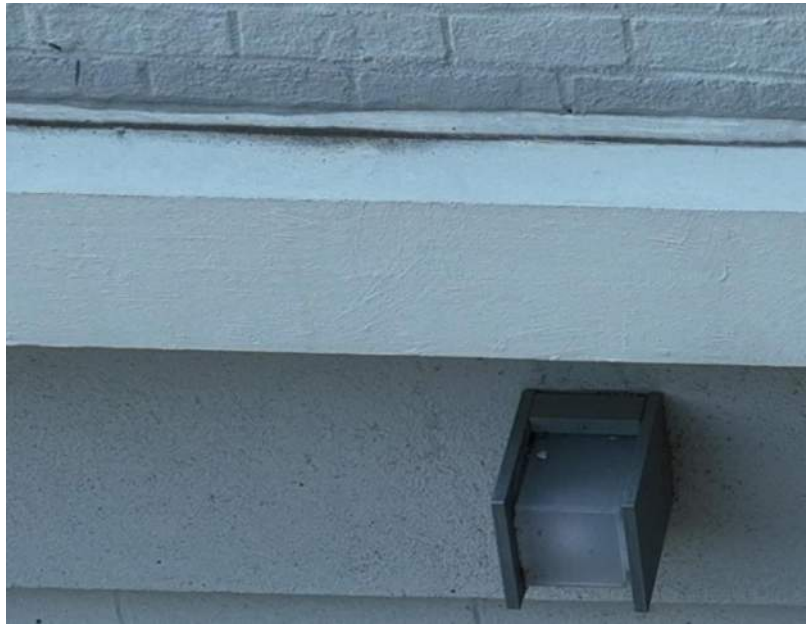
18 June Drone Survey, IMG#3-011
