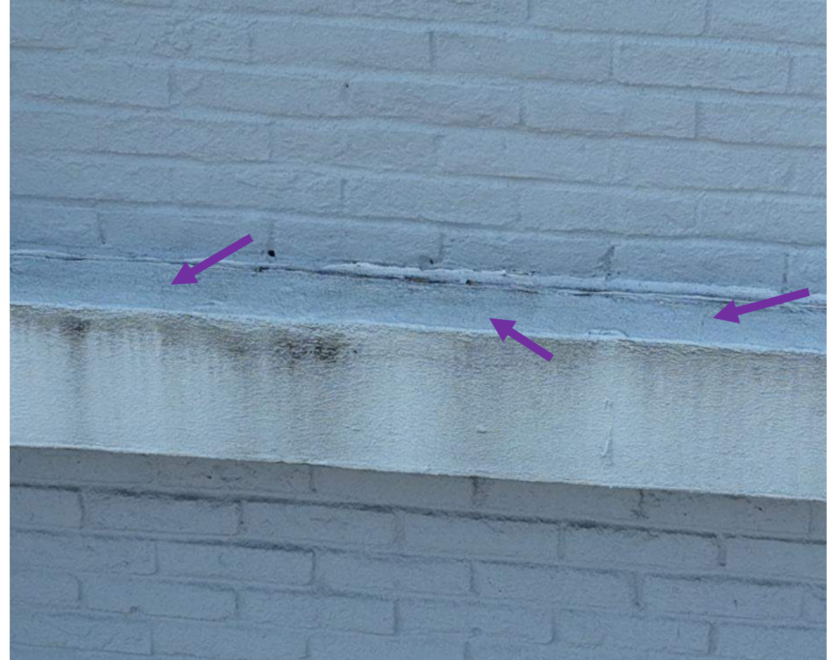
21 April 2025 Drone Survey, IMG 246
