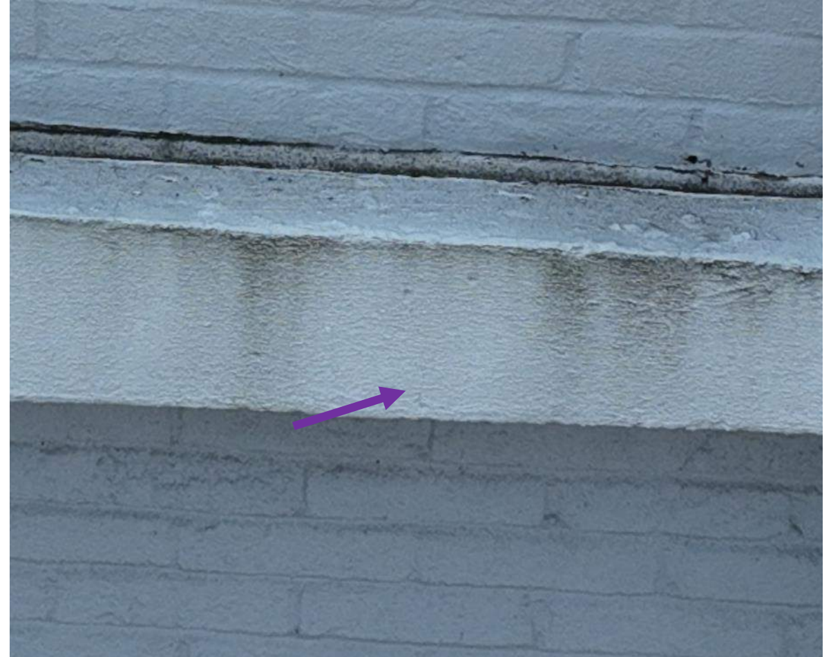
21 April 2025 Drone Survey, IMG 127
