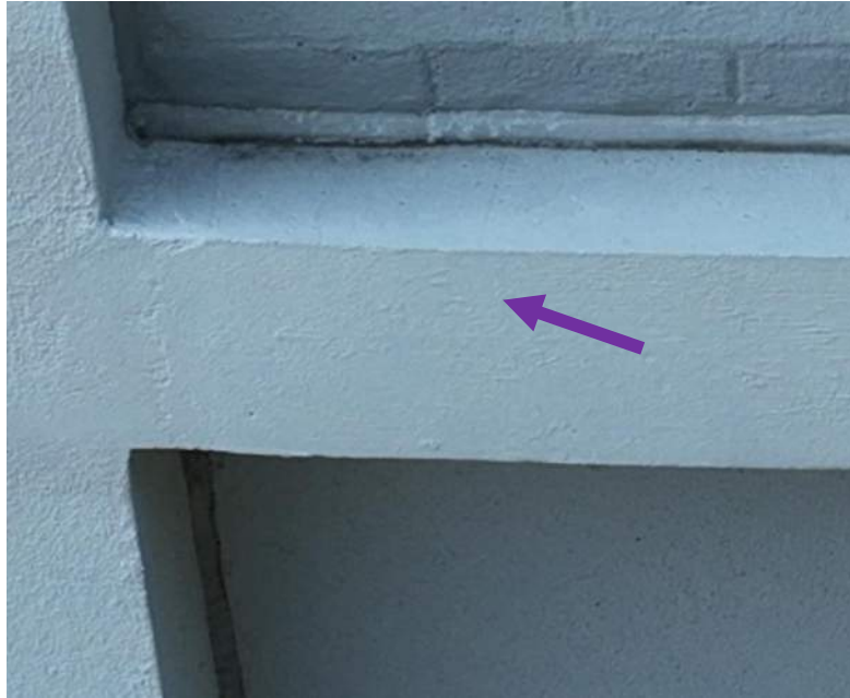
18 June Drone Survey, IMG#3-014
