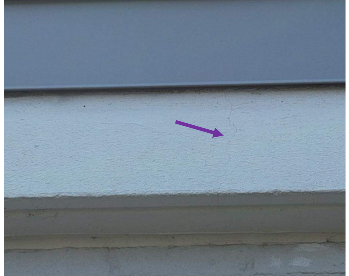
21 April 2025 Drone Survey, IMG 201
