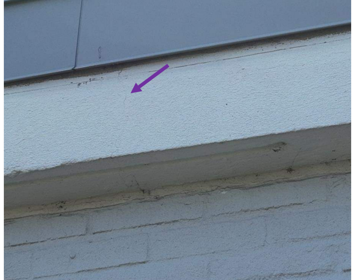
21 April 2025 Drone Survey, IMG 159
