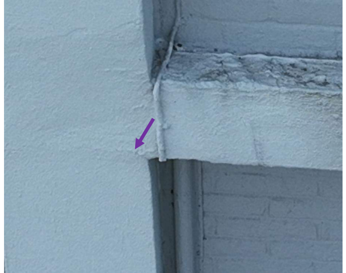
21 April 2025 Drone Survey, IMG 176
