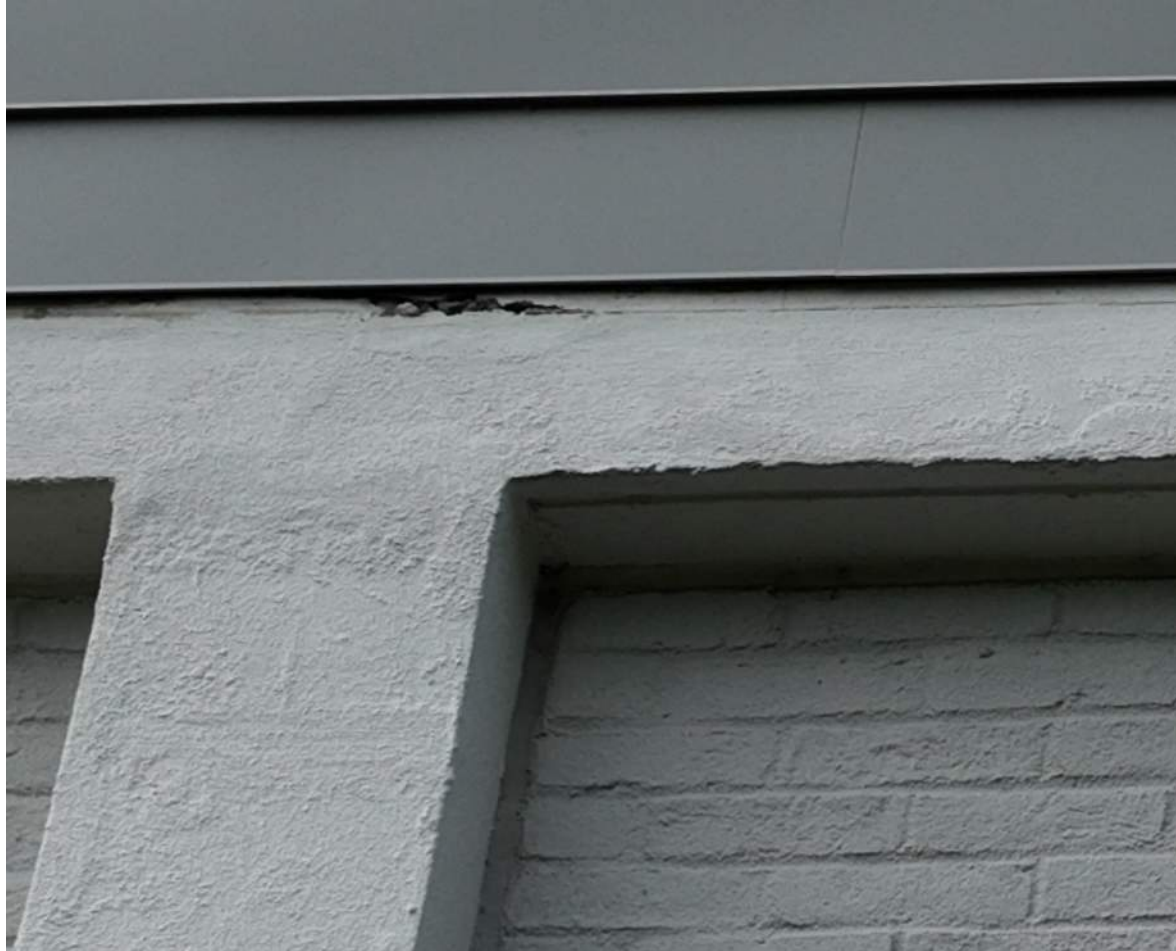
18 June 2024 Drone Survey, IMG#63
