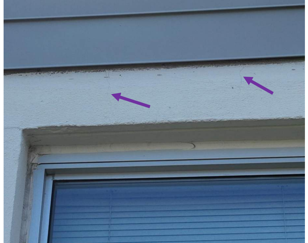
21 April 2025 Drone Survey, IMG#222
