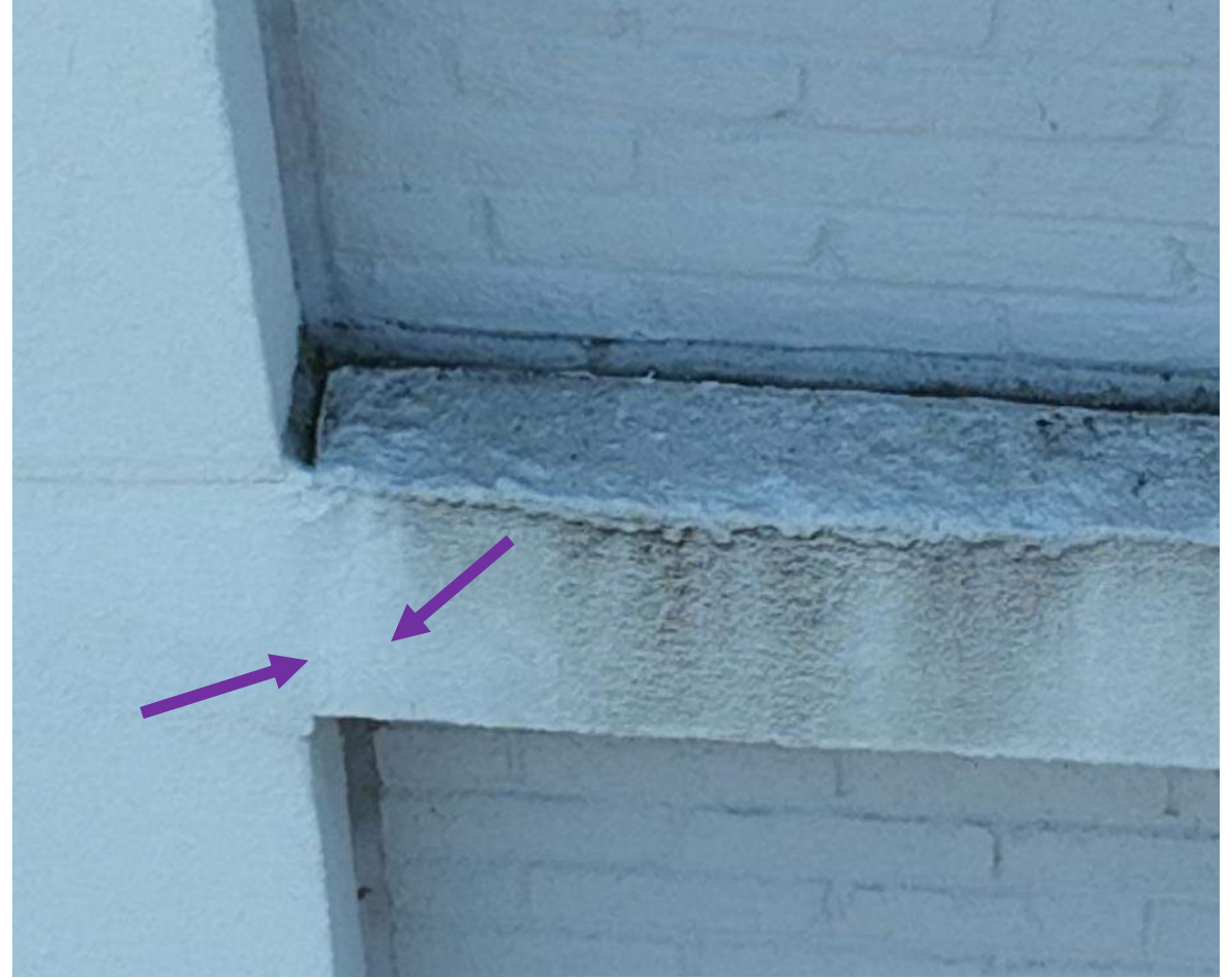
21 April 2025 Drone Survey, IMG 770
