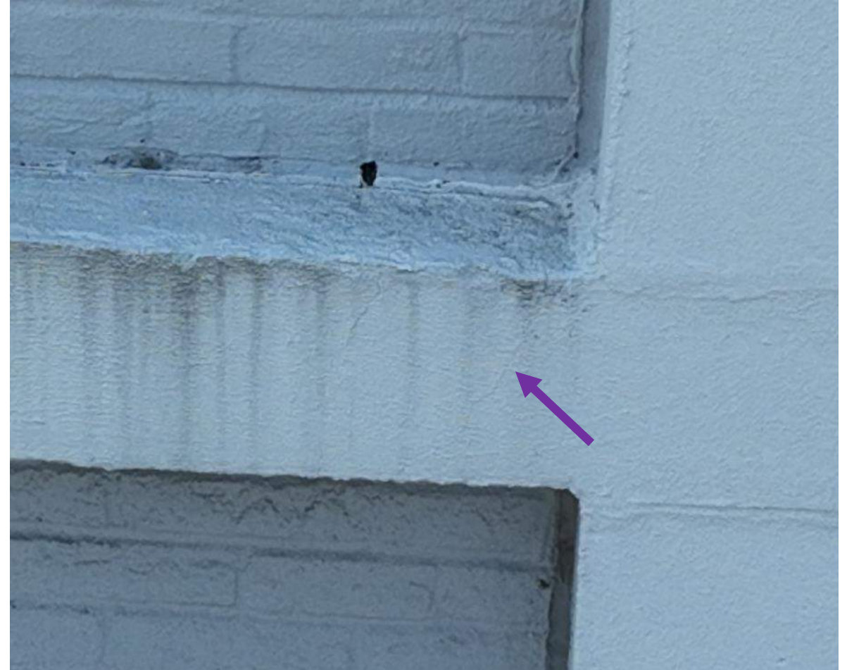
21 April 2025 Drone Survey, IMG 251
