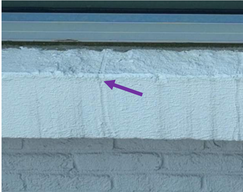
18 June 2024 Drone Survey, IMG#3-020
