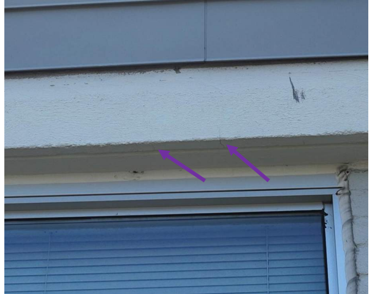
21 April 2025 Drone Survey, IMG#225
