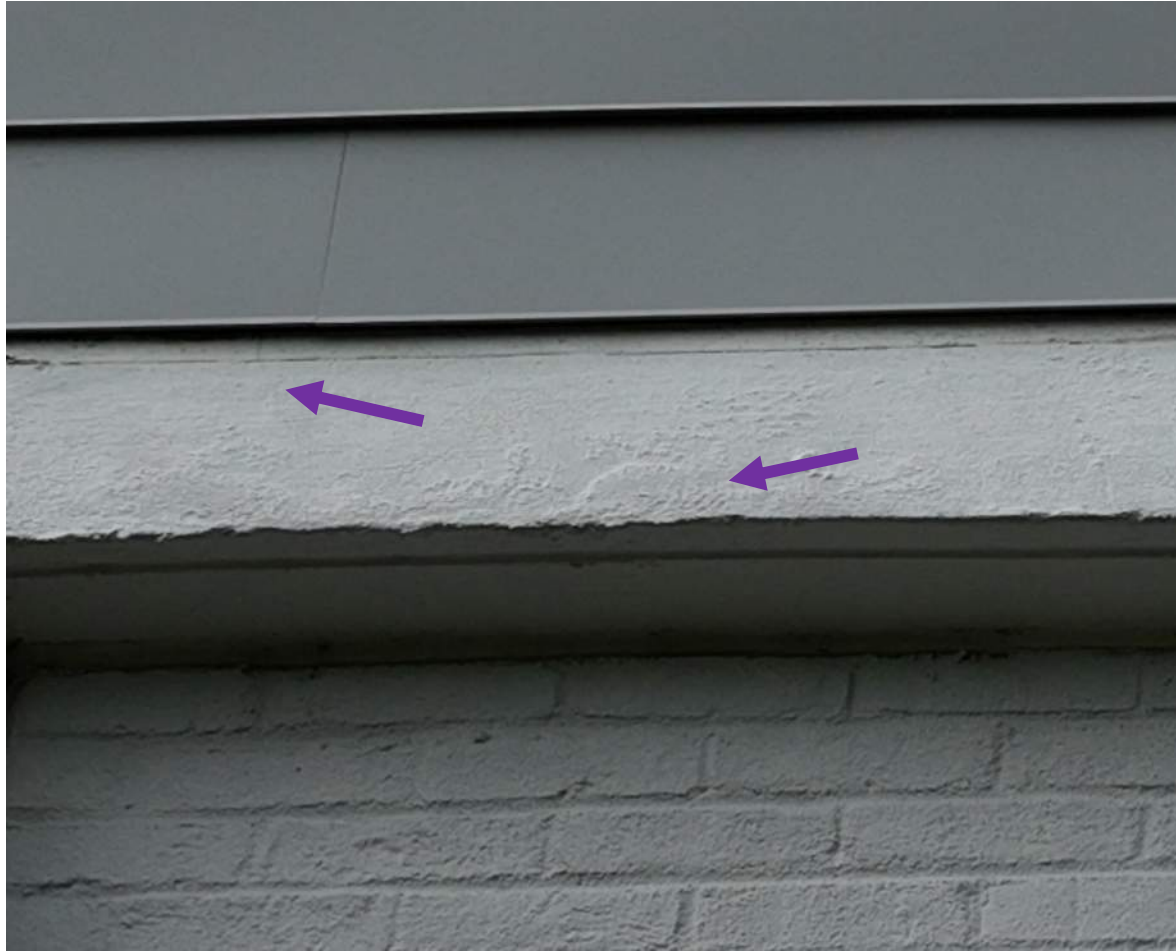
18 June 2024 Drone Survey, IMG#63
