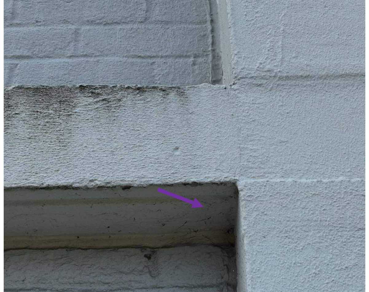
21 April 2025 Drone Survey, IMG 356
