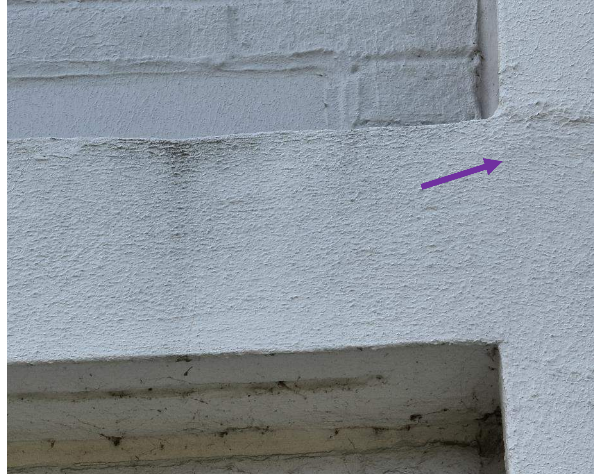
21 April 2025 Drone Survey, IMG 682
