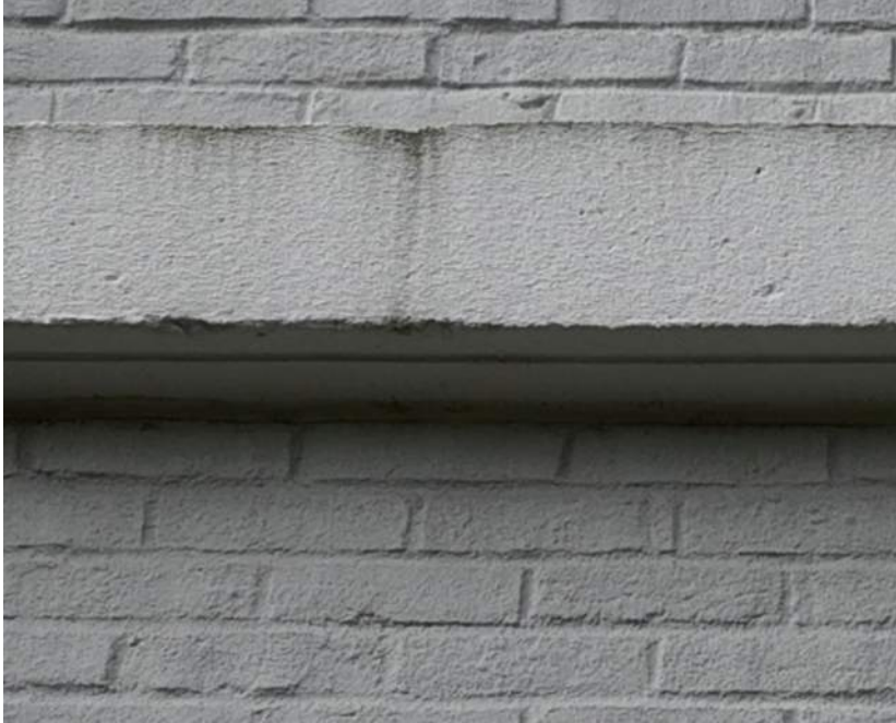
18 June 2024 Drone Survey, IMG#2-006
