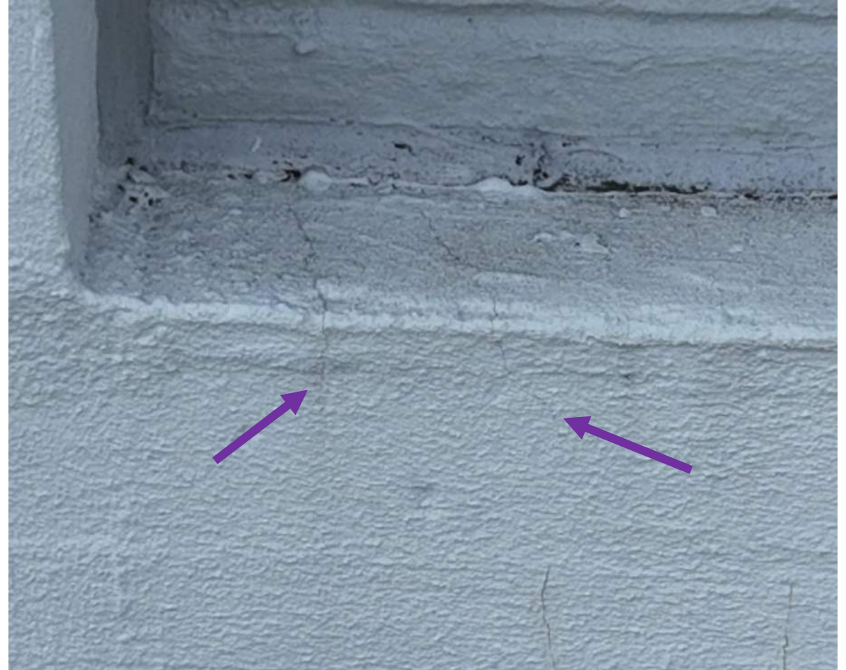
21 April 2025 Drone Survey, IMG#316
