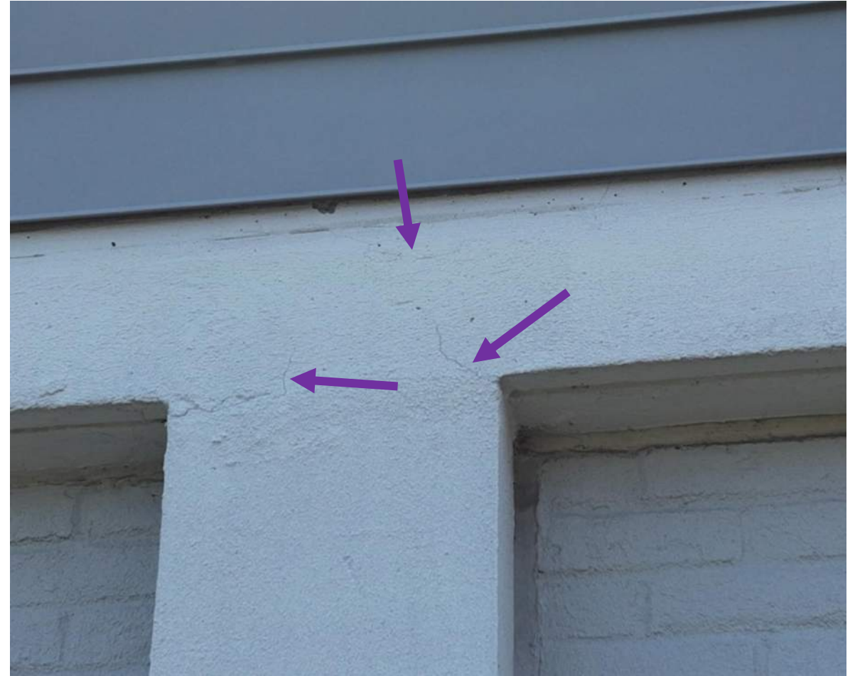
21 April 2025 Drone Survey, IMG#263
