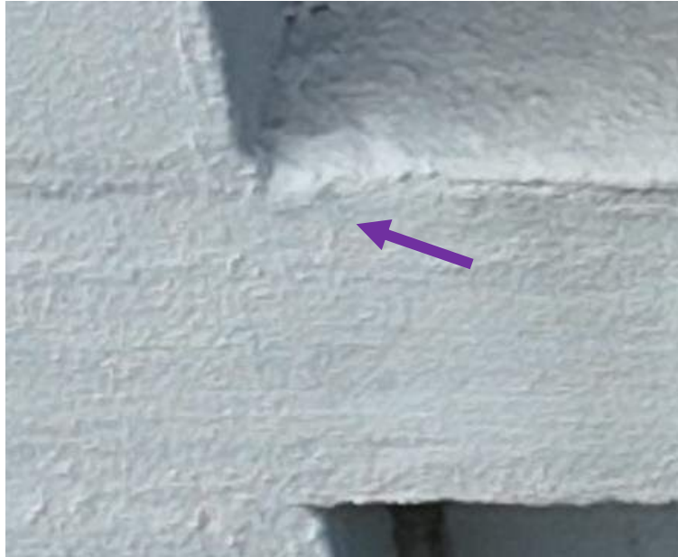
18 June 2024 Drone Survey, IMG#2-107
