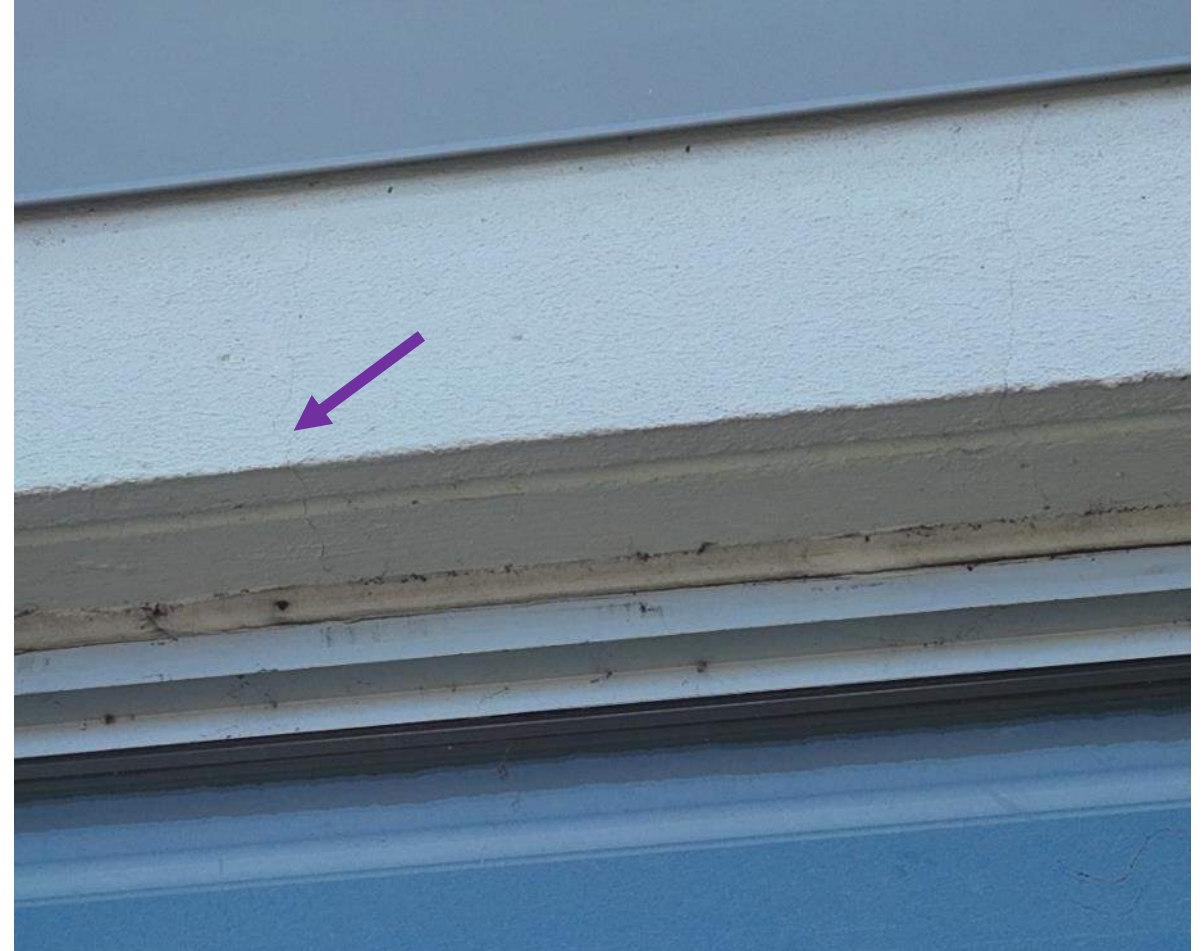
21 April 2025 Drone Survey, IMG 84
