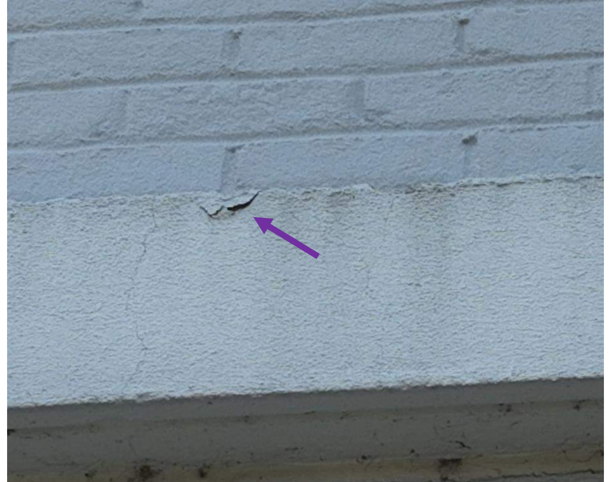
21 April 2025 Drone Survey, IMG 0511
