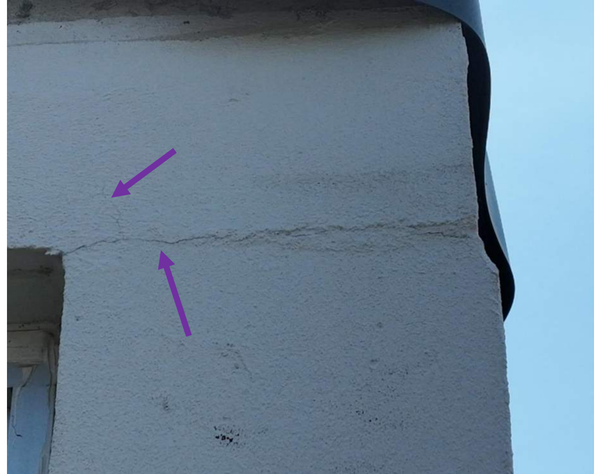
21 April 2025 Drone Survey, IMG#323
