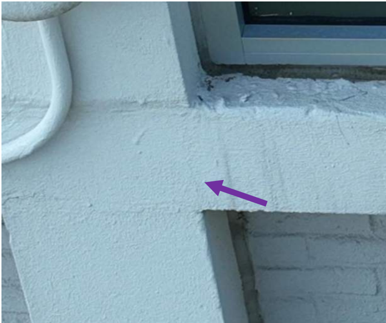
18 June Drone Survey, IMG#3-020
