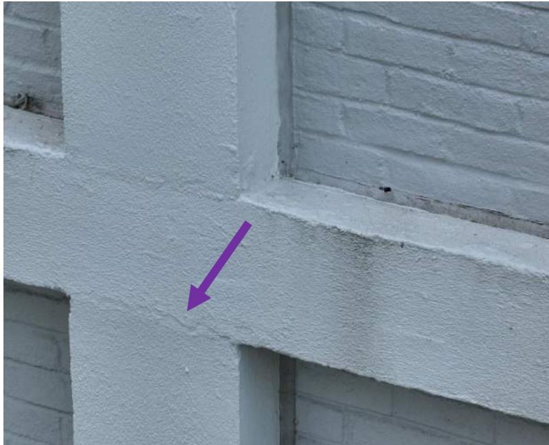
18 June 2024 Drone Survey, IMG#9-200
