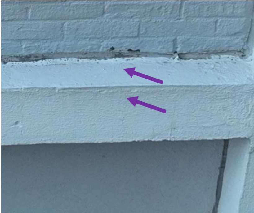
18 June Drone Survey, IMG#3-082
