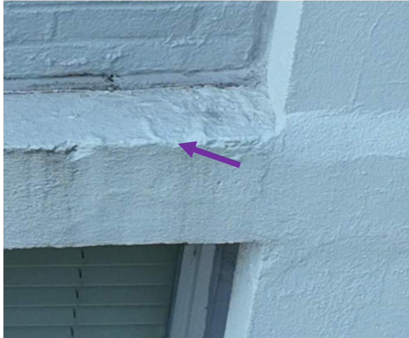
18 June Drone Survey, IMG#3-077
