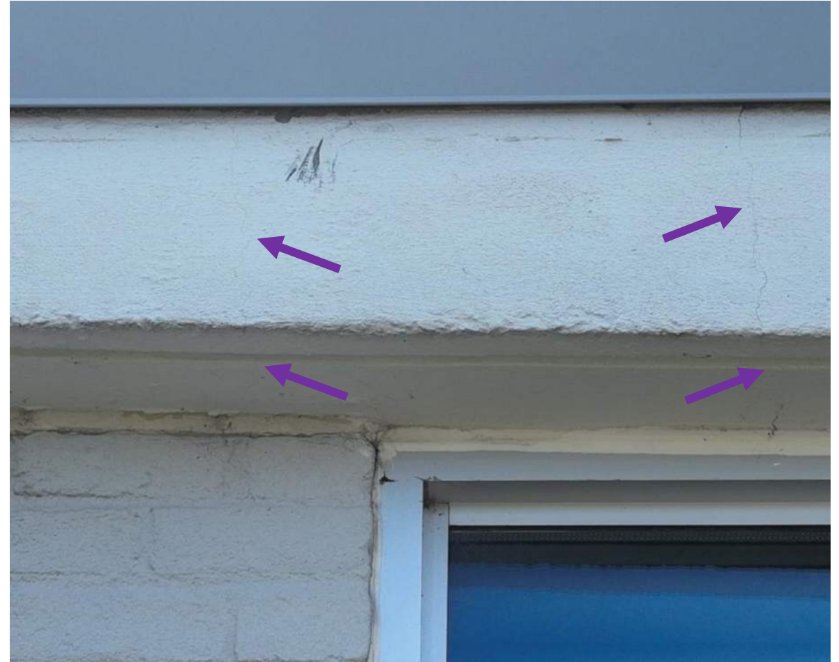
21 April 2025 Drone Survey, IMG#281
