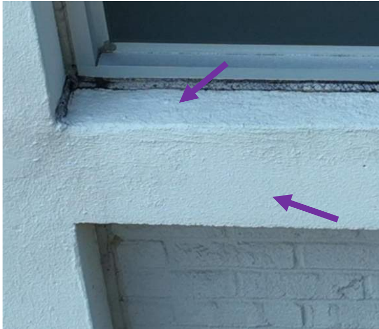
18 June 2024 Drone Survey, IMG#3-015
