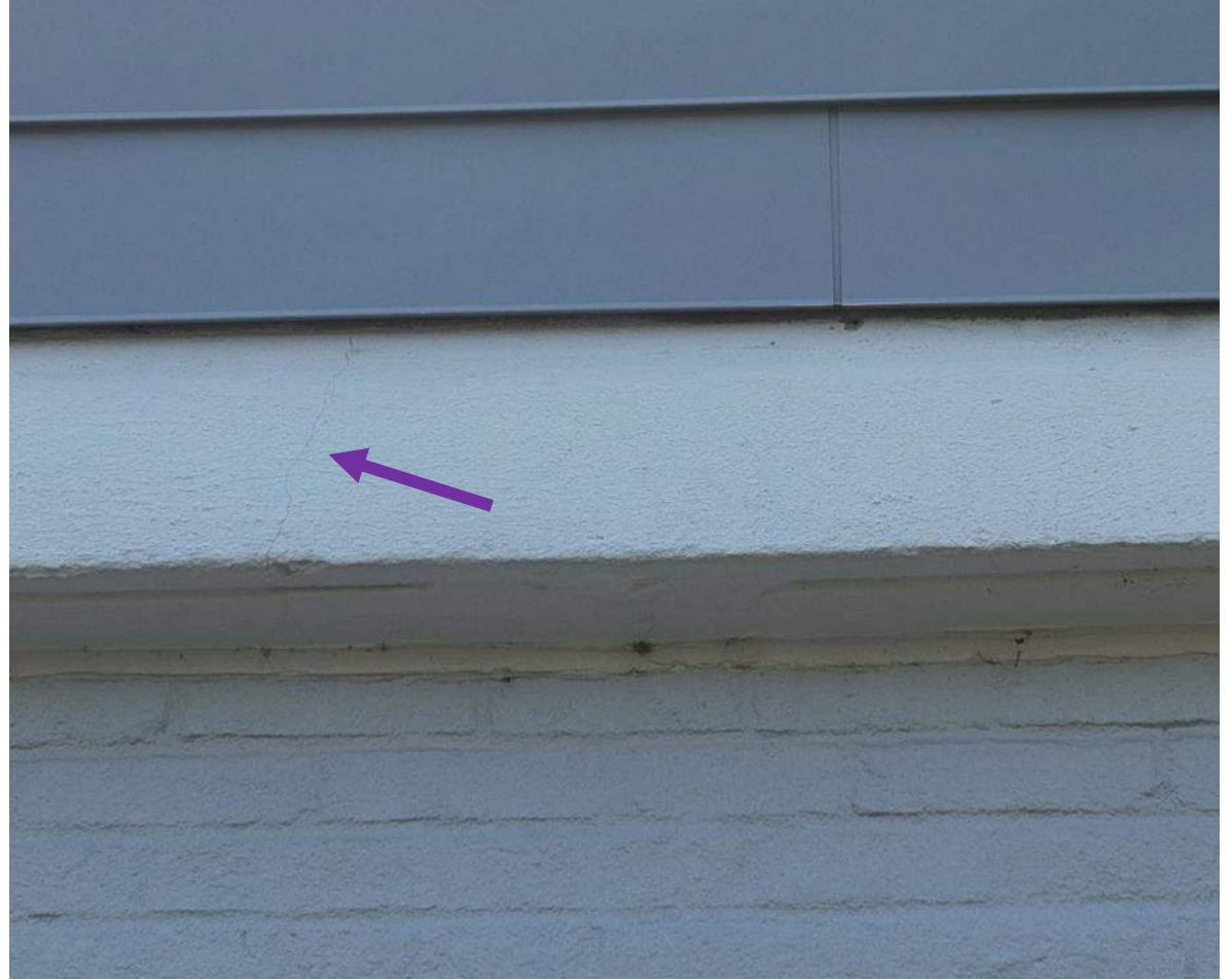
21 April 2025 Drone Survey, IMG 199
