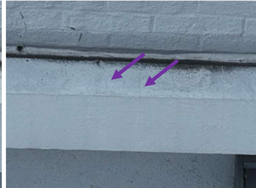
21 April 2025 Drone Survey, IMG#64
