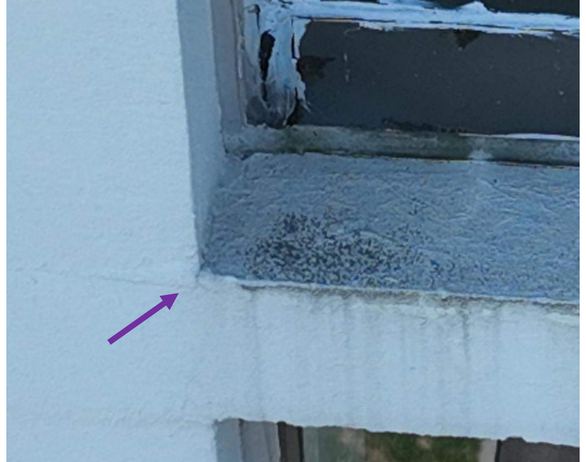
21 April 2025 Drone Survey, IMG 764
