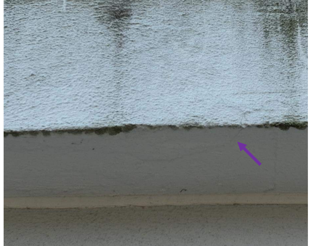
21 April 2025 Drone Survey, IMG 265
