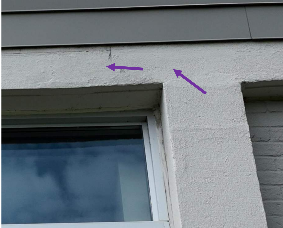
18 June 2024 Drone Survey, IMG#46
