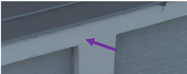
18 June Drone Survey, IMG#8-132, 8-166
