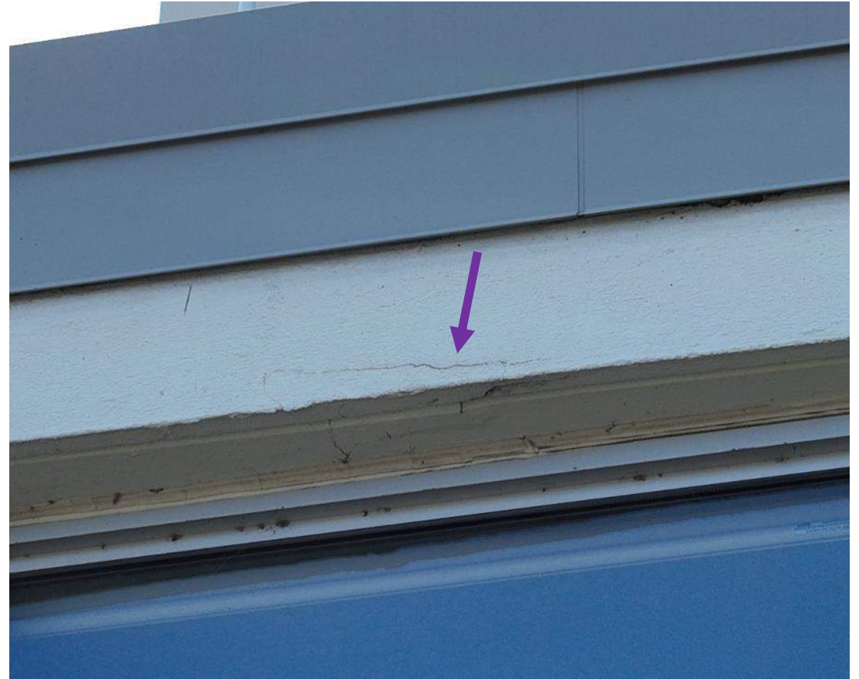
21 April 2025 Drone Survey, IMG 131
