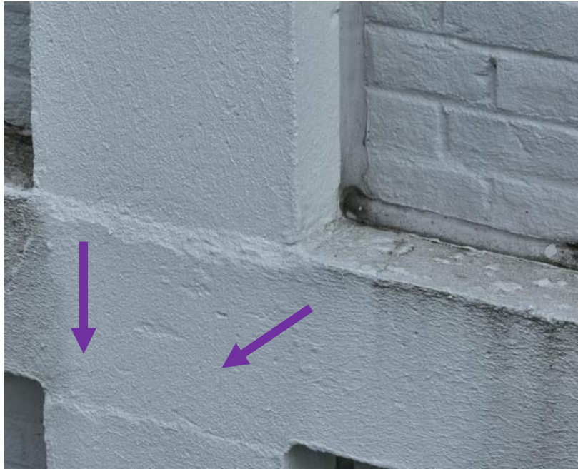
18 June 2024 Drone Survey, IMG#11-095
