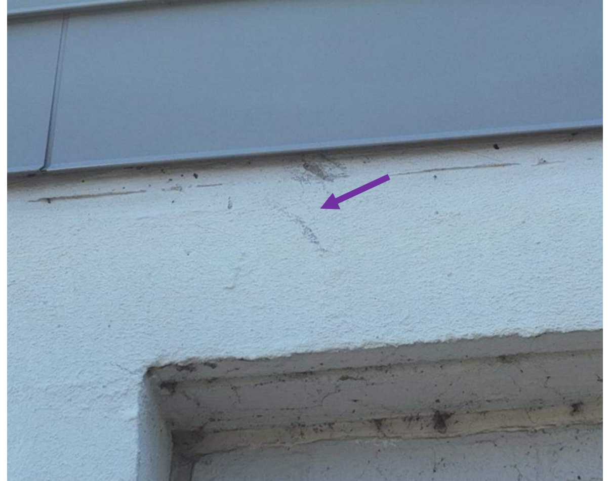
21 April 2025 Drone Survey, IMG 47
