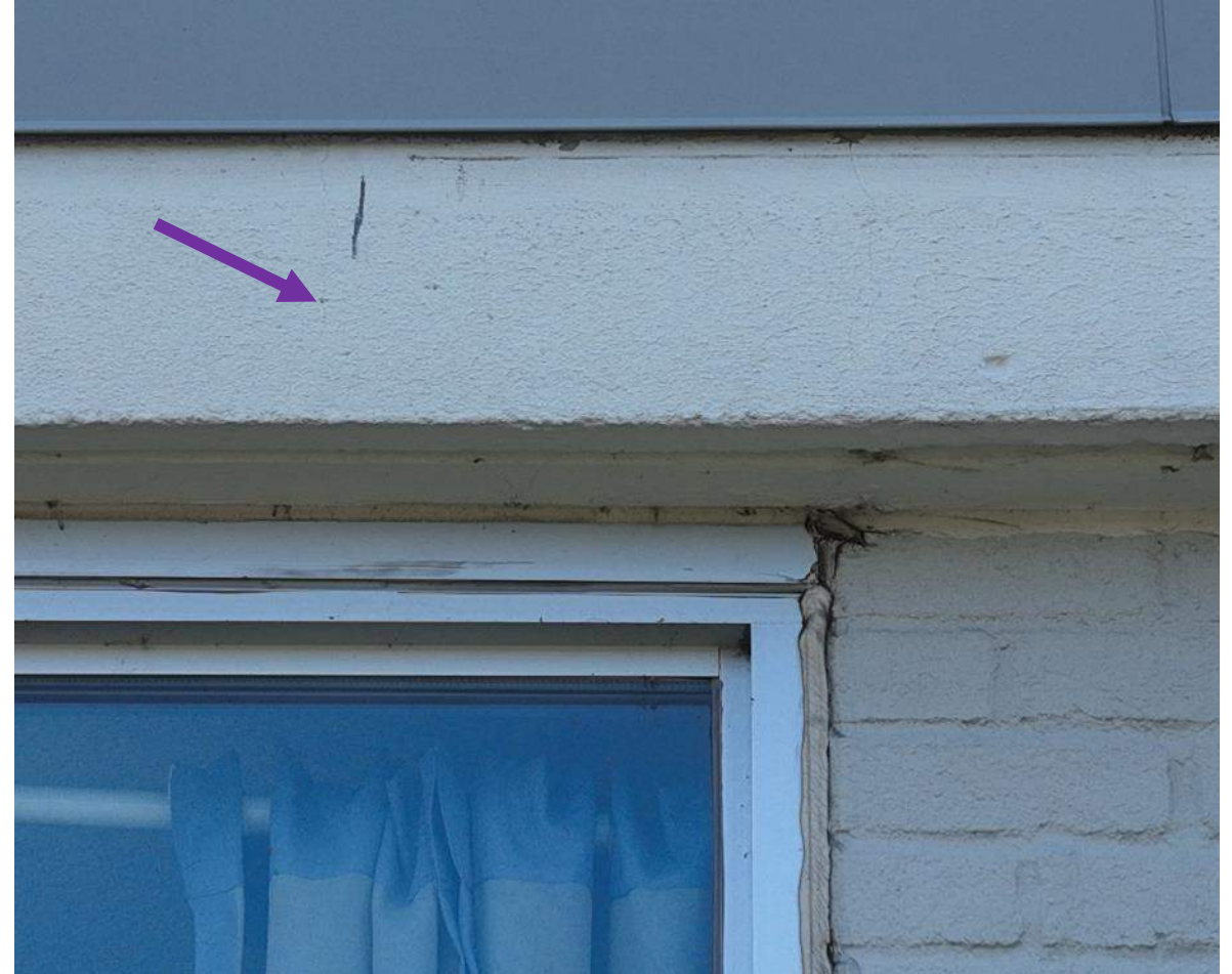
21 April 2025 Drone Survey, IMG 186
