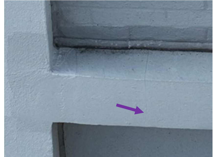
21 April 2025 Drone Survey, IMG#65
