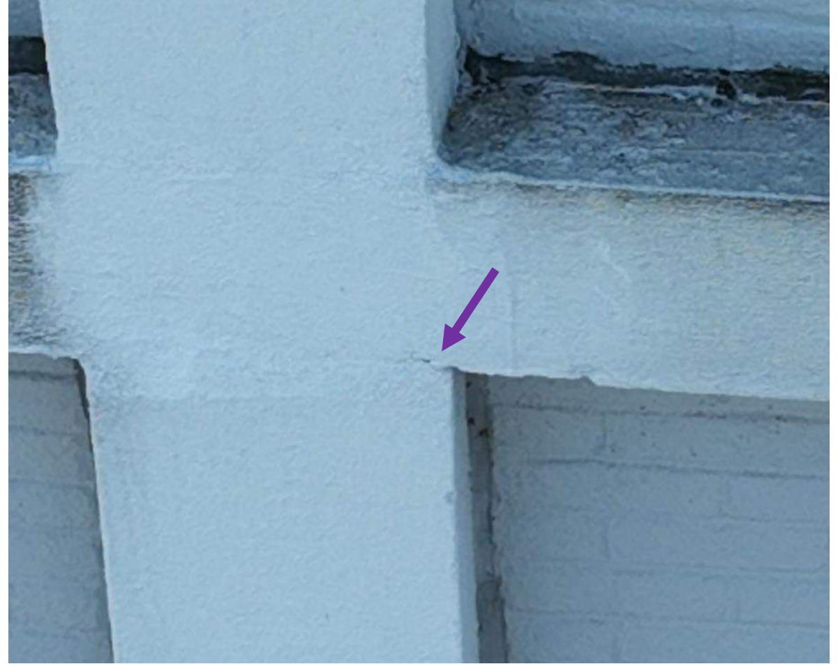
21 April 2025 Drone Survey, IMG 757
