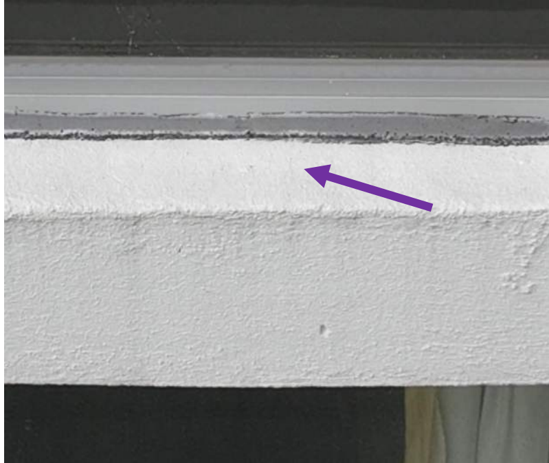
18 June 2024 Drone Survey, IMG#2-033
