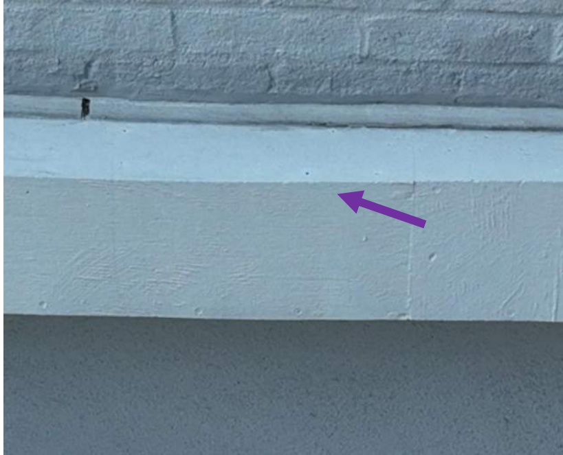
18 June 2024 Drone Survey, IMG#3-011
