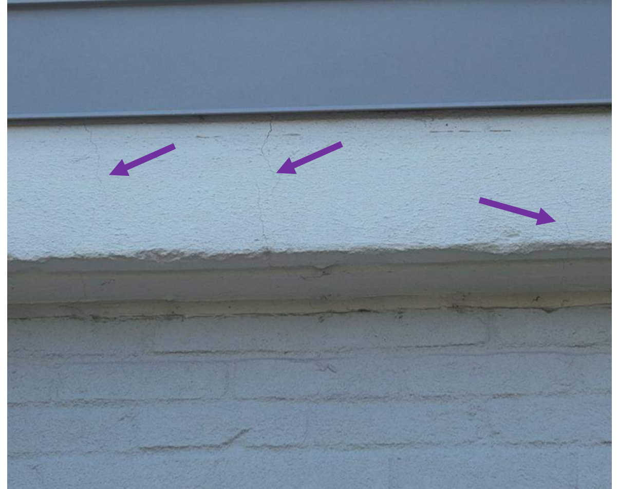
21 April 2025 Drone Survey, IMG 197
