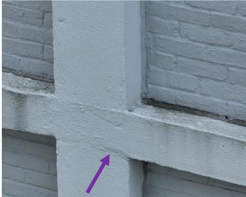
18 June 2024 Drone Survey, IMG#10-014
