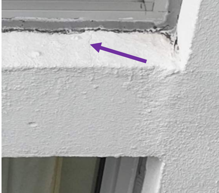
18 June 2024 Drone Survey, IMG#2-033
