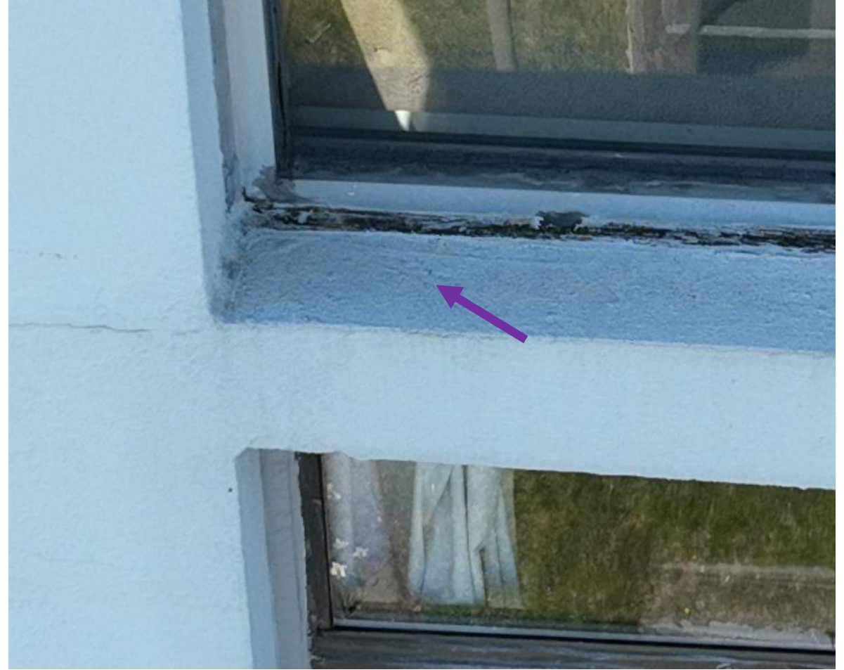
21 April 2025 Drone Survey, IMG 774
