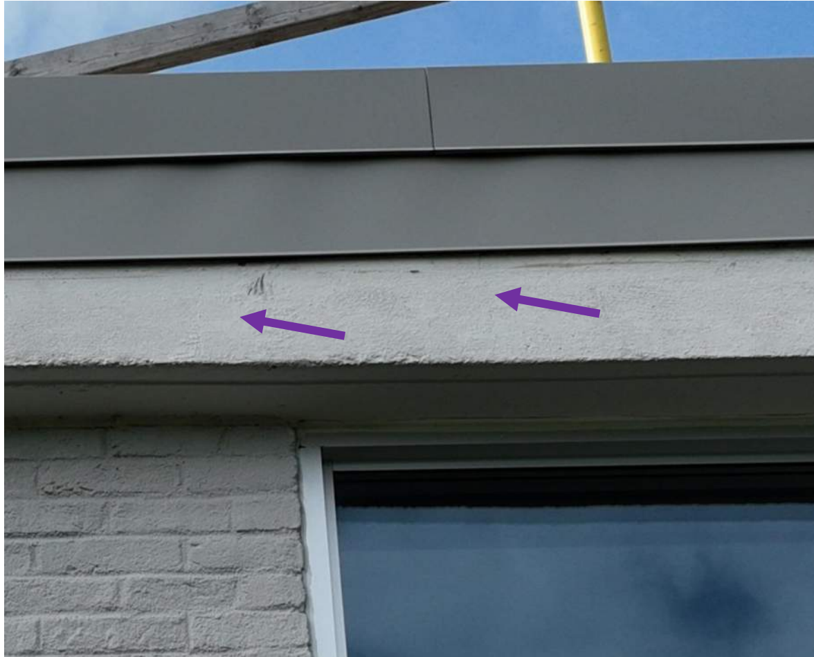
18 June 2024 Drone Survey, IMG#63
