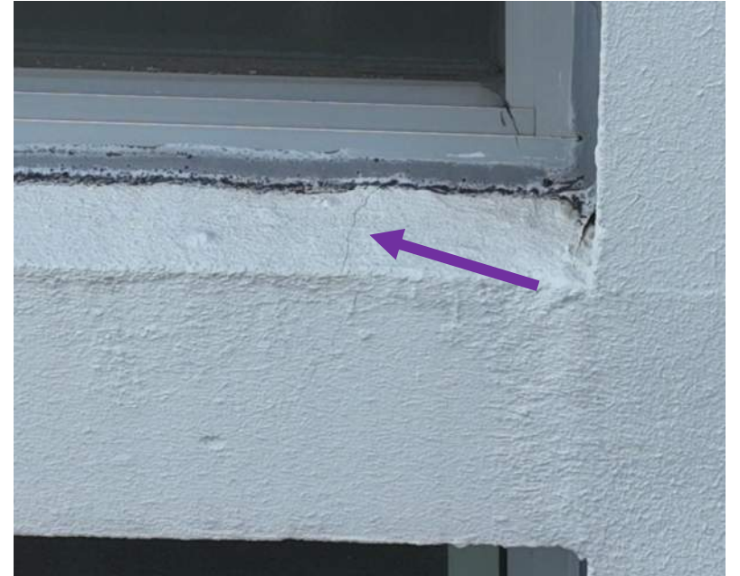
21 April 2025 Drone Survey, IMG#403
