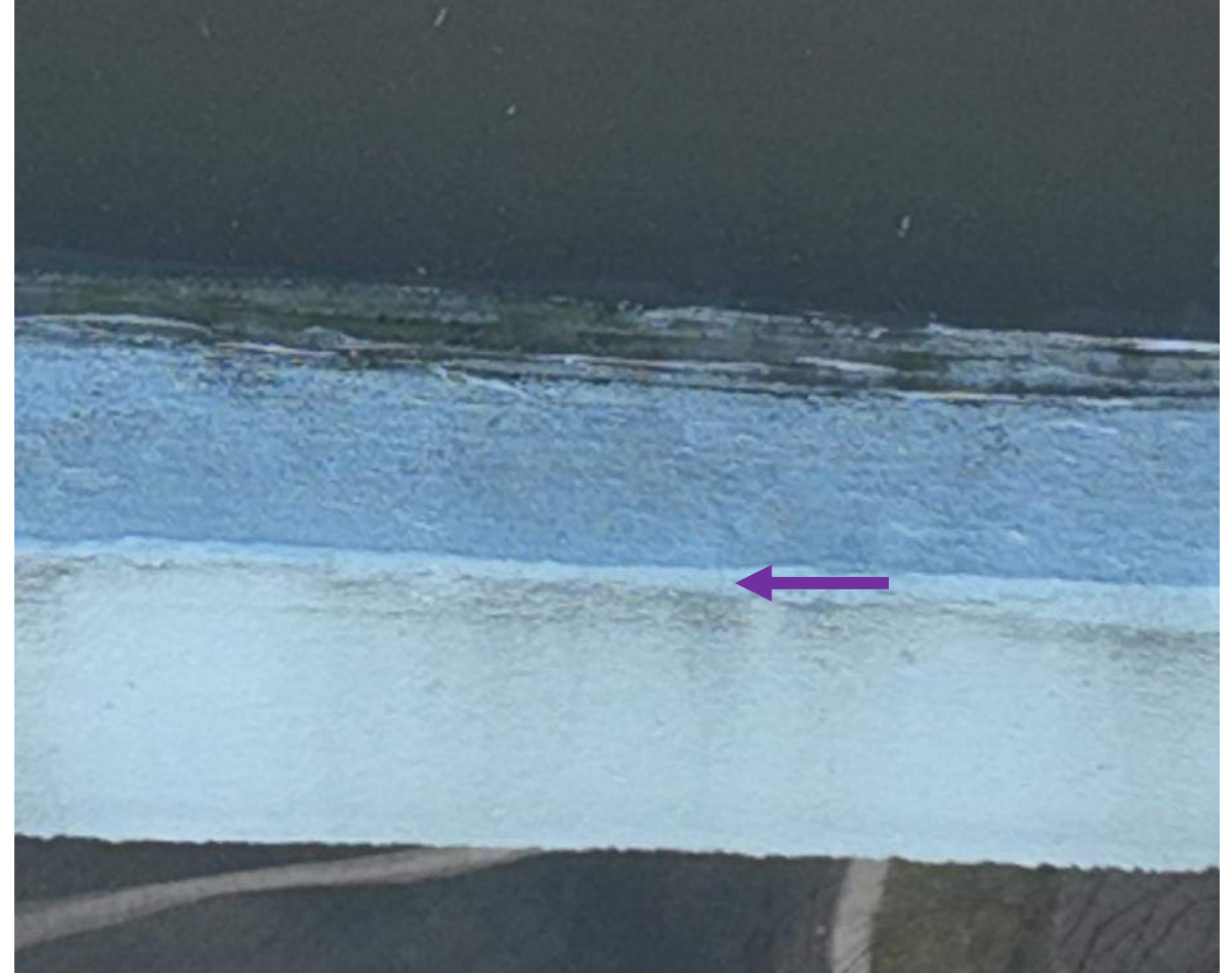
21 April 2025 Drone Survey, IMG 747
