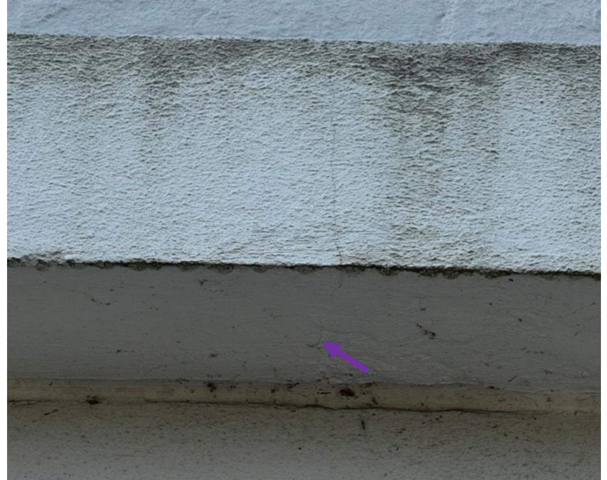
21 April 2025 Drone Survey, IMG 320
