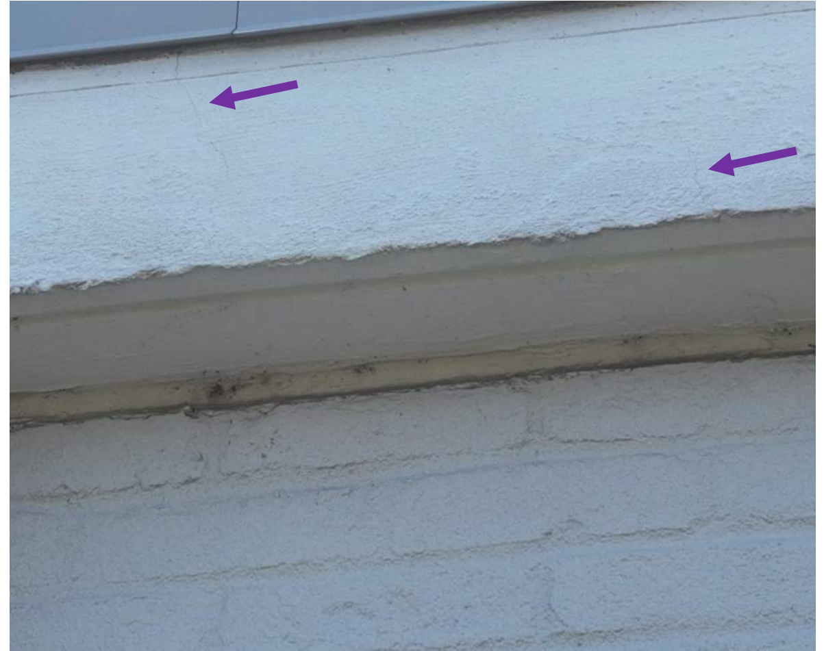
21 April 2025 Drone Survey, IMG#284
