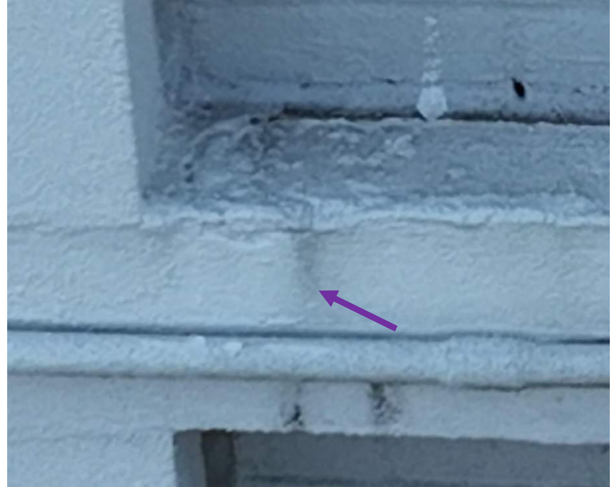
21 April 2025 Drone Survey, IMG#108
