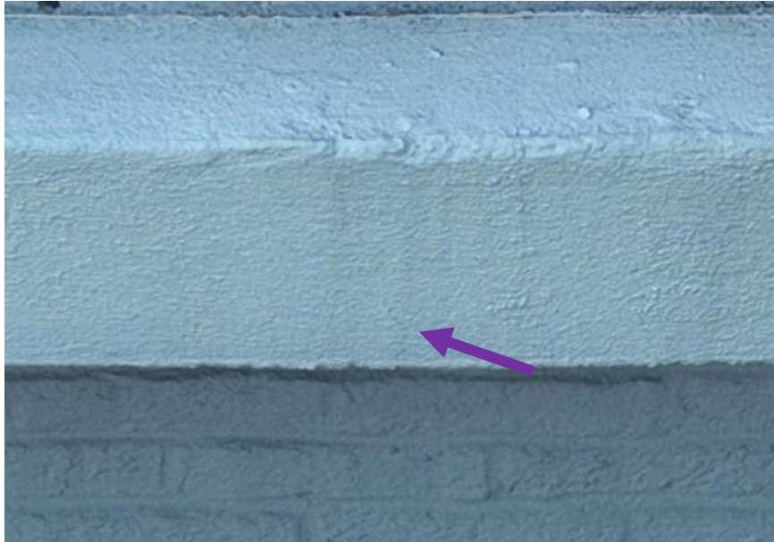
18 June Drone Survey, IMG#4-030
