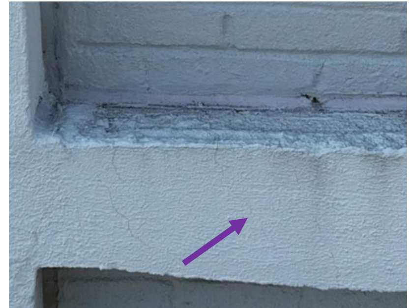
21 April 2025 Drone Survey, IMG#116
