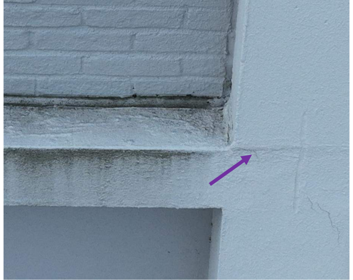
21 April 2025 Drone Survey, IMG 265
