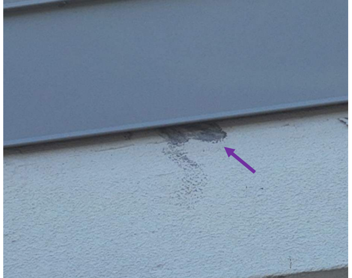
21 April 2025 Drone Survey, IMG 100
