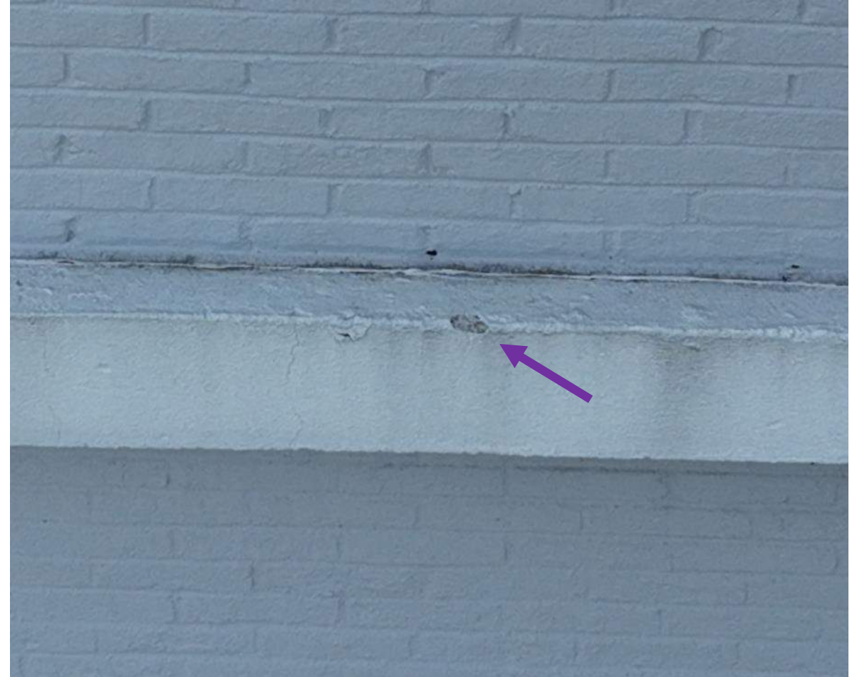
21 April 2025 Drone Survey, IMG 201
