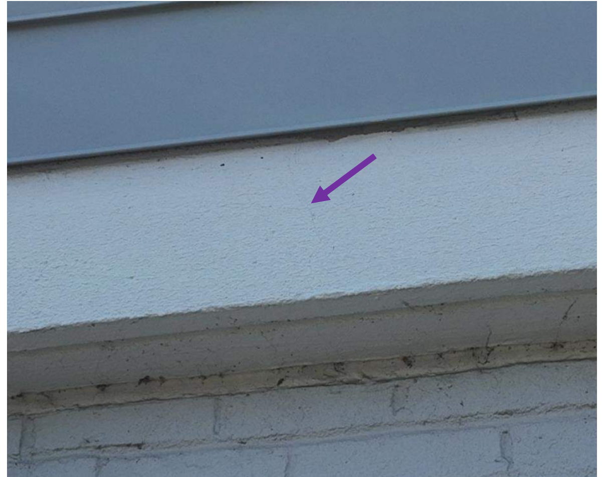
21 April 2025 Drone Survey, IMG 70
