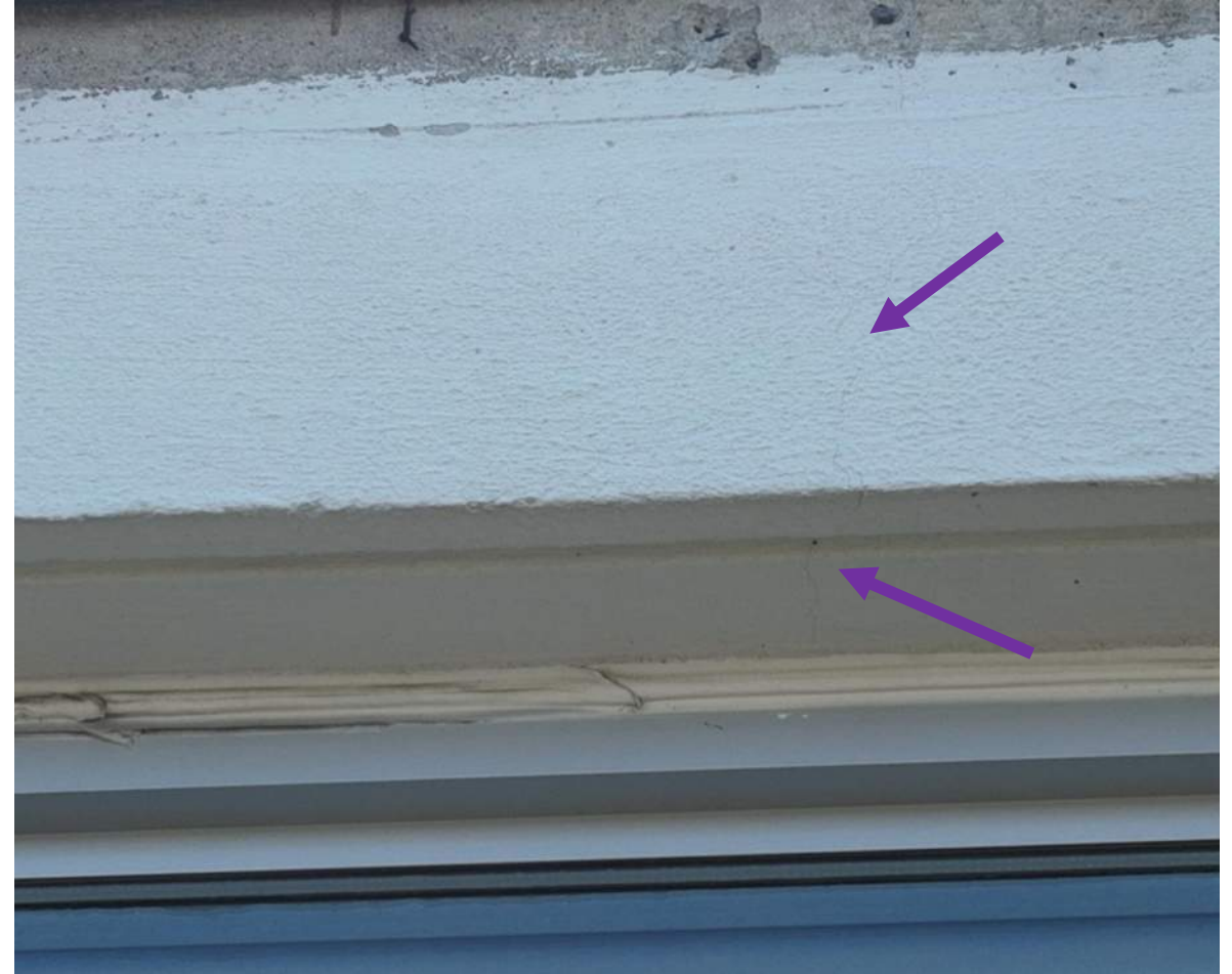
21 April 2025 Drone Survey, IMG#316
