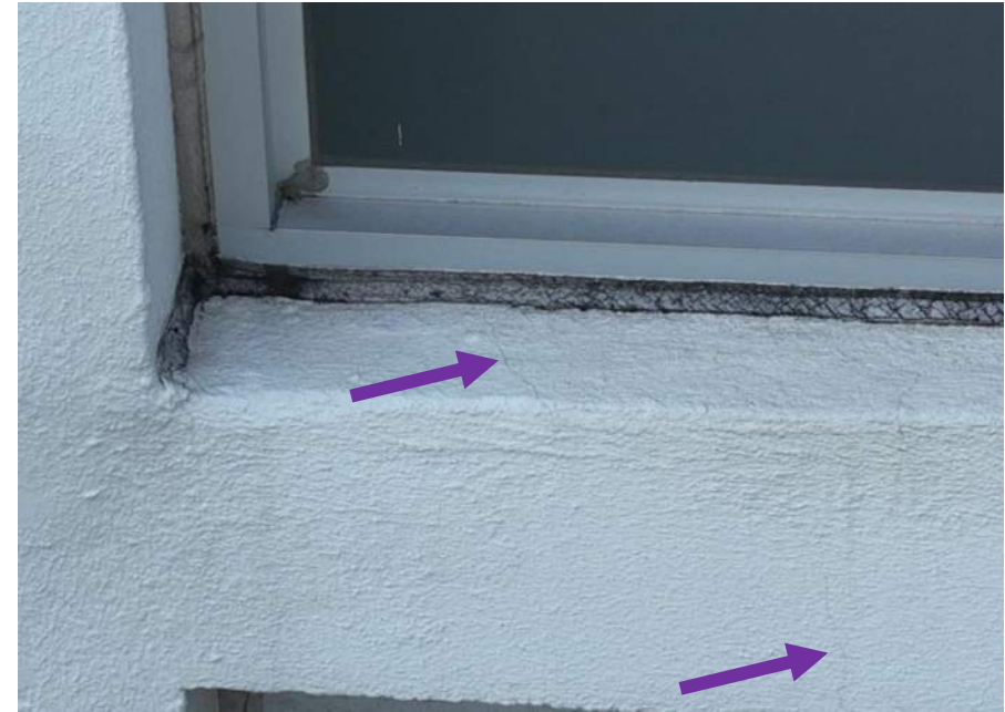
21 April 2025 Drone Survey, IMG#371
