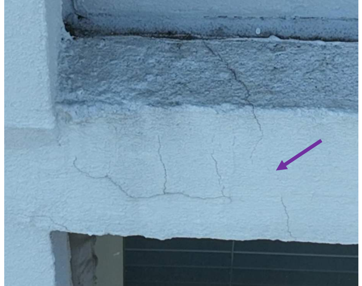
21 April 2025 Drone Survey, IMG#204
