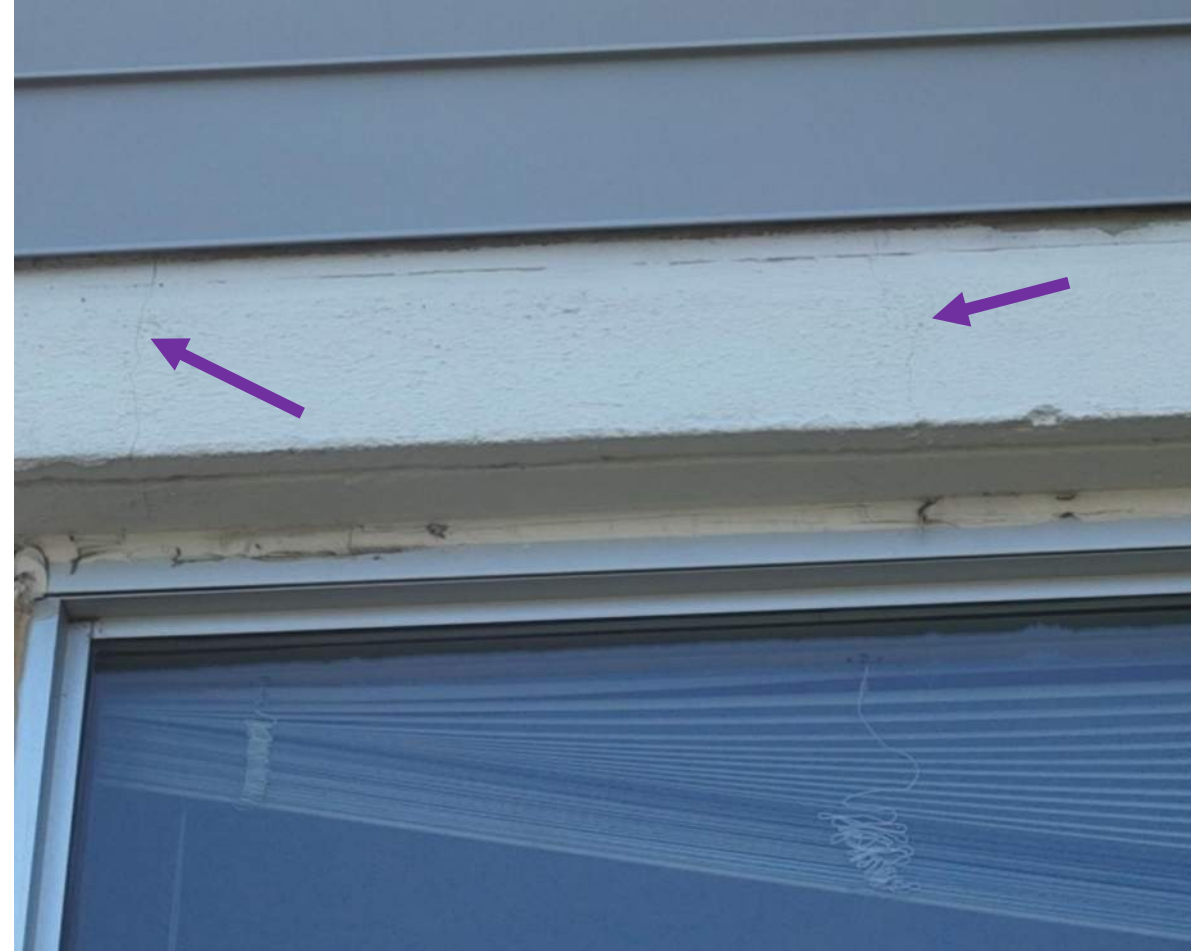
21 April 2025 Drone Survey, IMG#206
