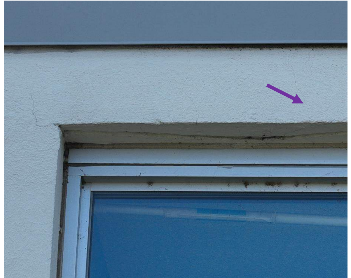
21 April 2025 Drone Survey, IMG 183
