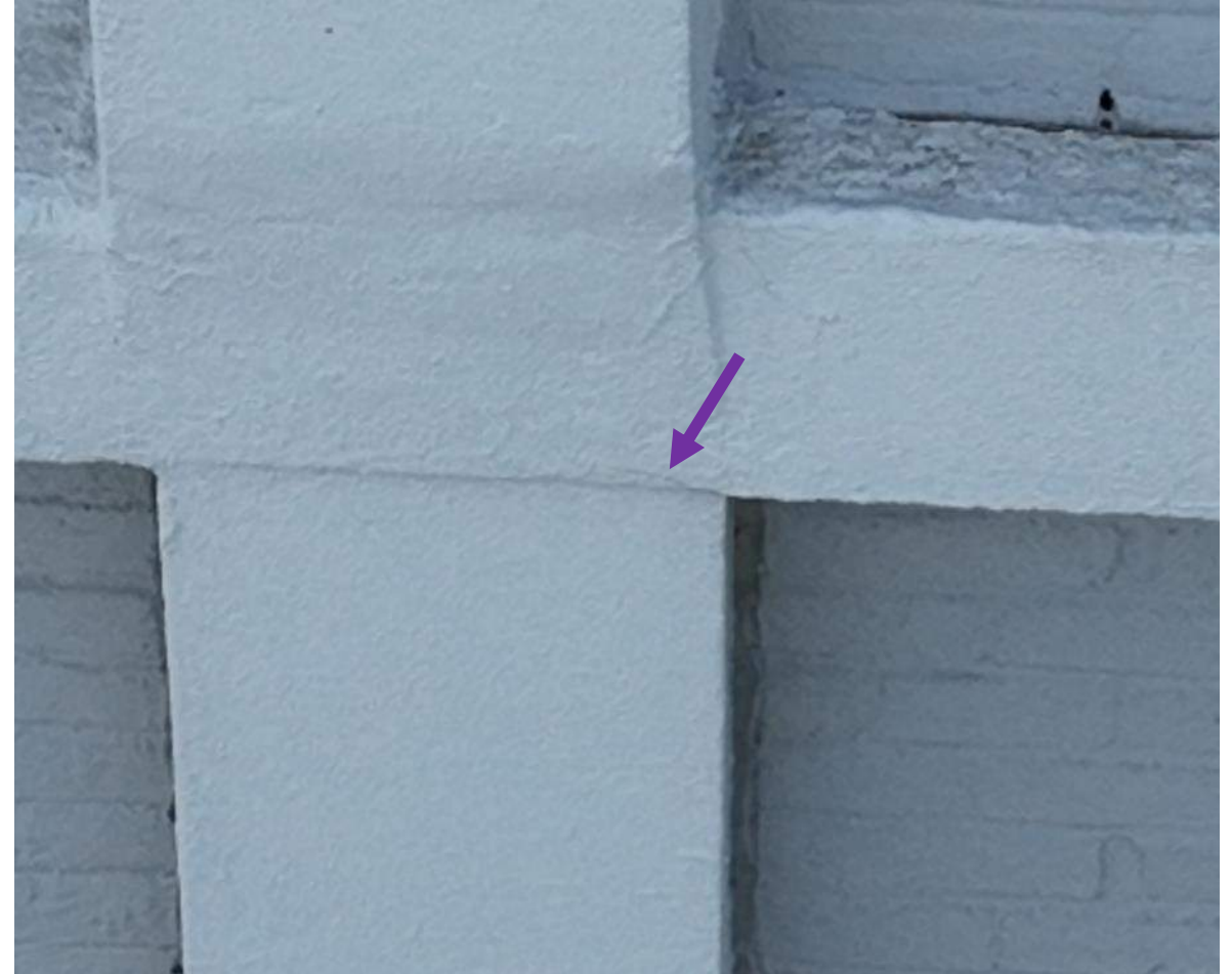
21 April 2025 Drone Survey, IMG 167
