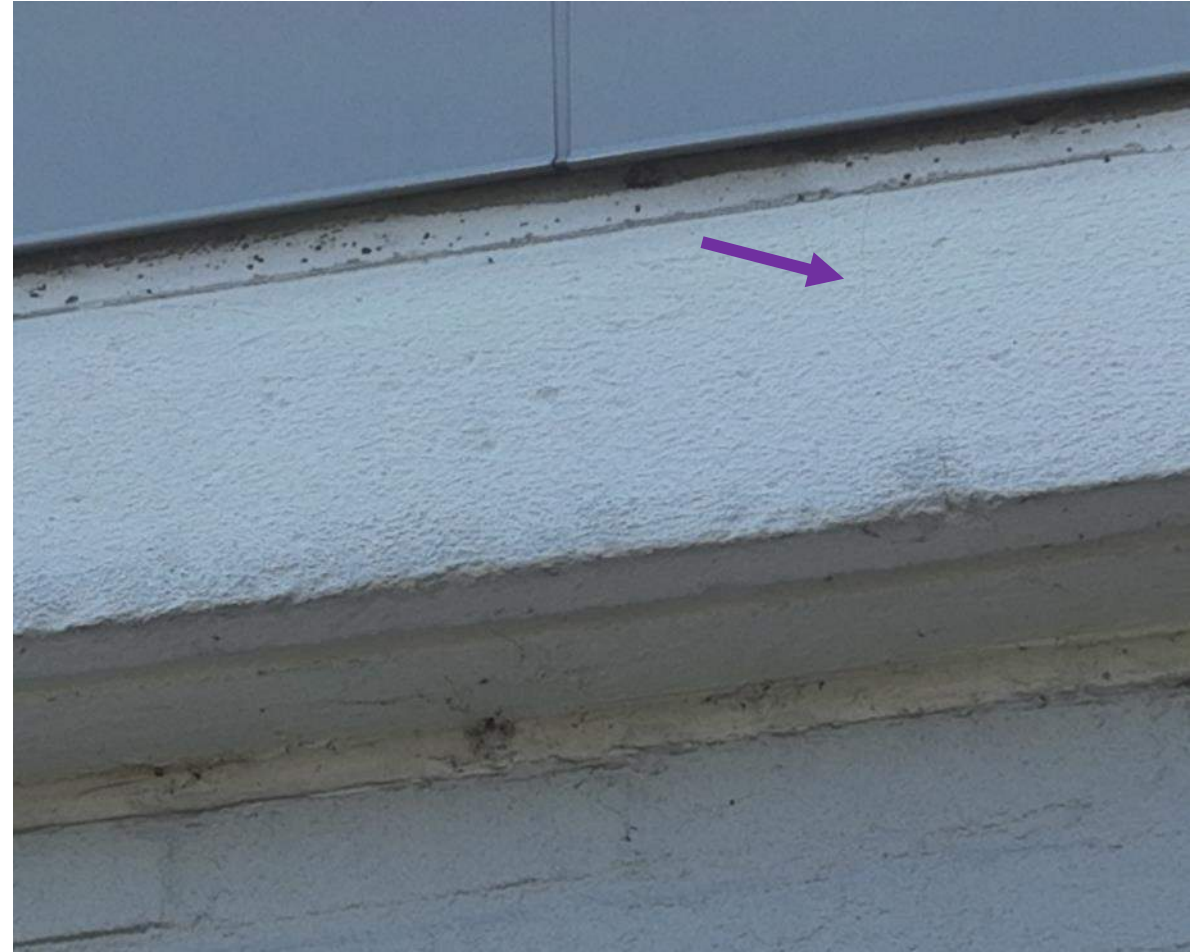
21 April 2025 Drone Survey, IMG 142
