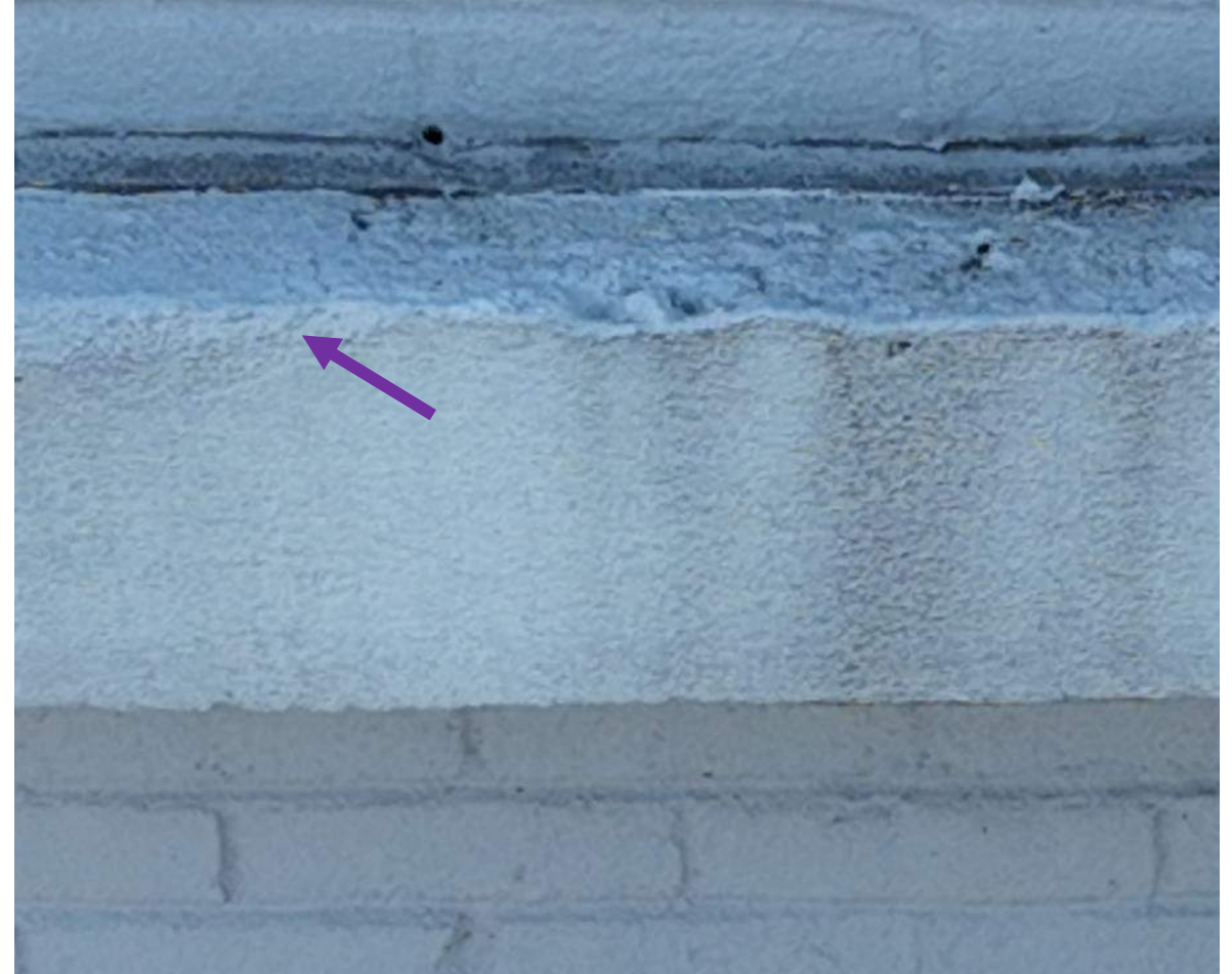
21 April 2025 Drone Survey, IMG 64
