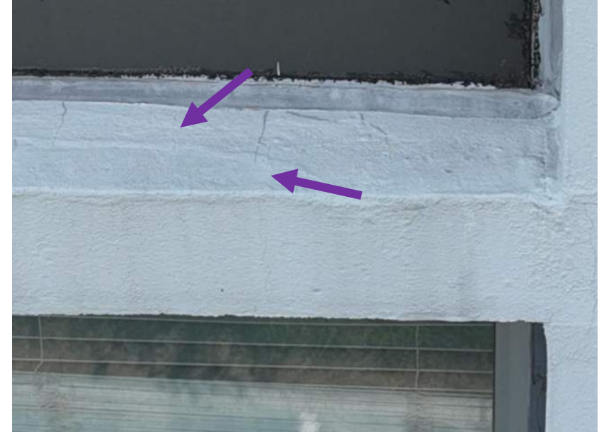
21 April 2025 Drone Survey, IMG#116
