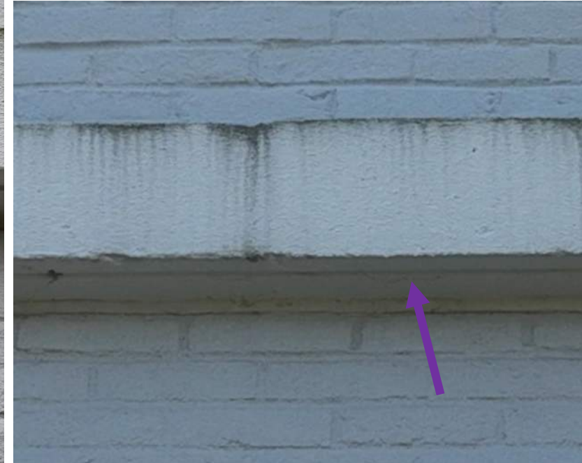
21 April 2025 Drone Survey, IMG#0398
