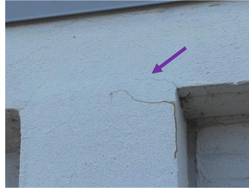
21 April 2025 Drone Survey, IMG#97
