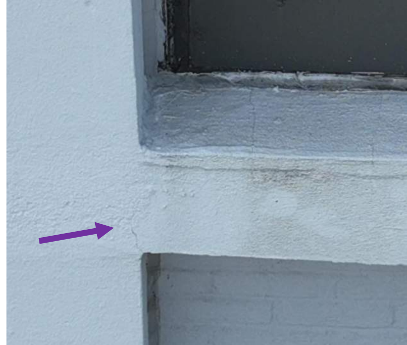
21 April 2025 Drone Survey, IMG#147
