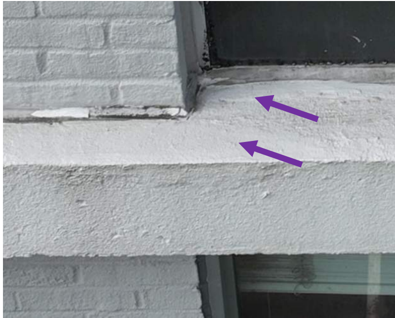
18 June 2024 Drone Survey, IMG#2-029
