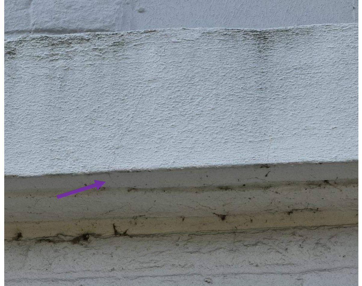
21 April 2025 Drone Survey, IMG 682
