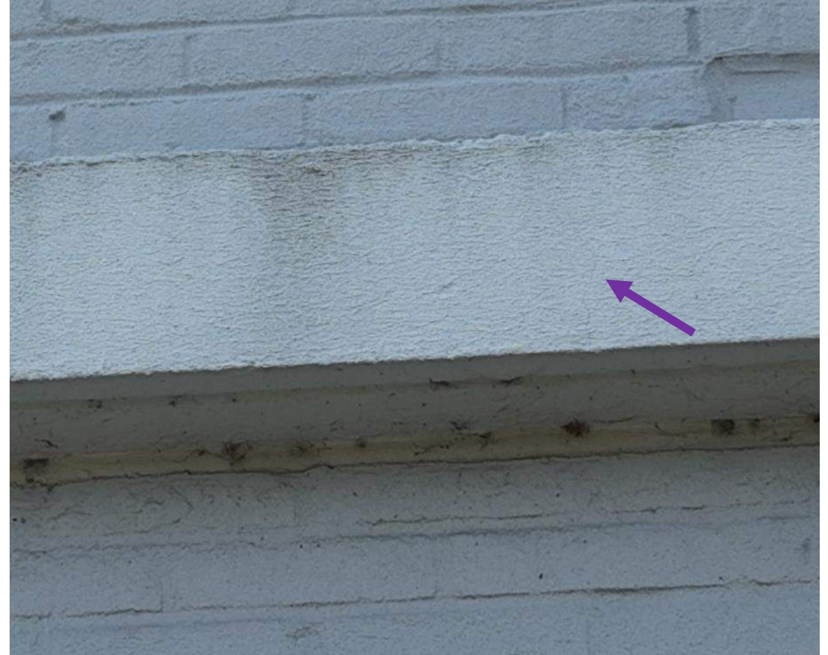
21 April 2025 Drone Survey, IMG 0511
