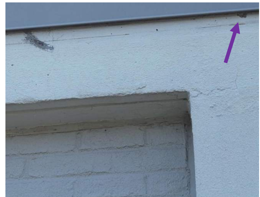
21 April 2025 Drone Survey, IMG#261
