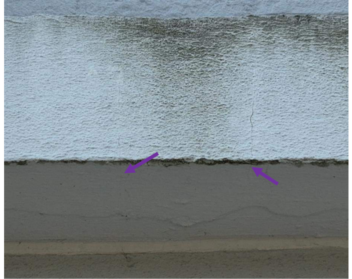
21 April 2025 Drone Survey, IMG 258
