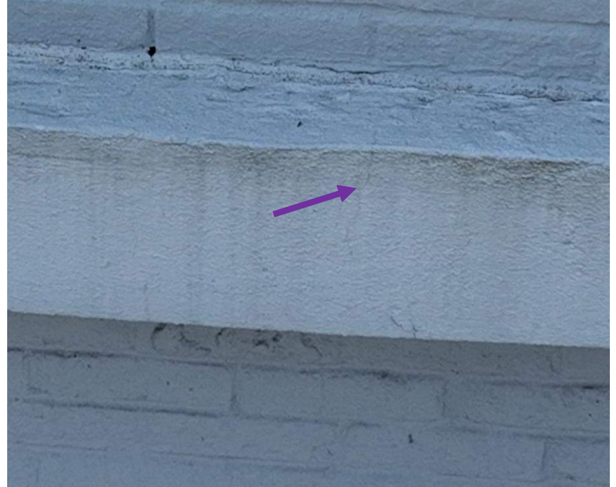
21 April 2025 Drone Survey, IMG 269
