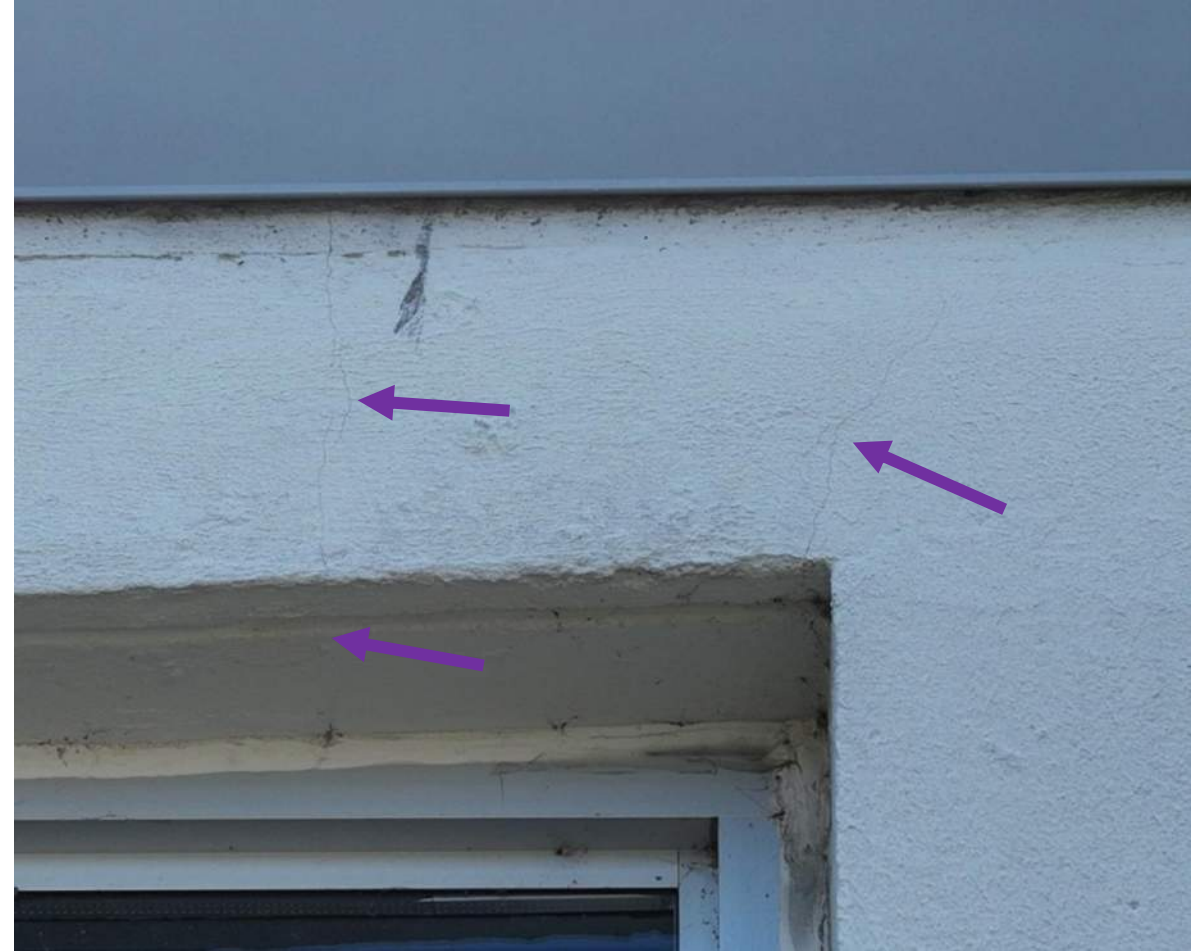
21 April 2025 Drone Survey, IMG#300
