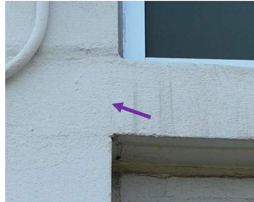
21 April 2025 Drone Survey, IMG#493
