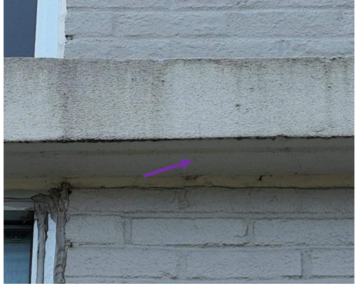
21 April 2025 Drone Survey, IMG 310
