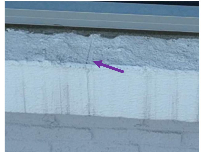
21 April 2025 Drone Survey, IMG#184
