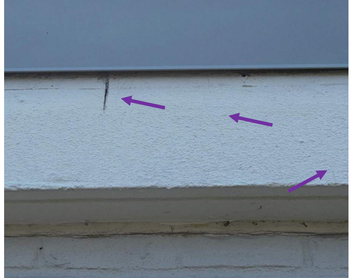
21 April 2025 Drone Survey, IMG#303
