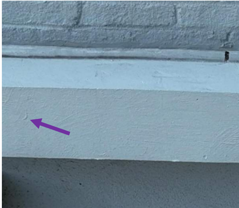
18 June Drone Survey, IMG#3-011
