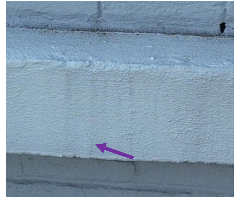
21 April 2025 Drone Survey, IMG#150
