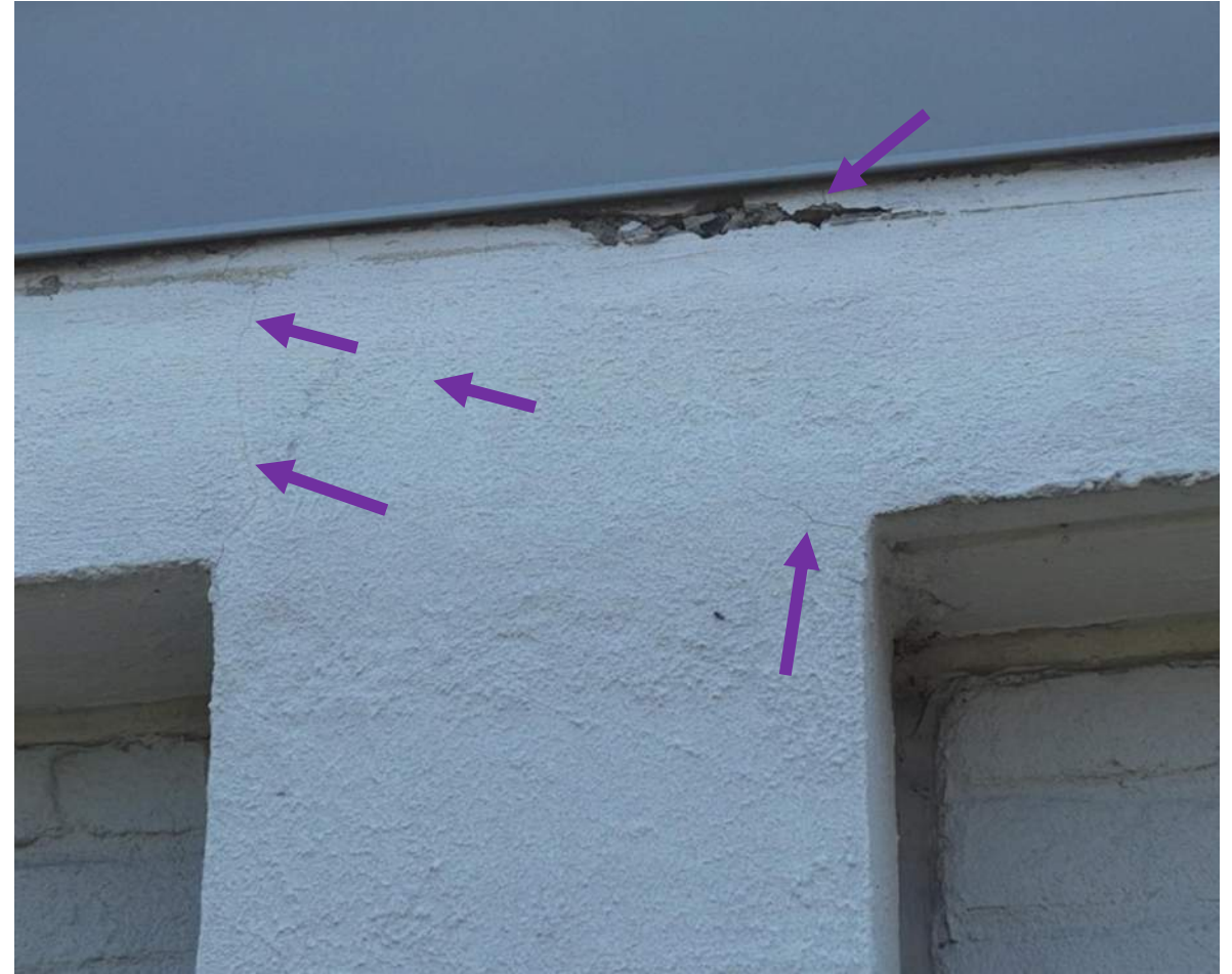
21 April 2025 Drone Survey, IMG#281
