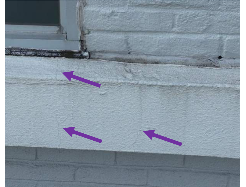
21 April 2025 Drone Survey, IMG#376
