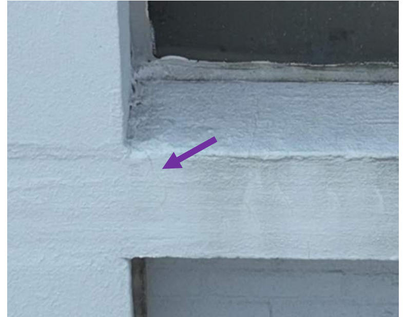
21 April 2025 Drone Survey, IMG#46
