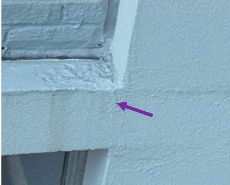
18 June Drone Survey, IMG#3-080
