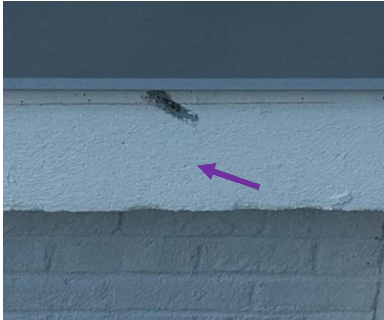
18 June Drone Survey, IMG#3-001
