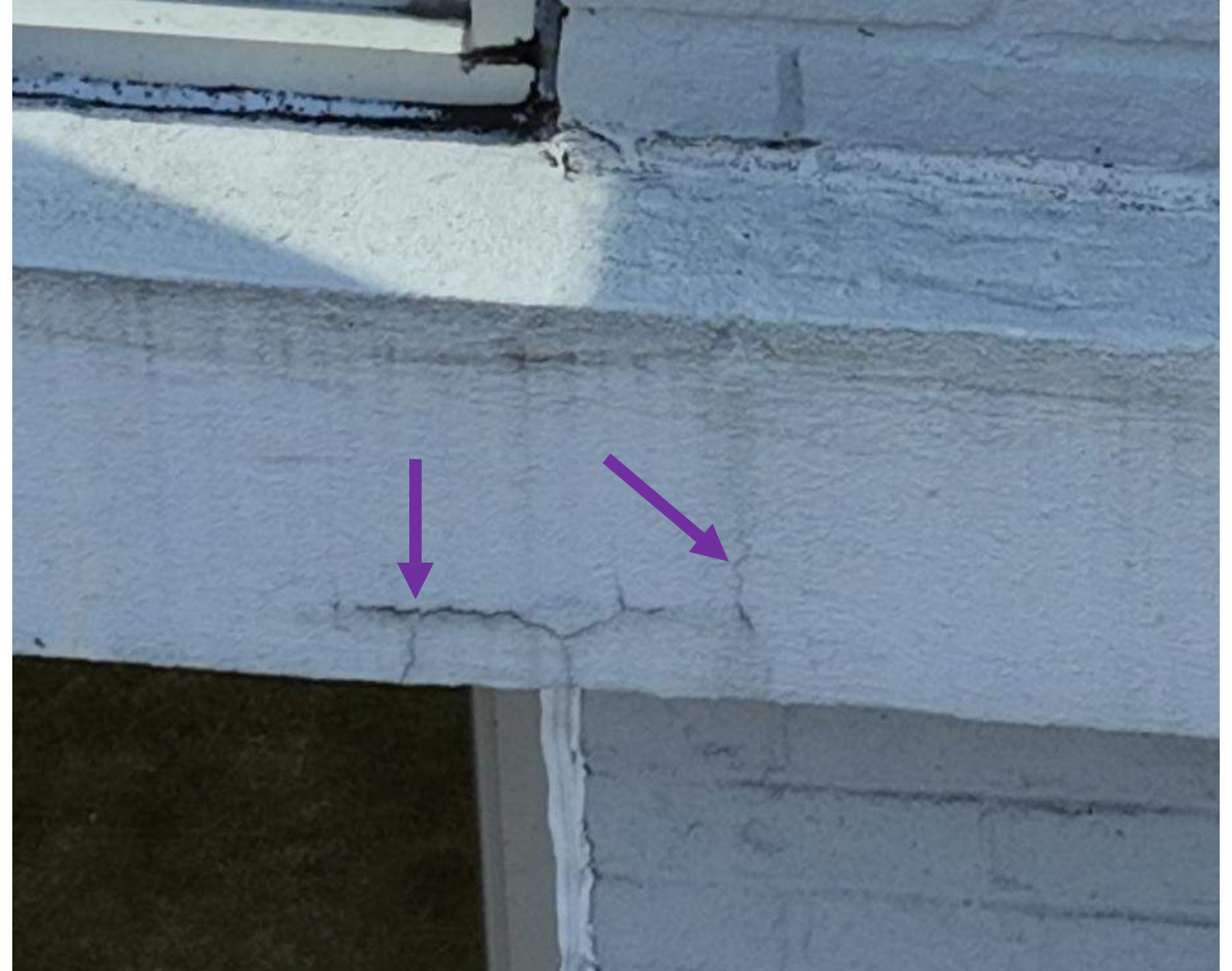
21 April 2025 Drone Survey, IMG 269
