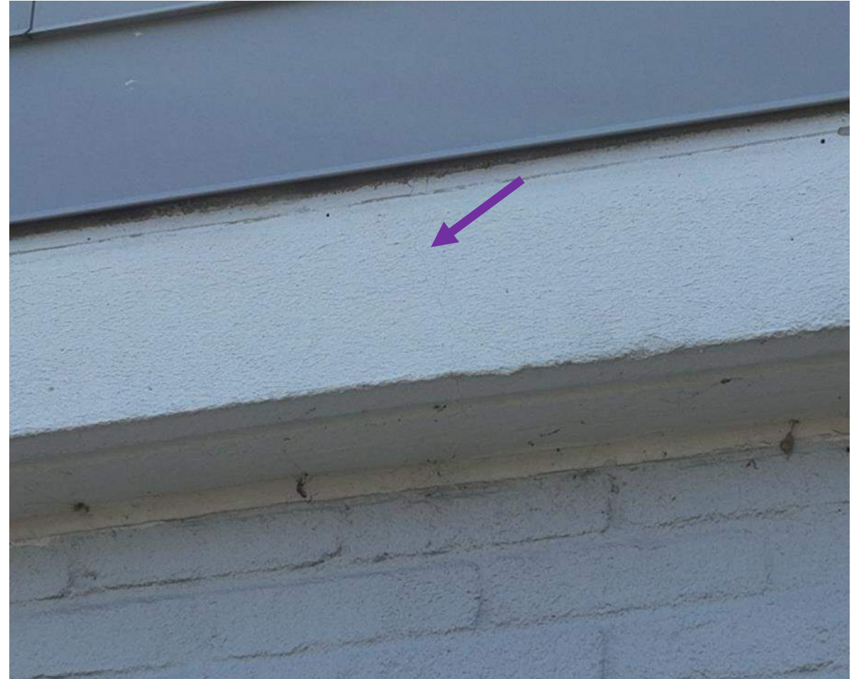
21 April 2025 Drone Survey, IMG 150
