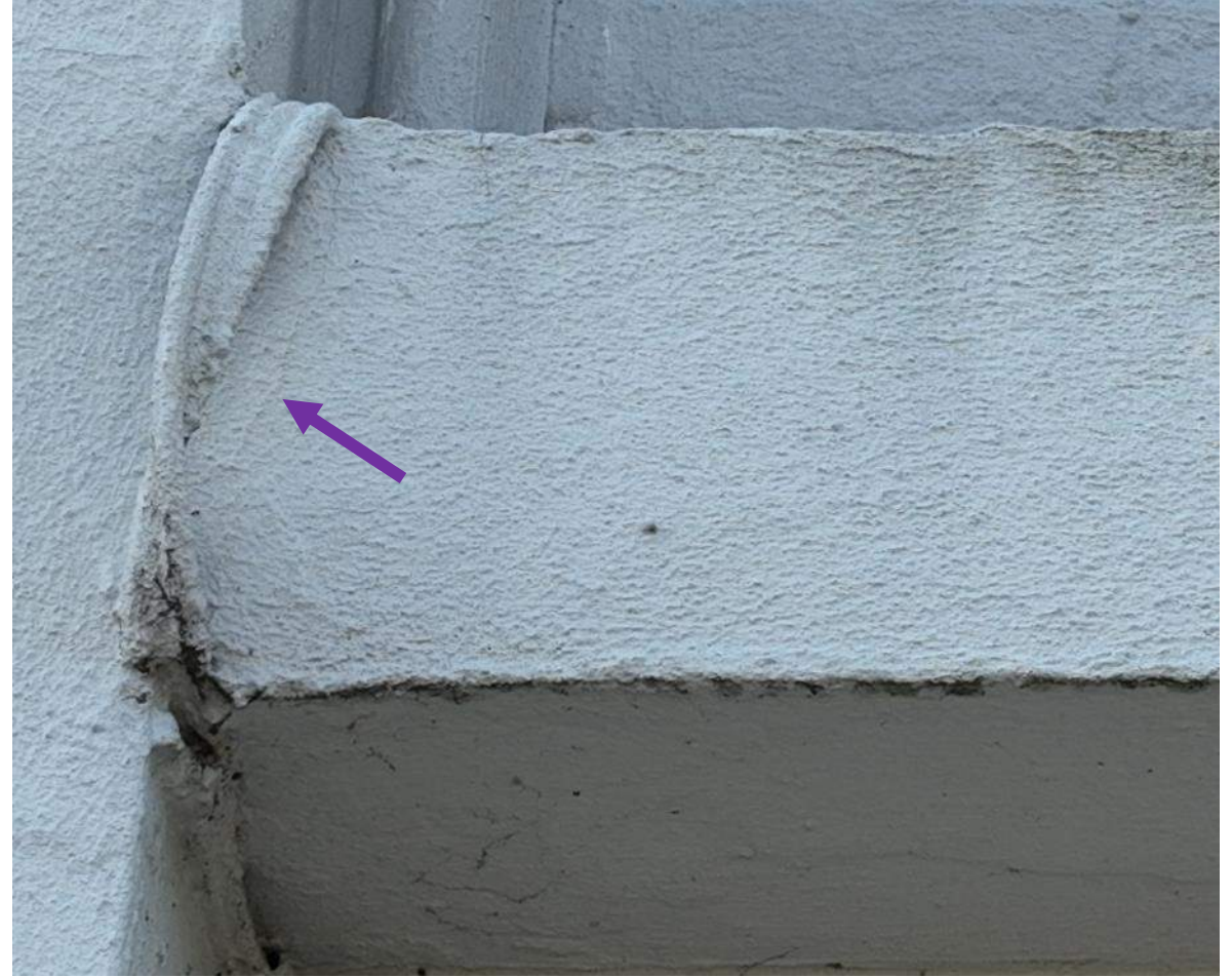
21 April 2025 Drone Survey, IMG 254
