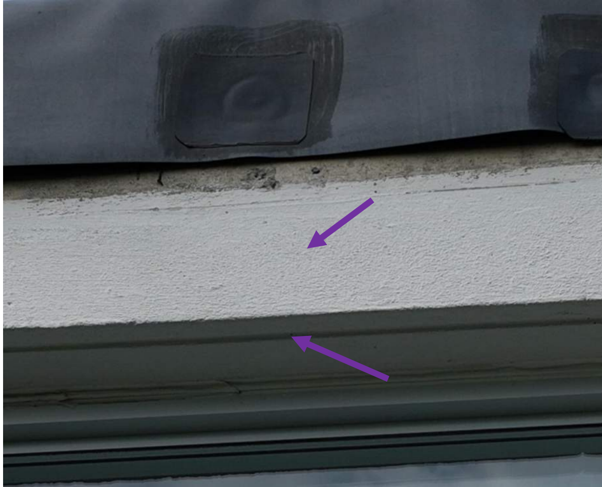
18 June 2024 Drone Survey, IMG#132
