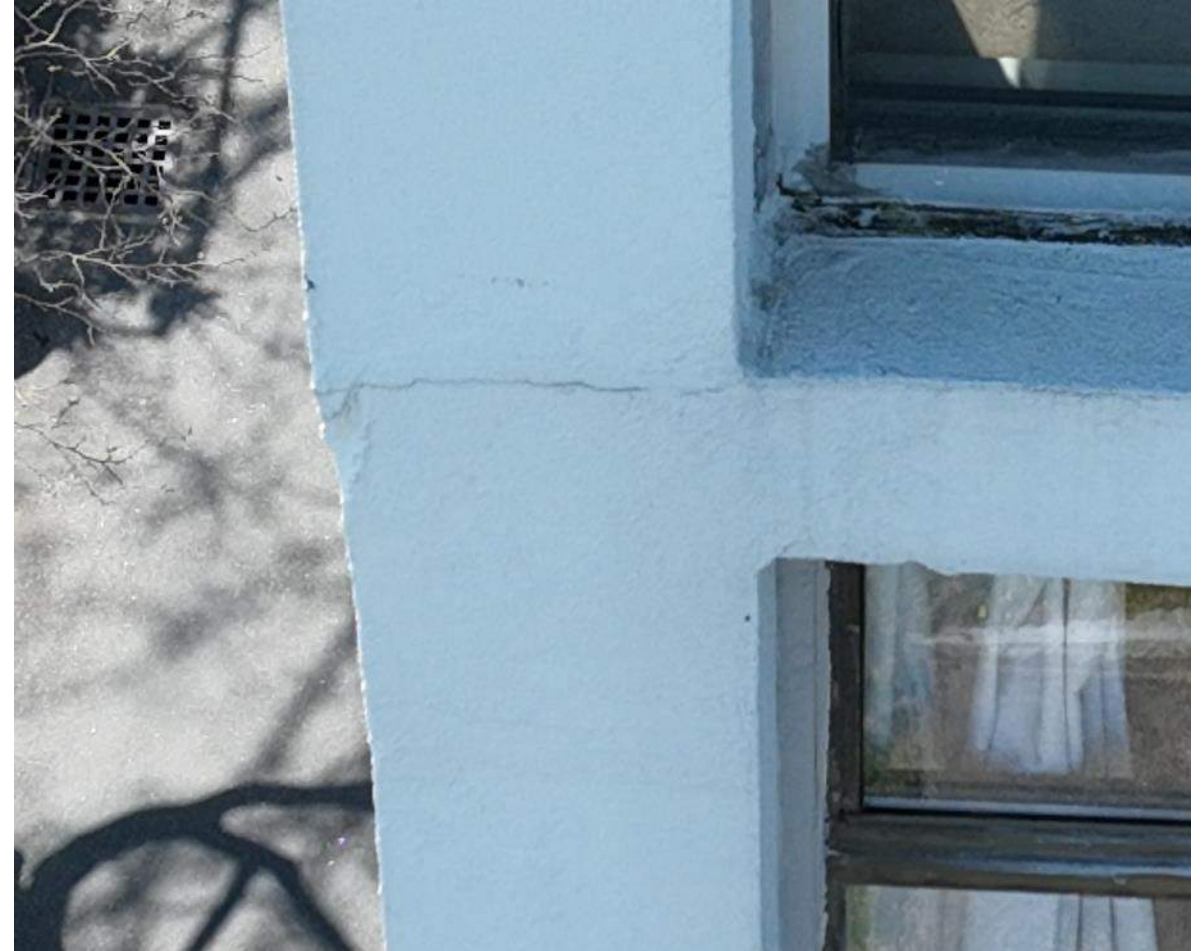
21 April 2025 Drone Survey, IMG 776
