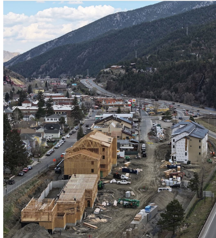
Fieldhouse Apartments, Idaho Springs, CO. Source: Developing Colorado
