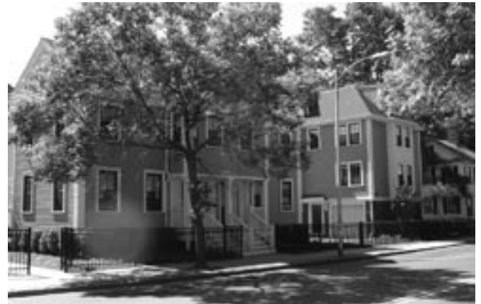
Just A Start completed construction at Scouting Way, creating 13 affordable family-sized rental units adjacent to Sennott Park.
