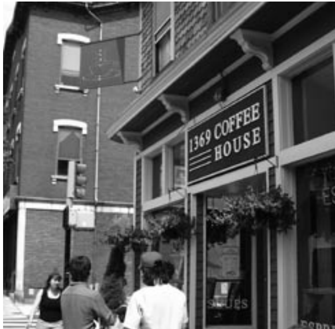
Storefront improvements at 1369 Cambridge Street were completed this year as part of the City's Façade Improvement Program.
