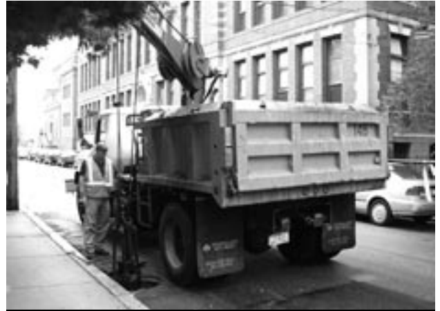
Catch basins are cleaned annually as part of the City's stormwater management program.
