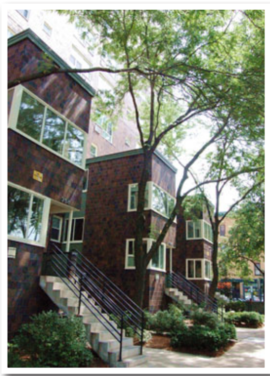
Inman Square Apartments (116 affordable rental units, preserved and renovated by HRI)
