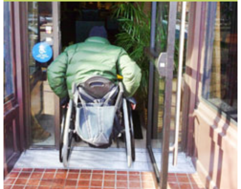
Giulia Restaurant, 1682 Mass. Ave., replaced existing uneven threshold transition with a simple metal threshold and automatic door opener.
