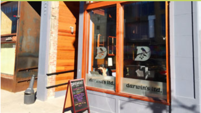
Darwin's, LTD, 313 Mass. Ave., replaced inaccessible storefront that included a 4 inch step with a new recessed entrance, smooth ramp, and automatic door opener.
