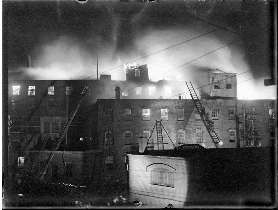
Four alarm fire at Hew's and Co.'s old pottery plant, North Cambridge, causing $500,000 damage. It's believed that this fire took place on the evening of August 14, 1930. )
