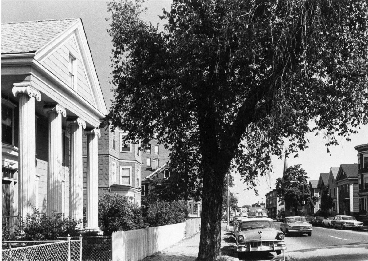
Western Avenue looking east, 1970. (#135 at far left)
