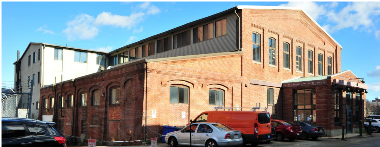
101 Rogers Street, west and south elevation
