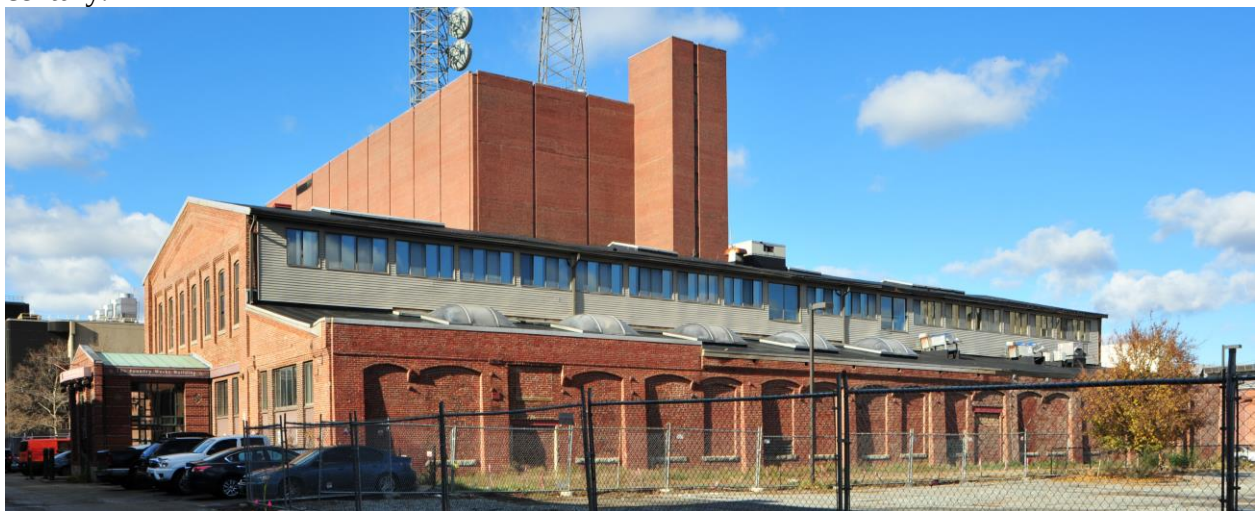
101 Rogers Street, east elevation
