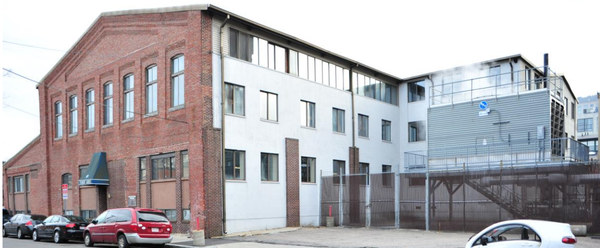
101 Rogers Street, north and west elevation. A portion of the original structure was removed and the property sold to the abutter to accommodate the cooling tower.
