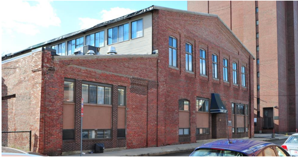
101 Rogers Street, north elevation
