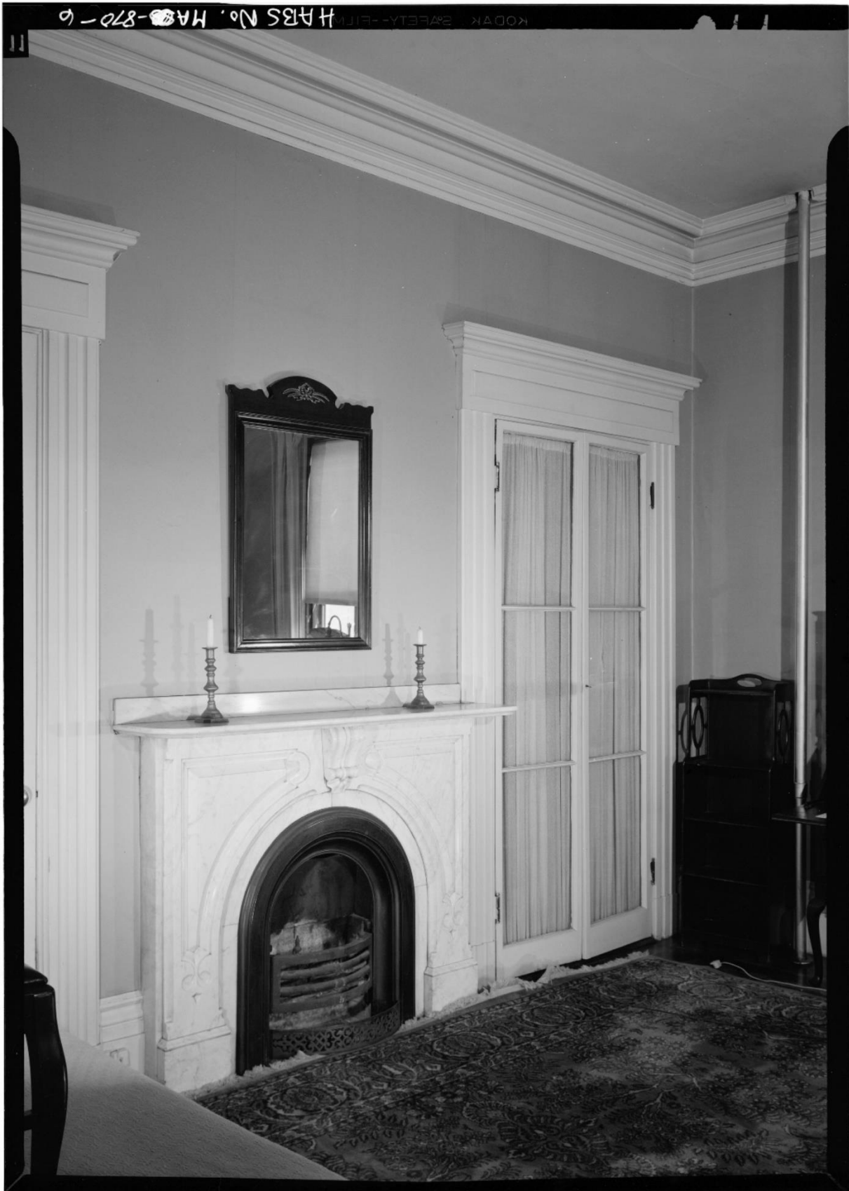
South parlor, detail of fireplace wall. HABS photo, 1964.
