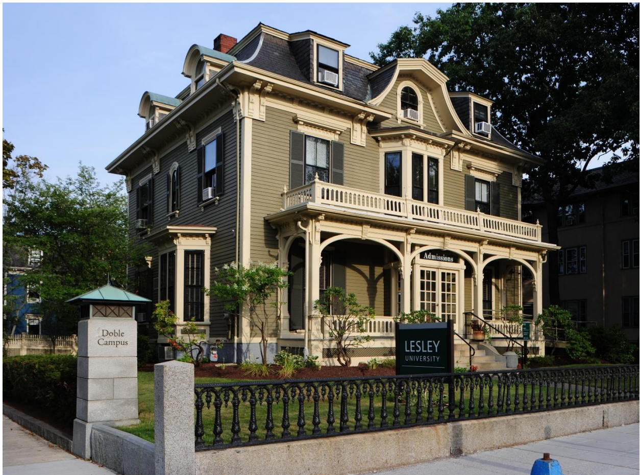
1627 Massachusetts Avenue. CHC photo, 2009.
