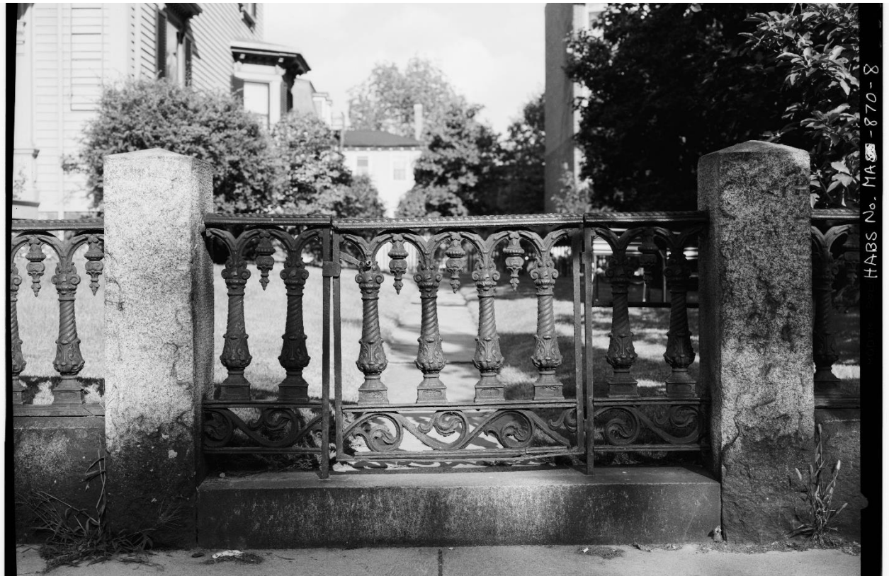
Cast iron fence and gate at Massachusetts Avenue. HABS photo, 1964.
