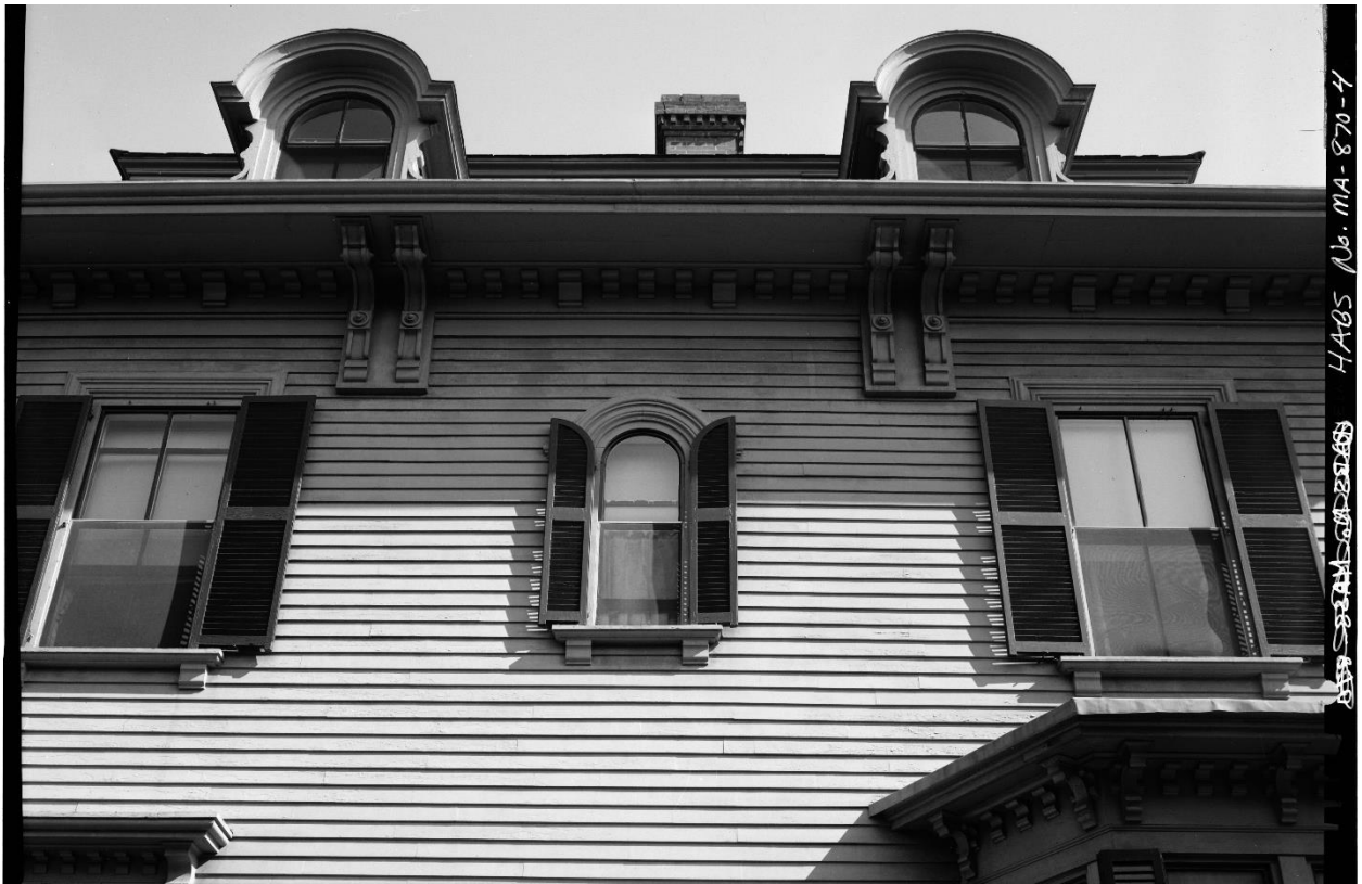
Detail of cornice and dormers. HABS photo, 1964.
