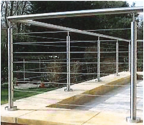
Stainless steel cable railing on retaining wall
