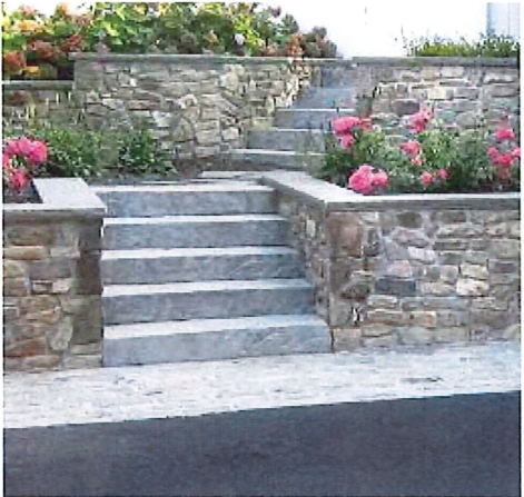
Stone veneer retaining wall with bluestone capstone, granite steps
