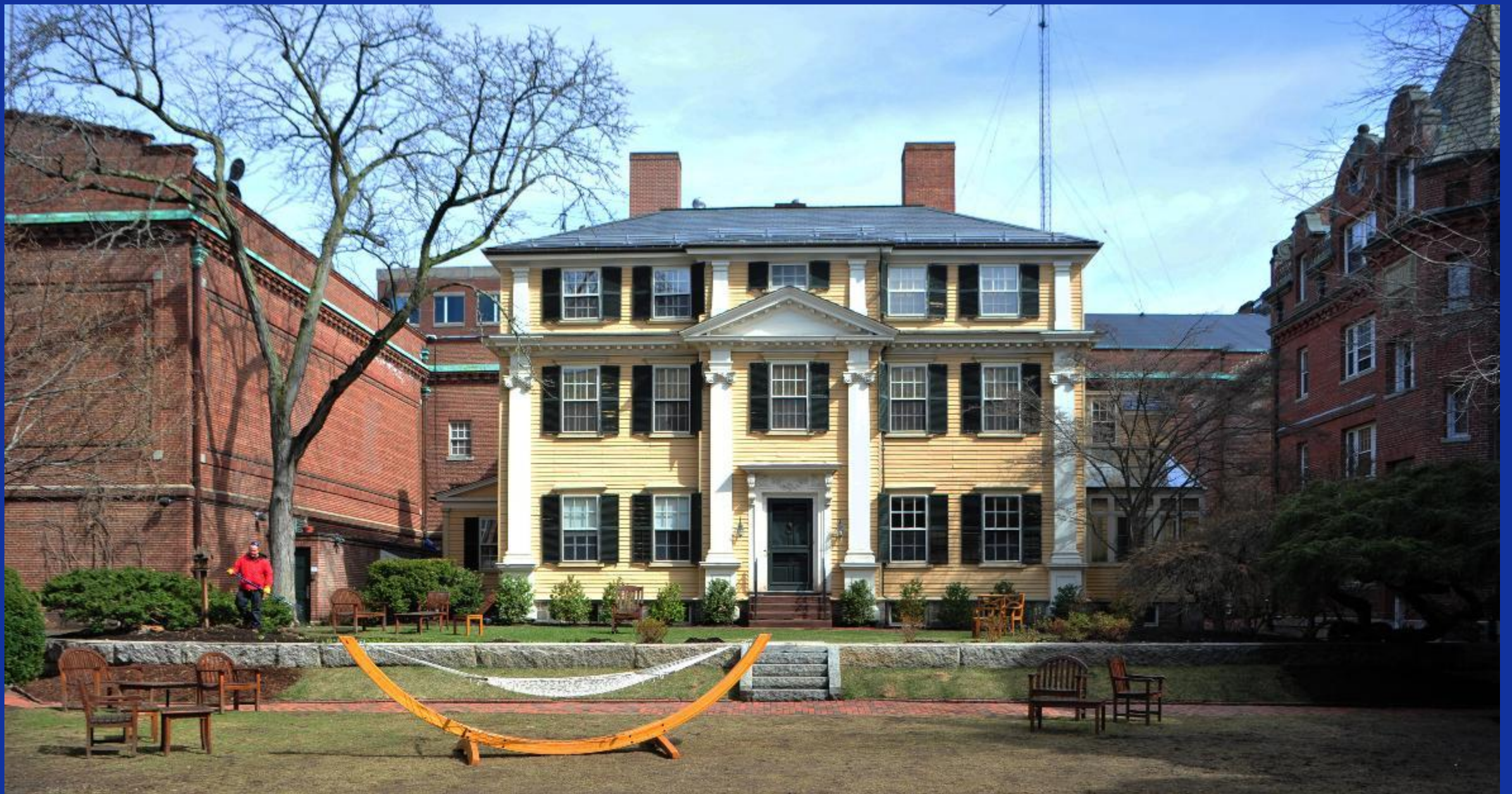
Apthorp House (1760, Peter Harrison, probable designer) Under construction 2019-2021
