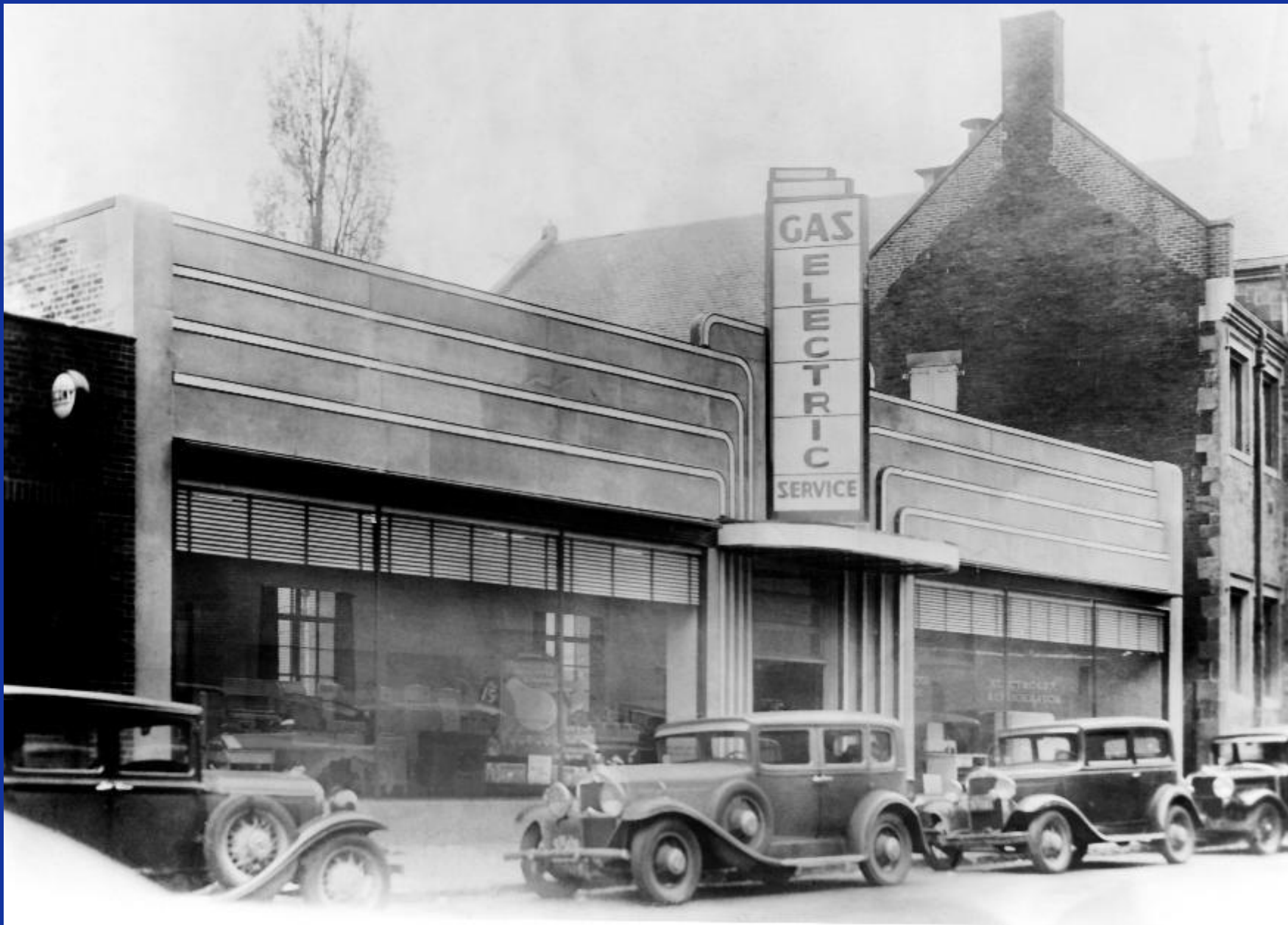
Cambridge Electric Light Co. store, 23-25 Church Street (1936, William L. Galvin, architect
