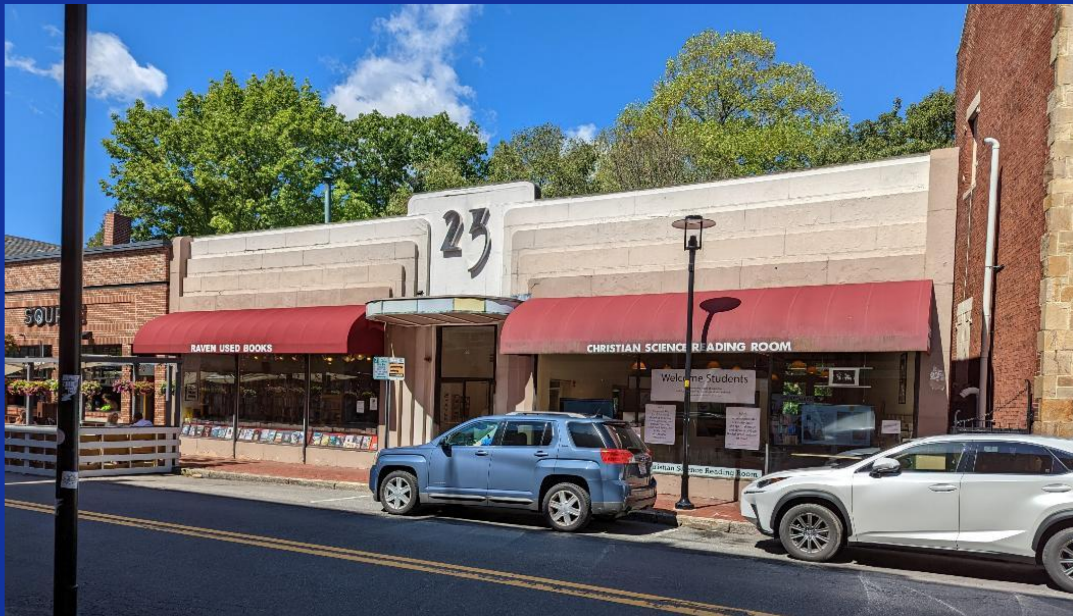
23 Church Street as renovated and painted in 1986
