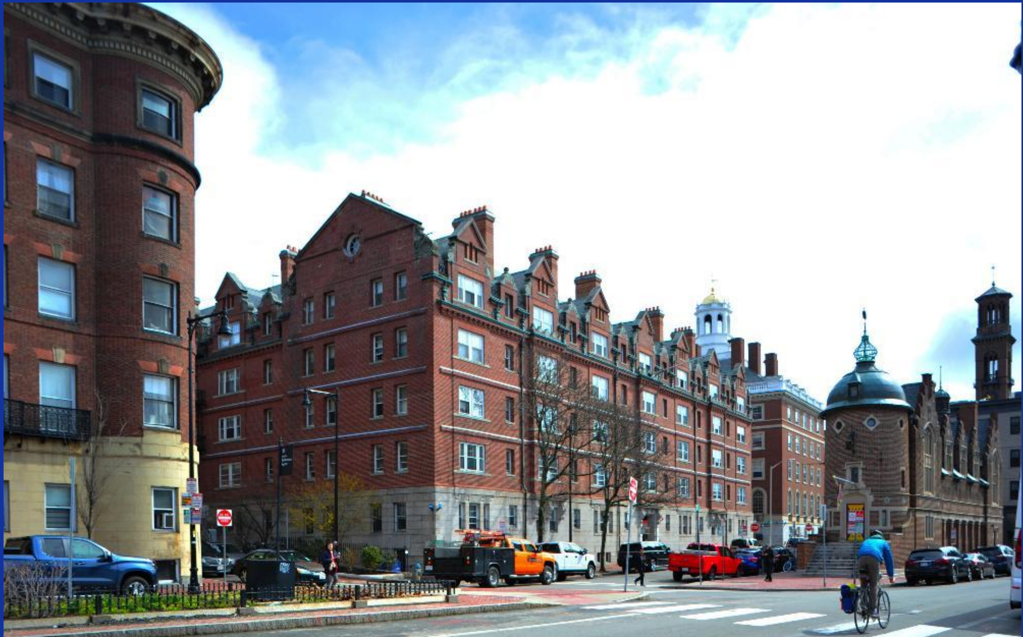
Randolph Hall (1897, Coolidge & Carlson, architects) Under construction 2021-2023
