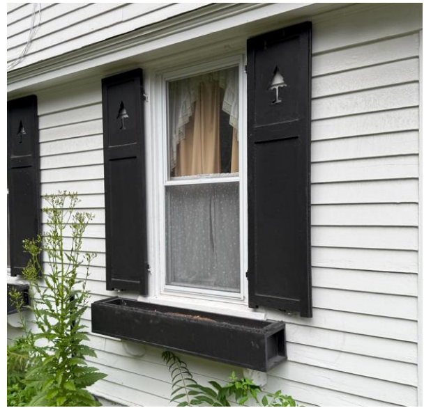
Typical window detail, original shutters and flower box
