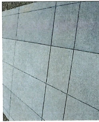
Concrete Paving SRI 35
