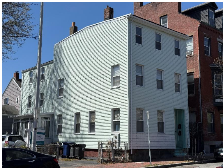
78 Otis Street façade and east side elevation, April 2026.
