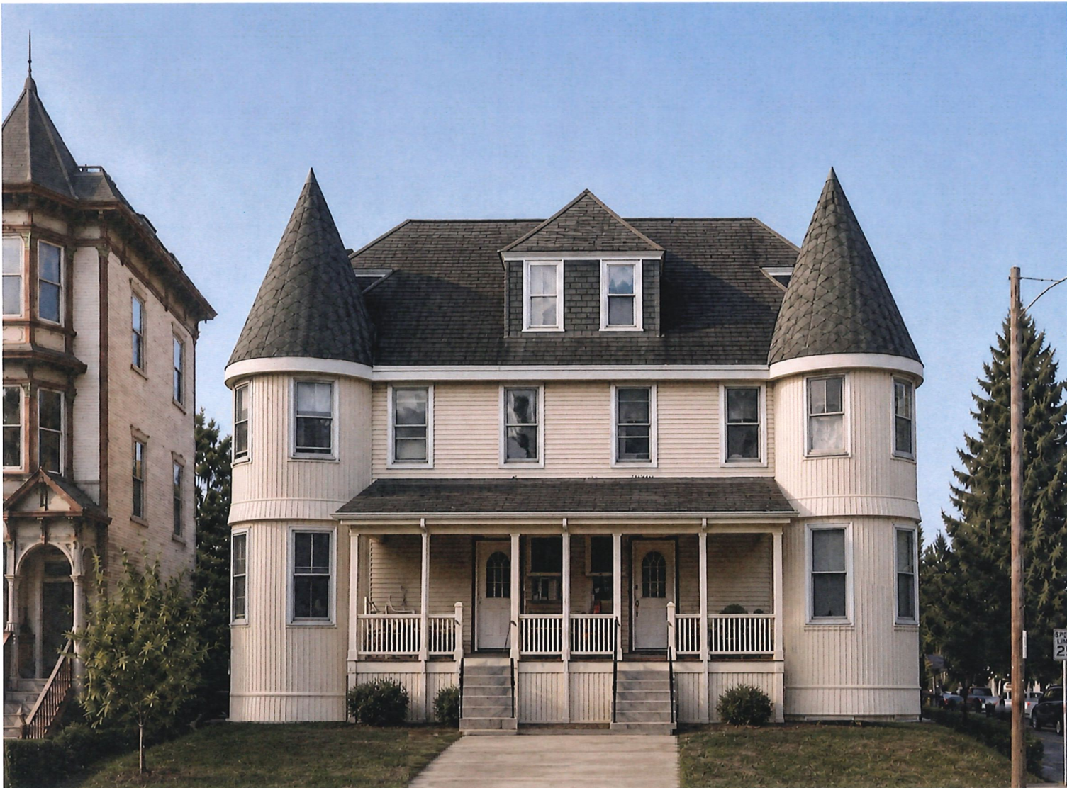
EXISTING CONDITION - SITE WITH CONTEXT
