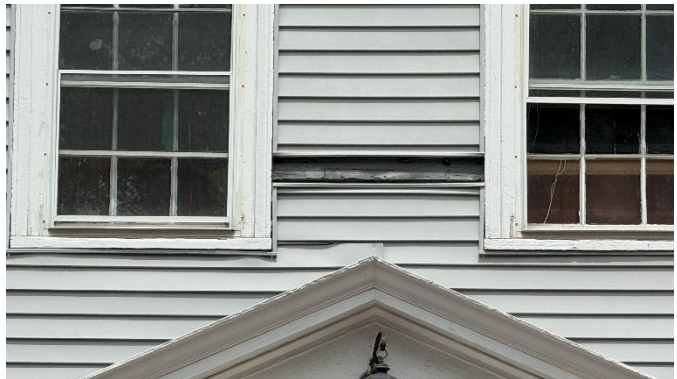
Wooden clapboard exposed from break in overlaying siding.
