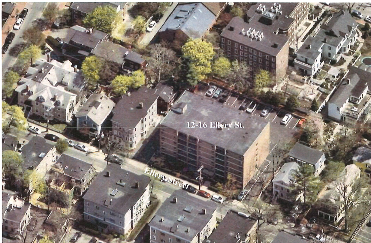
Ellery Street toward Mass Ave (to the right) -12-16 Ellery Street constructed in 1973
