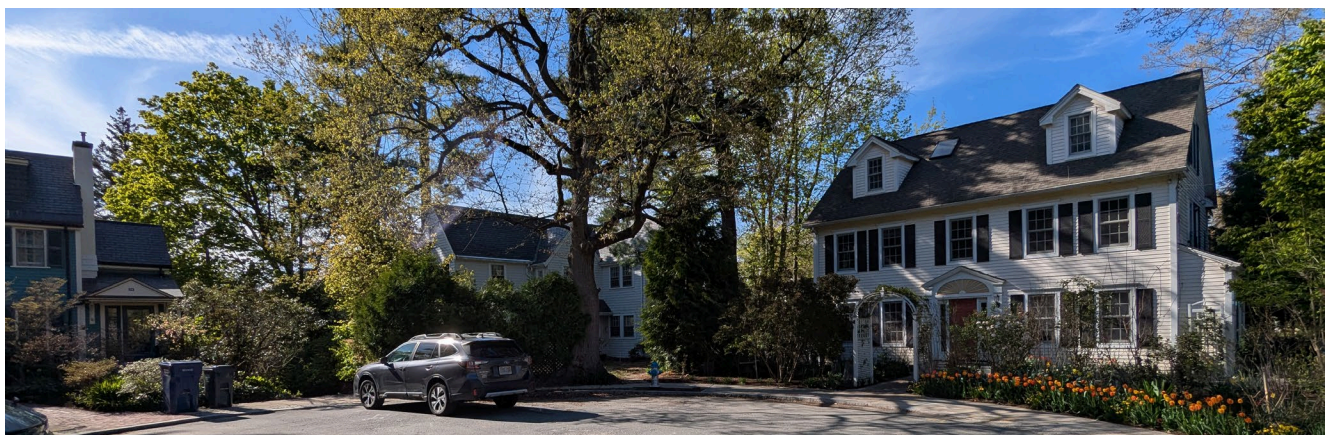
R-L: 5 Wyman Road (1926), 9 Wyman Road (1927) and 14 Wyman Road (1927), all by Duguid & Martin CHC 2026
