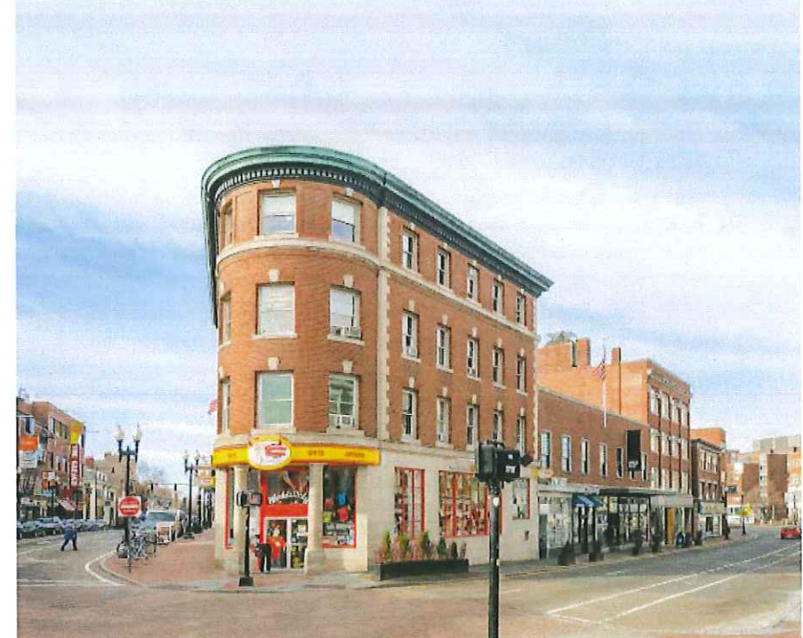
VIEW FROM BRATTLE STREET
