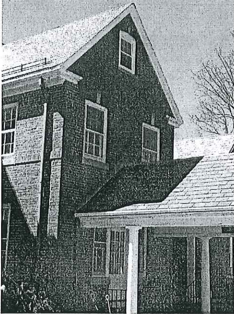
View of Center facade opposite Meeting House.
