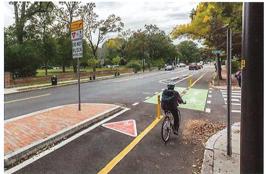
Photo: Crossing island at Lexington Avenue intersection.
