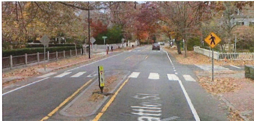
Photo: Former flush crossing island, which does not protect people from traffic
