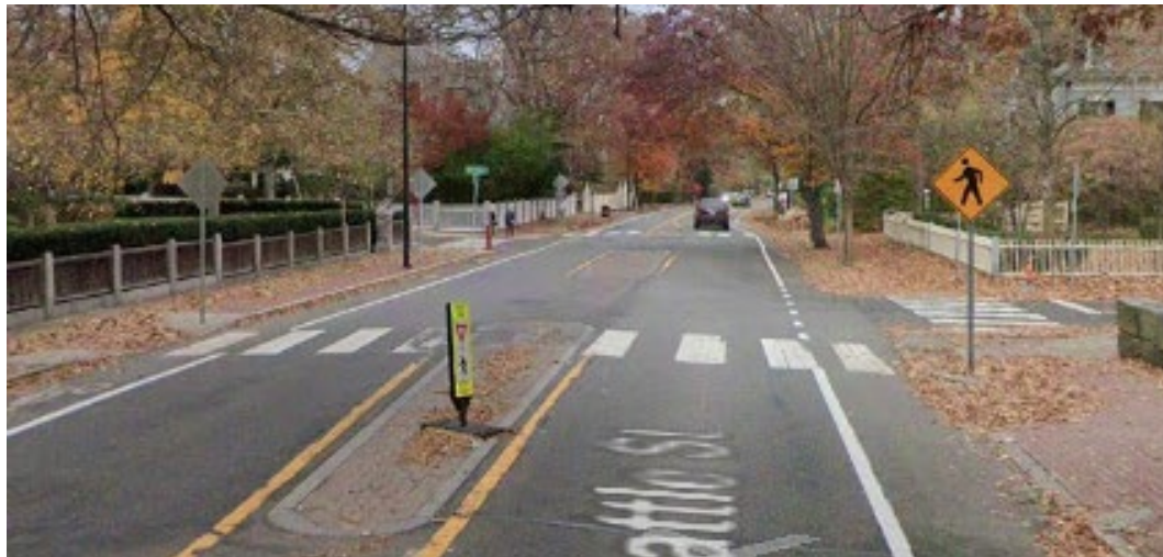
Photo: Former flush crossing island, which does not protect people from traffic
