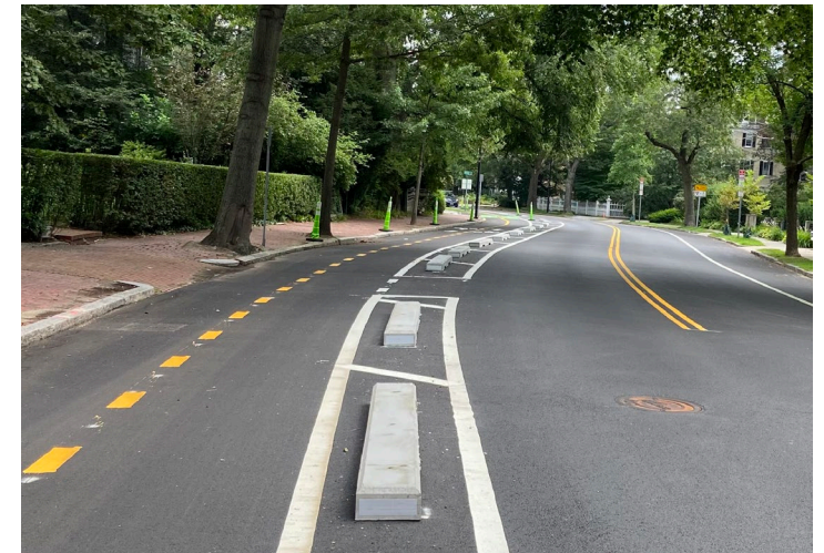
A section of precast curbing on Brattle Street on installation day. (2023)
