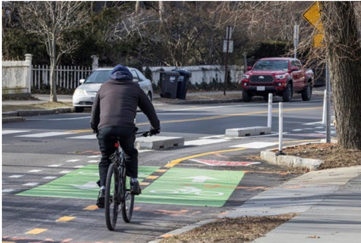
Photo: Curb Extension at Willard Street reduced
