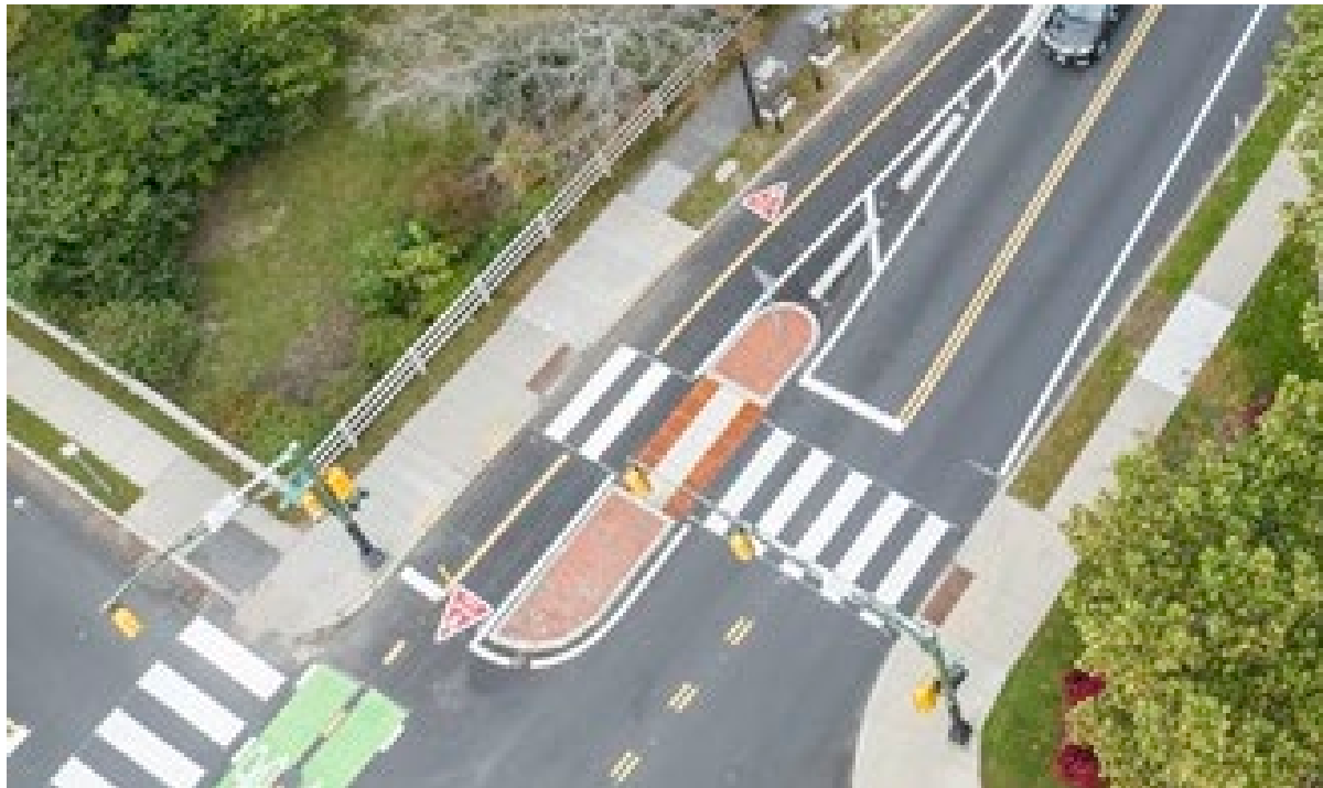
Photo: Crossing island at Fayerweather Street intersection.
