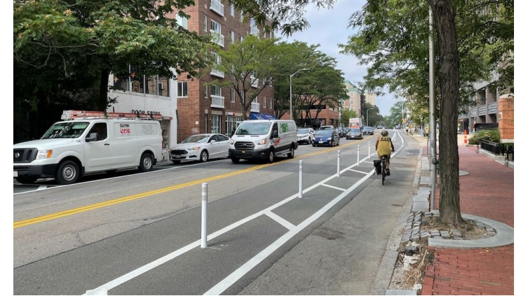
A separated bike lane on Mass Ave near Central Square. (2021)
