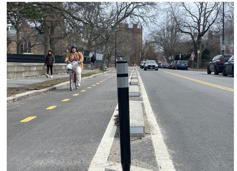
Example: Black flexible delineator posts are an option instead of white if they still have white reflective tape.
