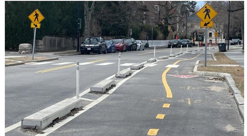
Extra posts installed (every 20ft) near Longfellow Park where the lane curves around a curb extension. (2024)
