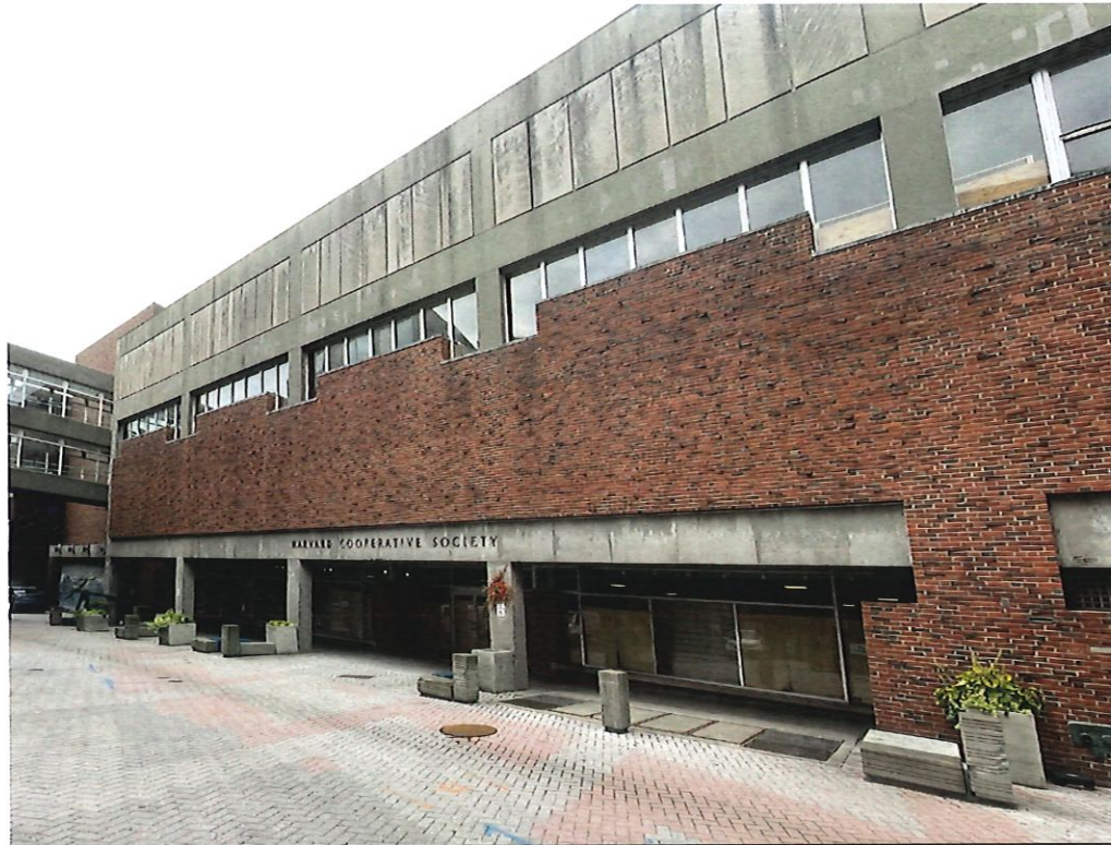
Existing Conditions - Exterior
