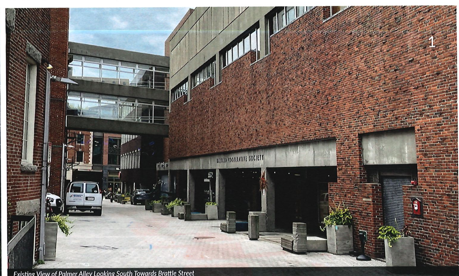
Existing View of Palmer Alley Looking South Towards Brattle Street
