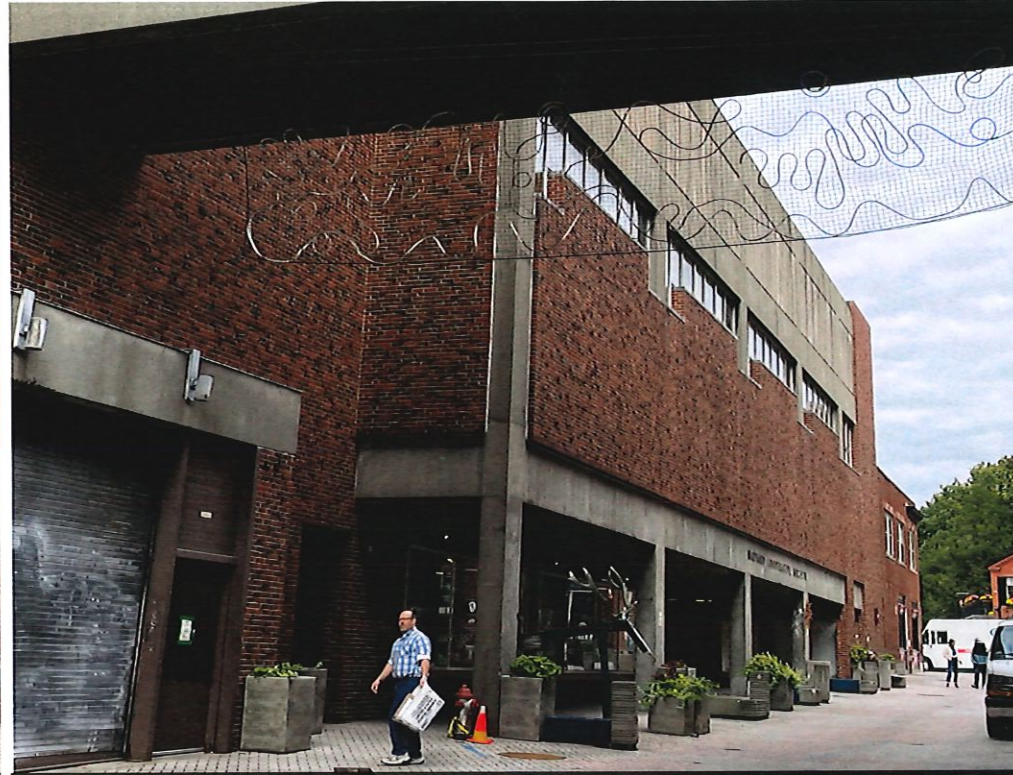
Existing Conditions - Exterior
