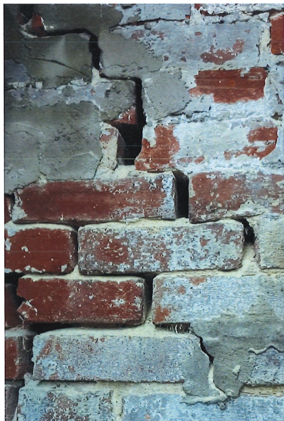
DETERIORATED MASONRY AT FOUNDATION WALL
