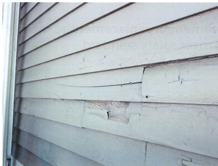
DETERIORATED SIDINGS, BUILDING PAPER, ROOF SHINGLES, AND CEILING
