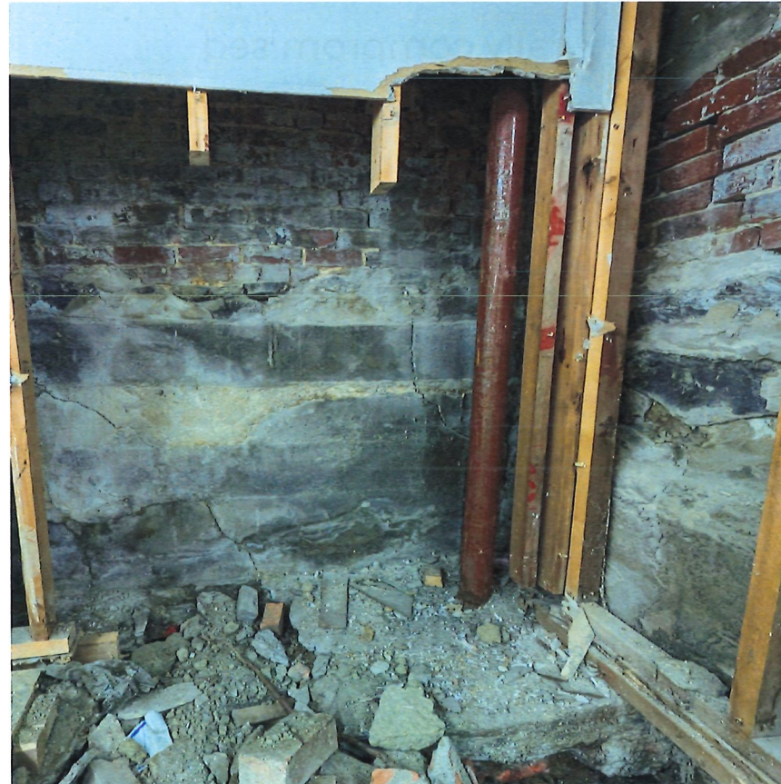
PREVIOUS UNDERPINNING/ REPAIR AT SE CORNER
