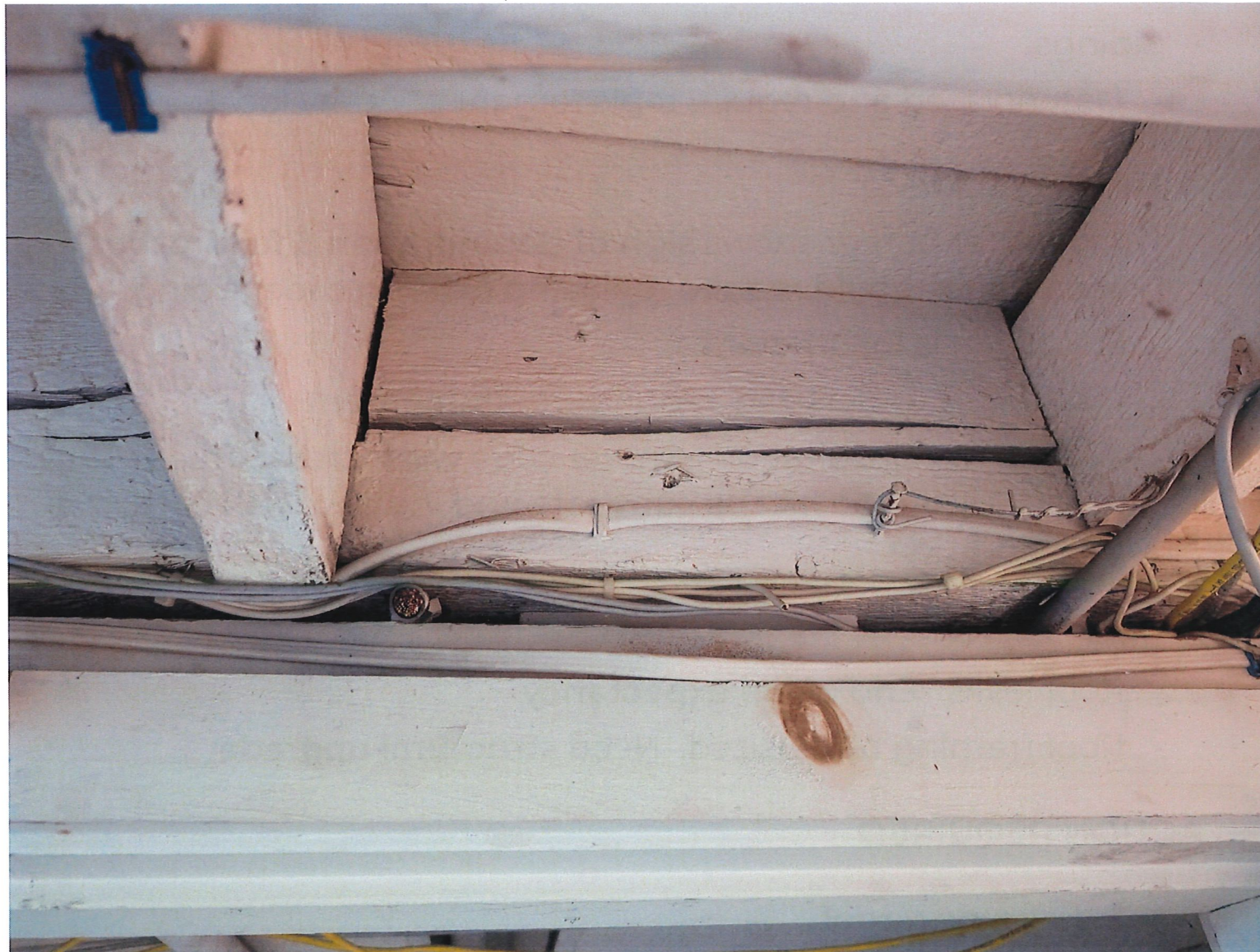
COMPROMISED FLOOR FRAMING BEAM
