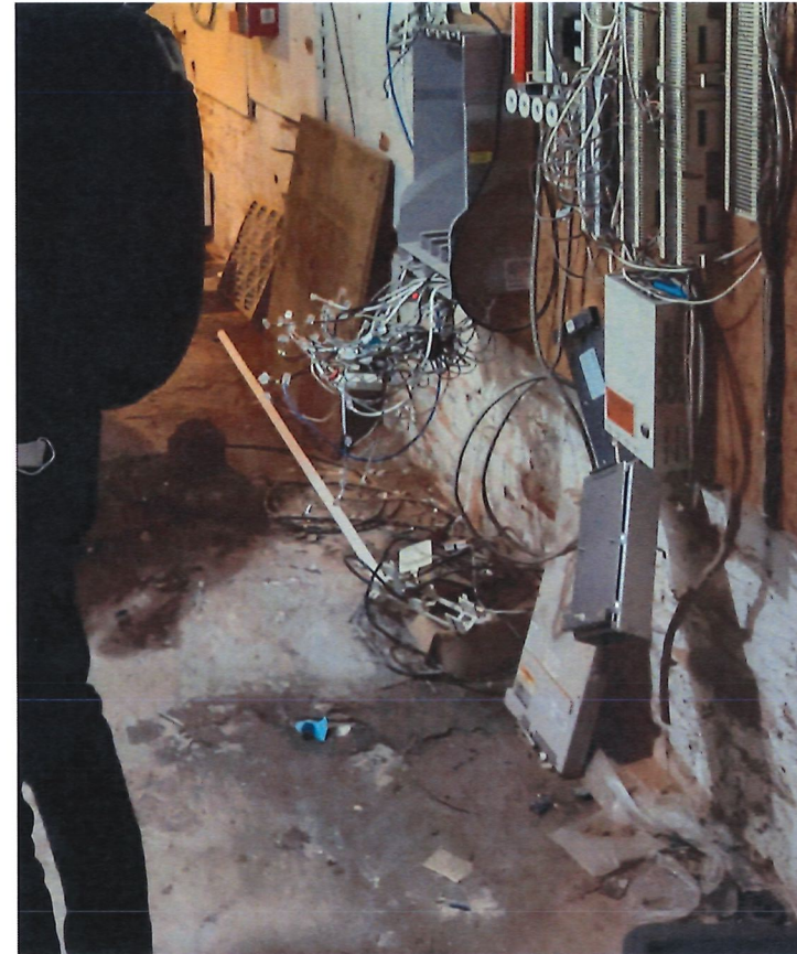
WATER INFILTRATION AT SLAB
