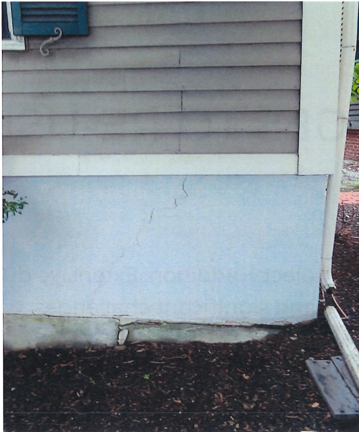
EXISTING FOUNDATION CRACKS/ BILLOWING
