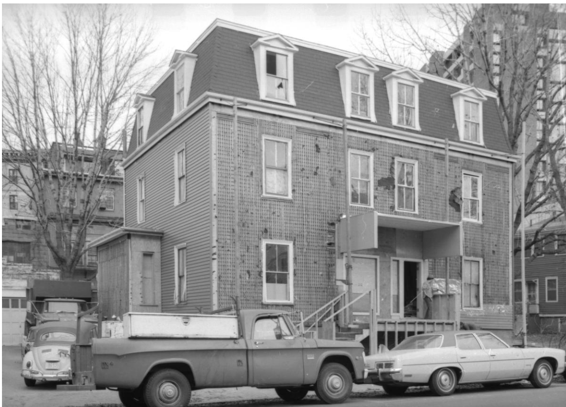
15 Mt. Auburn St., 1973. Asphalt siding and battens are being removed from the front façade; the left side has received new clapboards and trim. The residential double entries have been removed and a new canopy has been installed CHC staff photo
