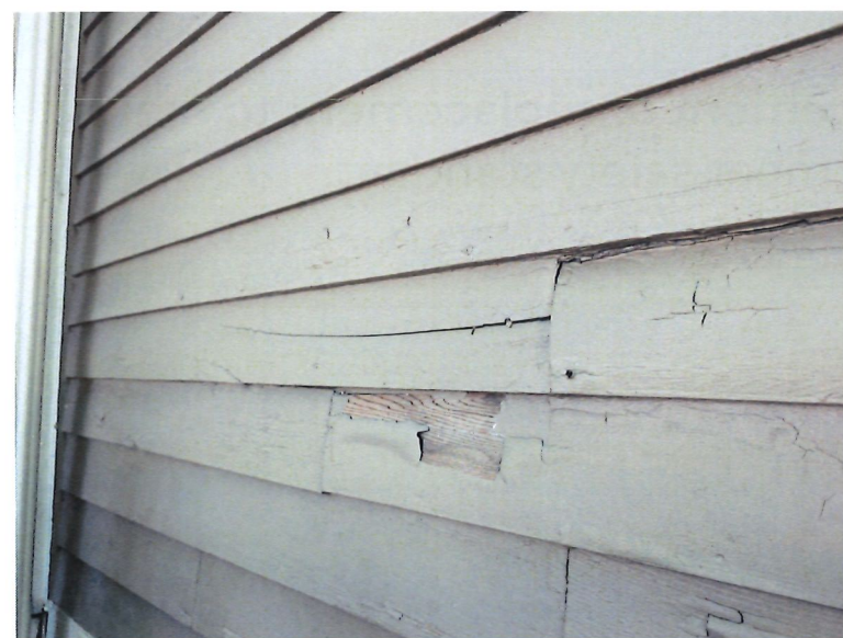
DETERIORATED SIDINGS, BUILDING PAPER, ROOF SHINGLES, AND CEILING
