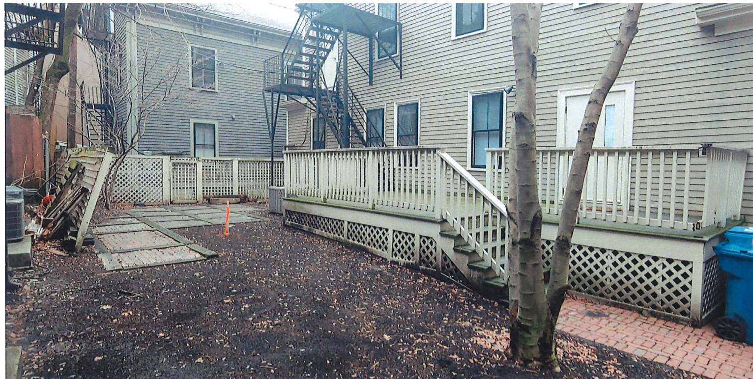
GARDEN ENTRANCE AND DECK
