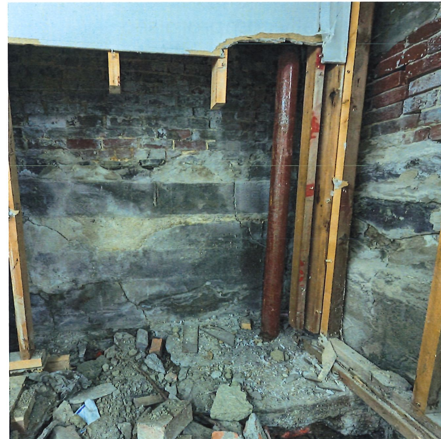
PREVIOUS UNDERPINNING/ REPAIR AT SE CORNER
