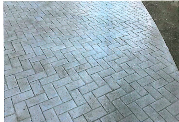
Colored, Stamped Concrete Paving
