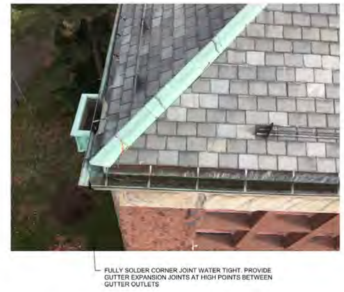
6 EXISTING HIP TERMINATION NTS
