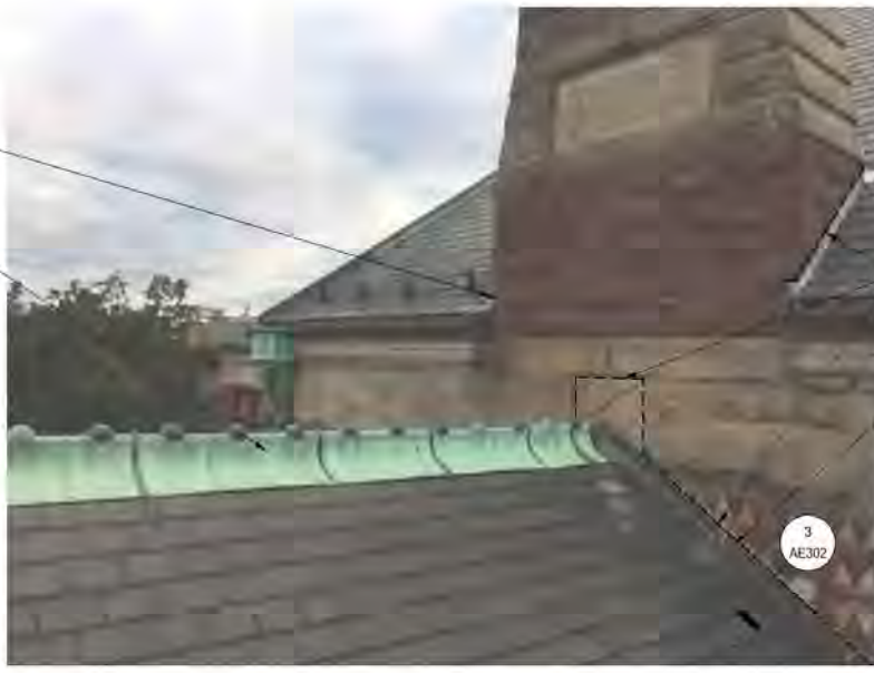
1 TYPICAL (E) RIDGE TERMINATION AT RISING WALL NTS
