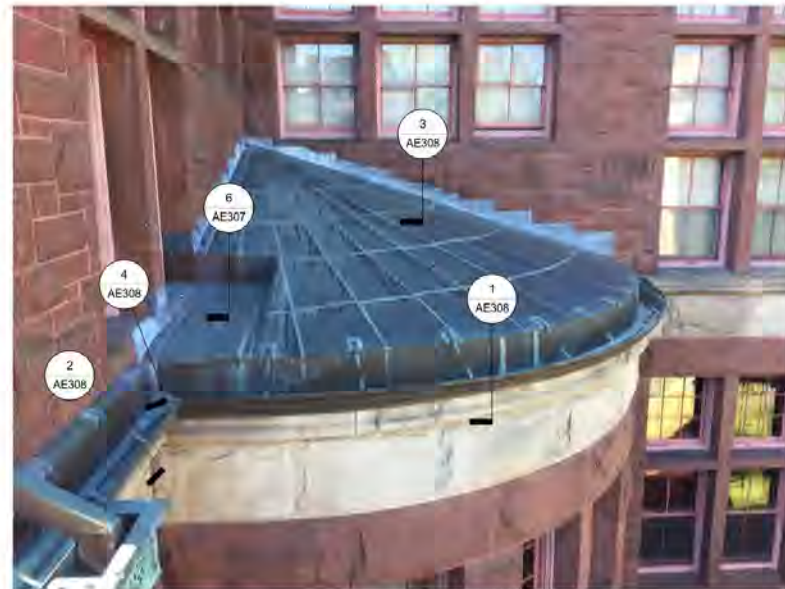
1 (E) COPPER PORTICO ROOF NTS
