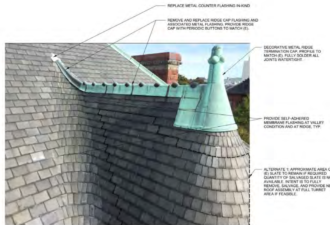
5 FRONT ENTRANCE DORMER CAP FLASHING NTS
